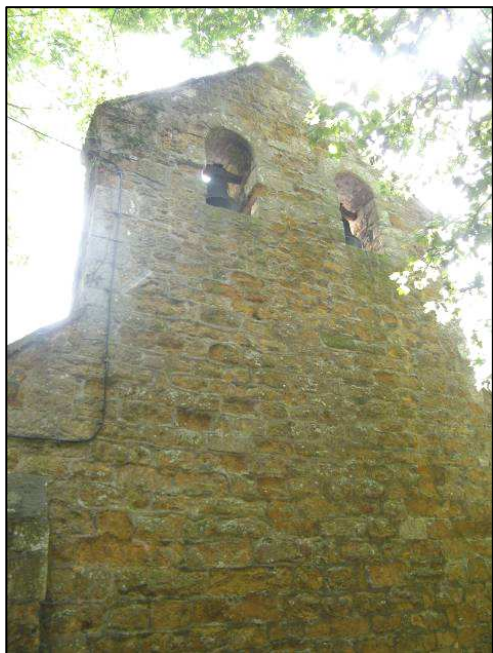
Plate 4 (shot 15): West elevation bell-cote
