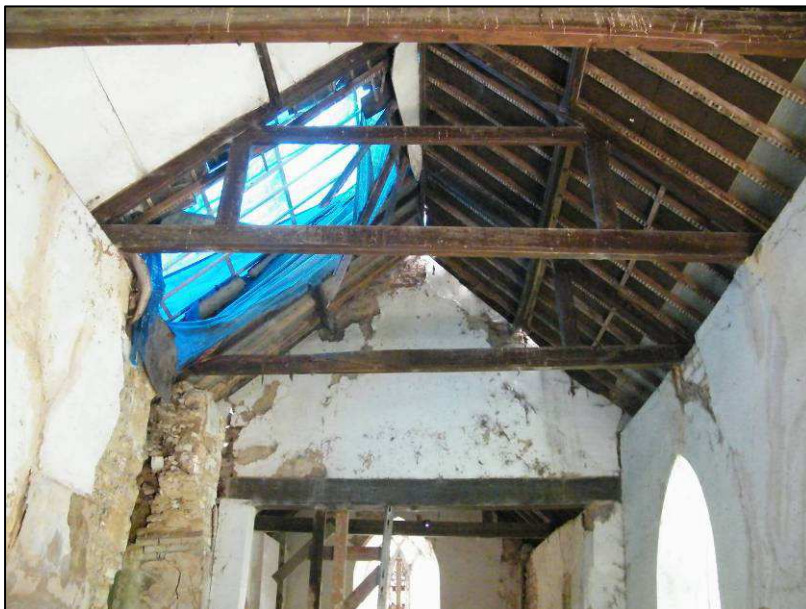
Plate 12 (shot 37): Queen post roof structure, looking east
