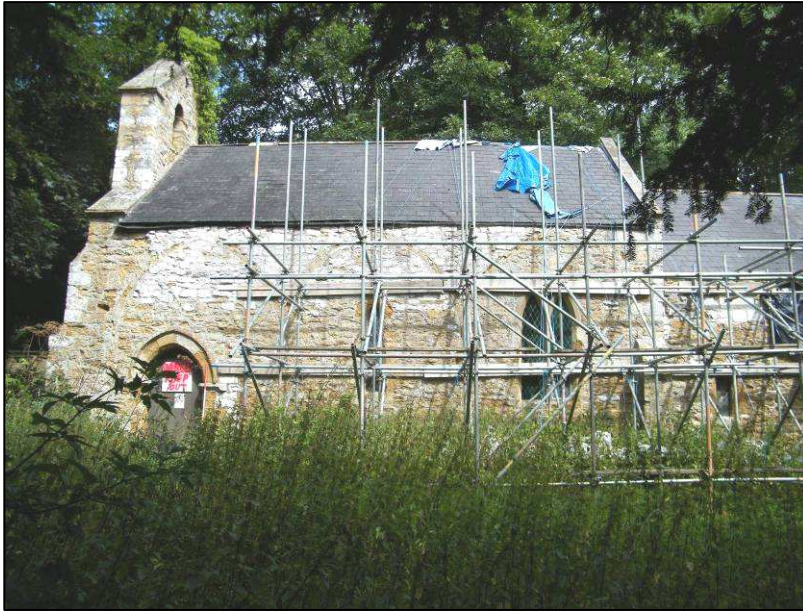
Plate 1 (shot 6): South elevation of the nave
