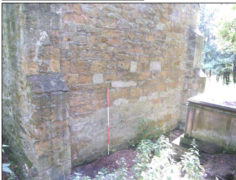
Plate 5 (shot 14): West elevation buttresses, 2m scale
