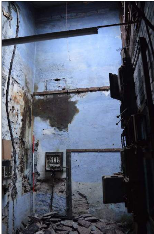
Plate 61 (shot 361): Bearing box on south wall. Looking southeast, 2m scale
