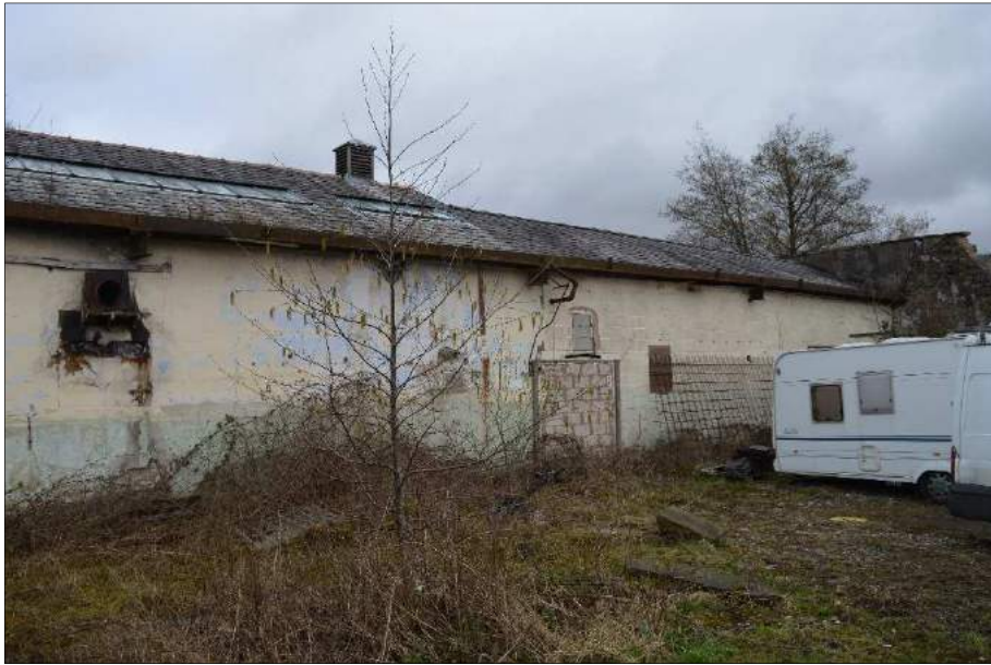
Plate 48 (shot 135): South elevation. Looking north, 1m scale
