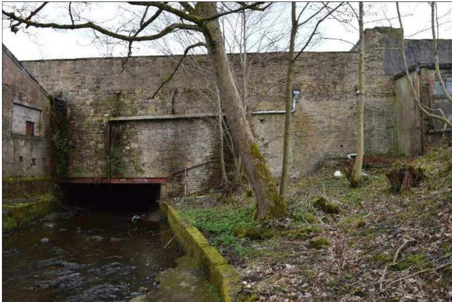
Plate 75 (shot 192): West elevation and culvert. Looking northeast, 2m scale
