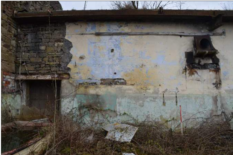
Plate 49 (shot 136): Close up of the south elevation showing former access to the spinning mill as well as an old bearing box. Looking northwest, 1m scale
