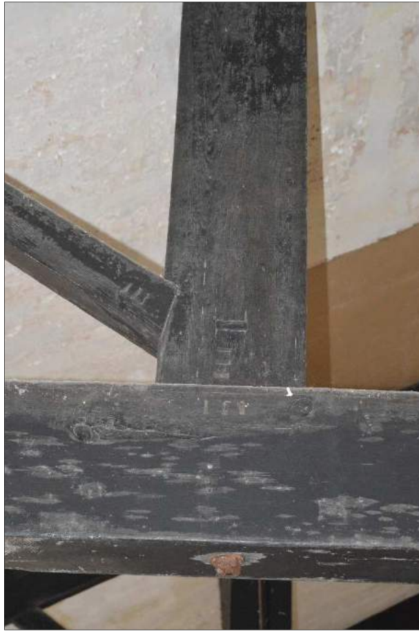
Plate 43 (shot 70): Close up of carpenter's assembly marks.
