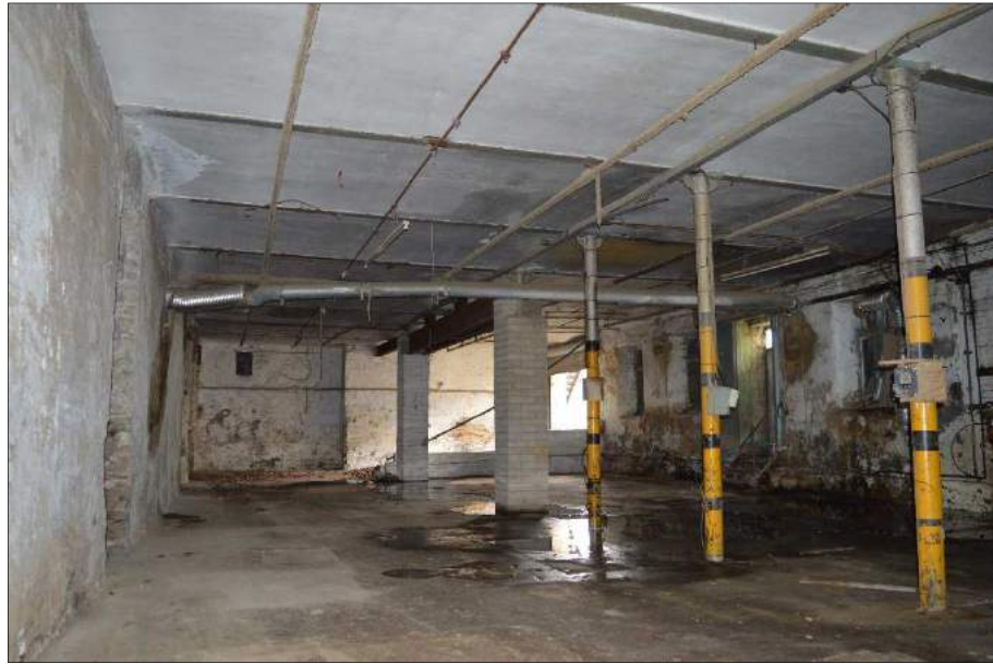
Plate 12 (shot 311): Ground floor, northern half of building A. Looking
