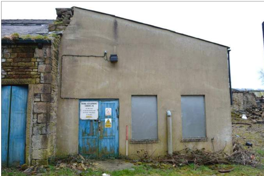
Plate 63 (shot 43): Lean-to extension, northwest elevation. Looking southeast, 1m scale
