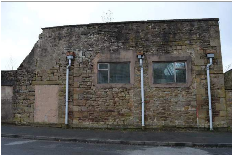
Plate 47 (shot 125): West elevation of engine house with remains of the early 1894 spinning mill left of the quoins. Looking southwest, 1m scale
