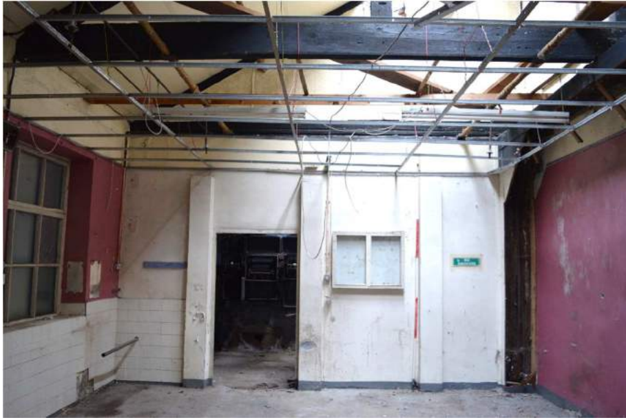
Plate 60 (shot 359): Later partition wall. Looking northeast, 2m scale
