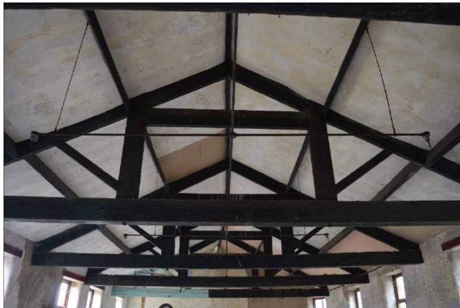
Plate 42 (shot 67): Roof structure. Looking west
