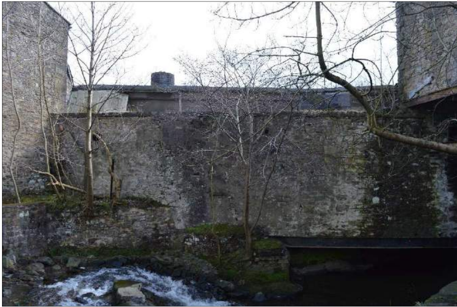
Plate 74 (shot 408): North elevation with culvert. Looking south
