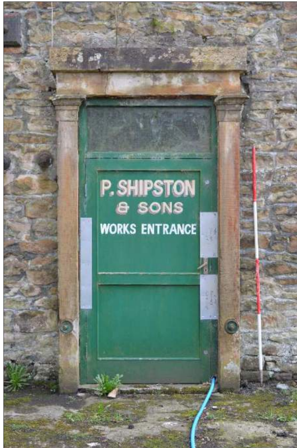
Plate 2 (shot 386): Main entrance of building A. Looking southeast, 2m scale
