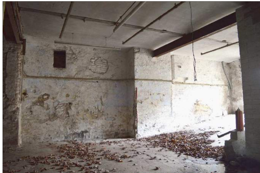
Plate 13 (shot 312): Bearing boxes in the workshop's west partition. Looking west, 2m scale
