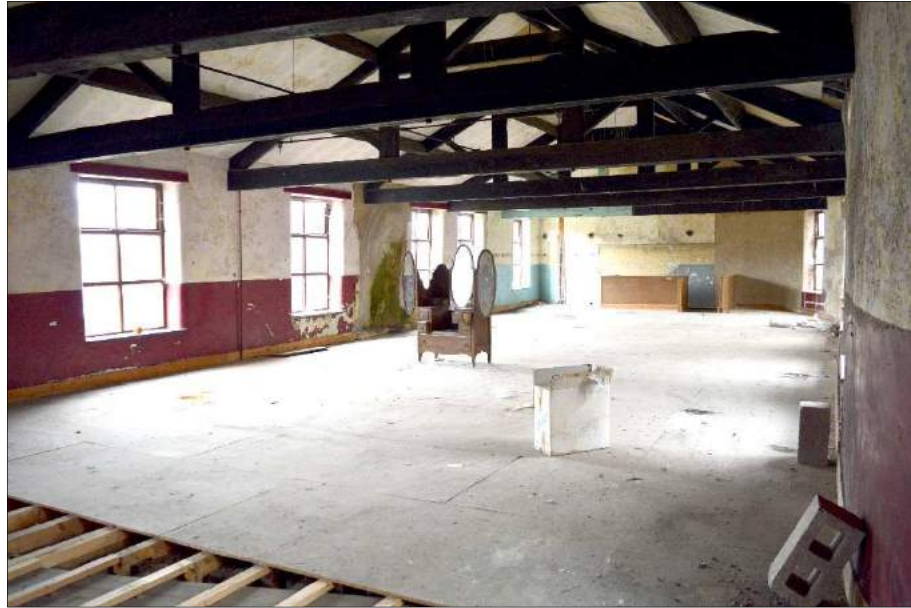
Plate 41 (shot 87): First floor. Looking southwest, 1m scale
