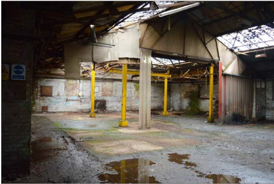
Plate 72 (shot 228): General view towards the south. Looking south, 2m scale
