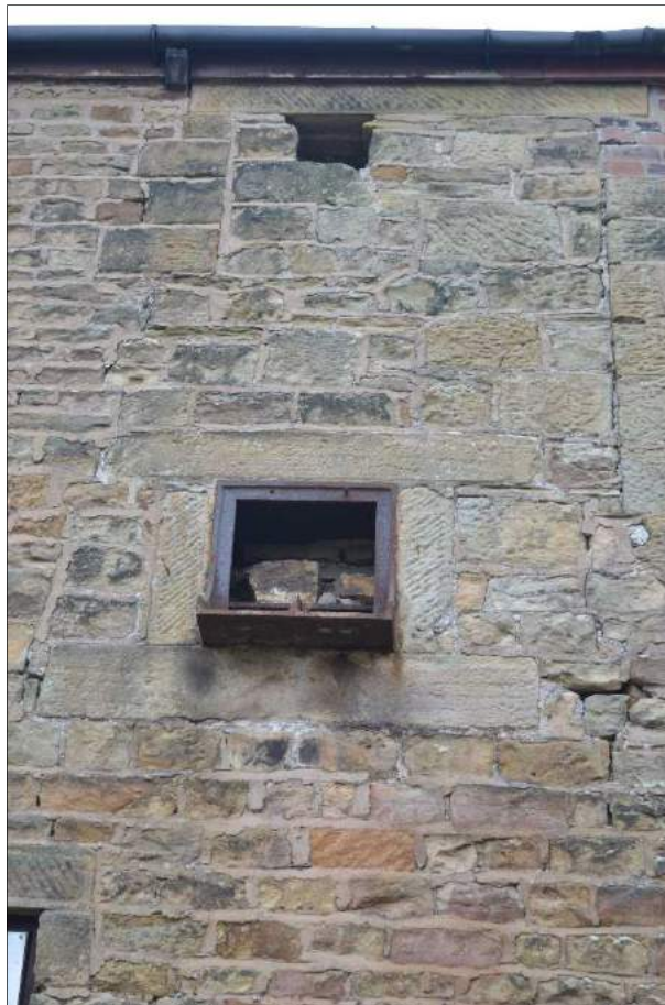
Plate 32 (shot 16): Later bearing box within blocked window. Looking north
