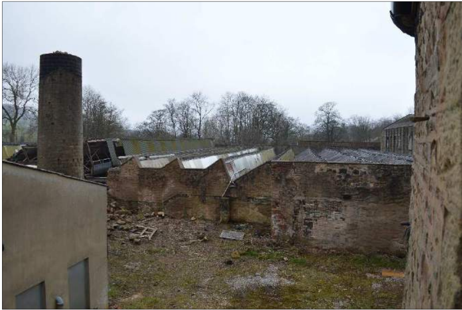
Plate 76 (shot 57): Overlooking northeast elevation and roof of building E. Looking west-southwest
