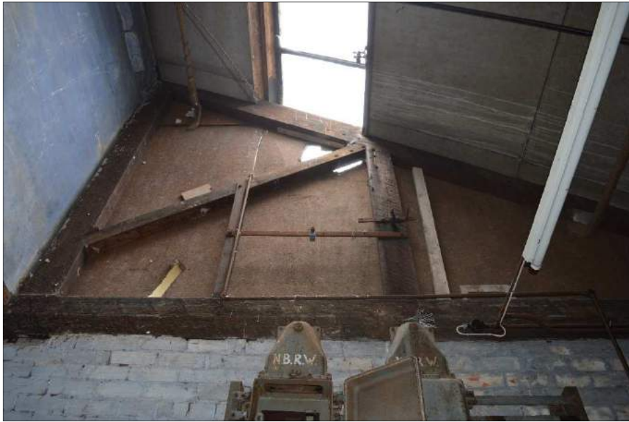
Plate 62 (shot 366): Roof truss. Looking southwest
