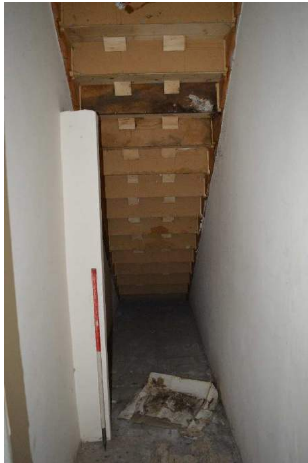
Plate 40 (shot 98): Later staircase to first floor. Looking south, 1m scale
