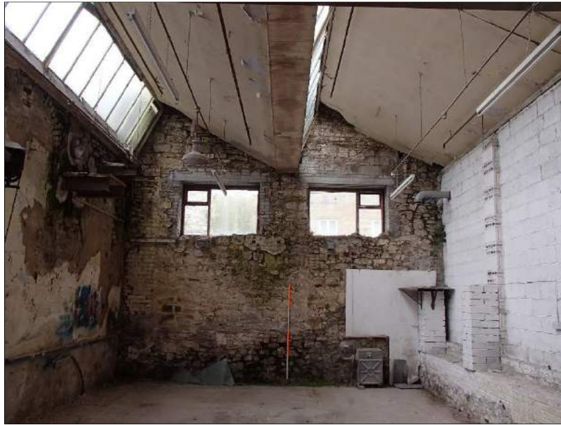
Plate 50 (shot 415): Building C engine house interior, looking northeast, 2m scale
