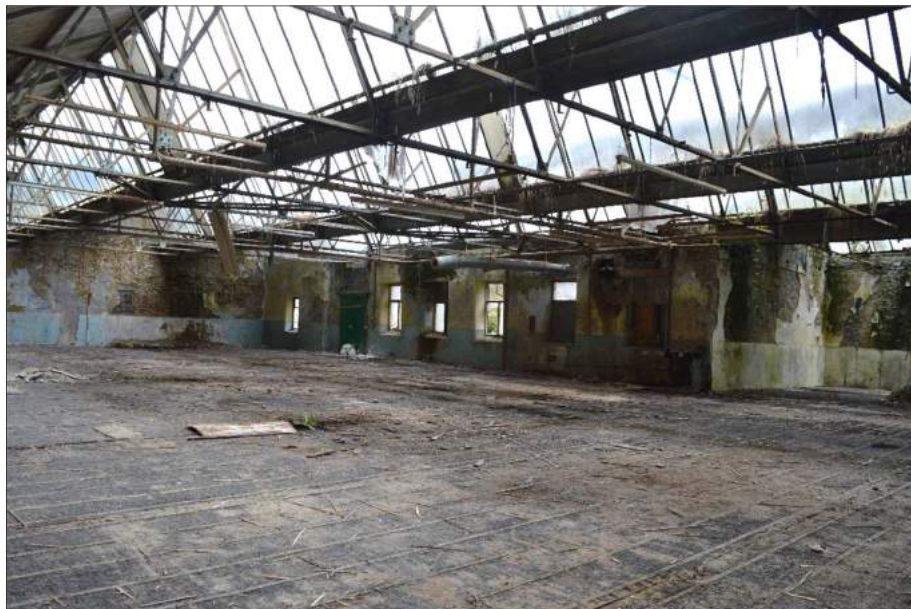
Plate 23 (shot 239): First floor of the spinning mill. Looking northwest, 2m scale
