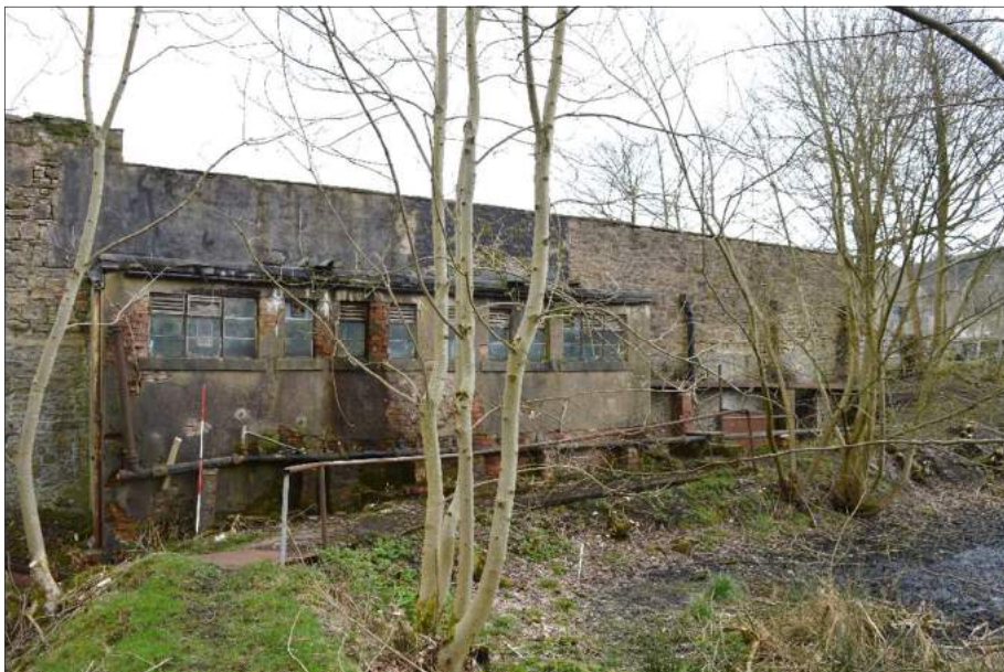
Plate 87 (shot 191): Lavatories from 1947 on the west elevation. Looking east, 2m scale
