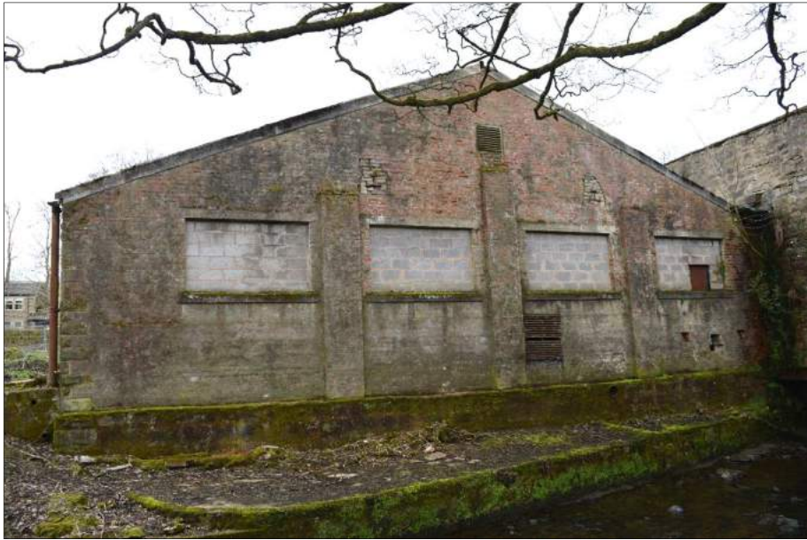
Plate 70 (shot 193): South elevation. Looking northeast
