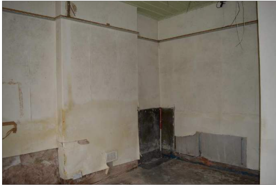
Plate 37 (shot 120): Former office and blocked up fireplace. Looking southeast, 1m scale
