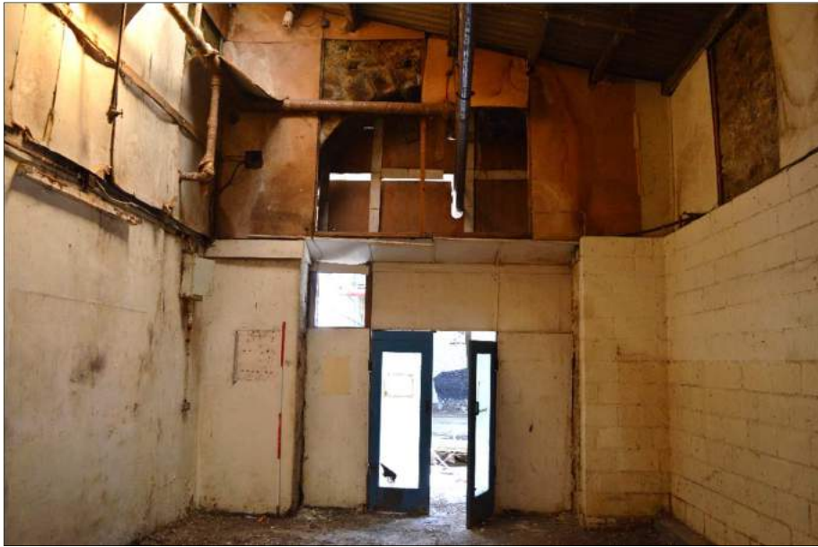
Plate 66 (shot 343): Interior view of later partition. Looking southeast, 2m scale
