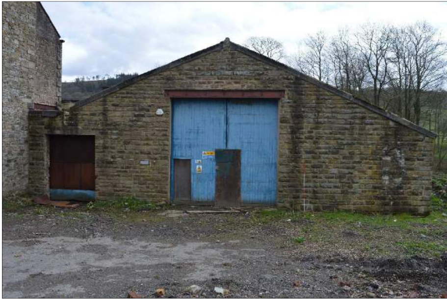
Plate 68 (shot 371): North elevation of D. Looking south, 2m scale
