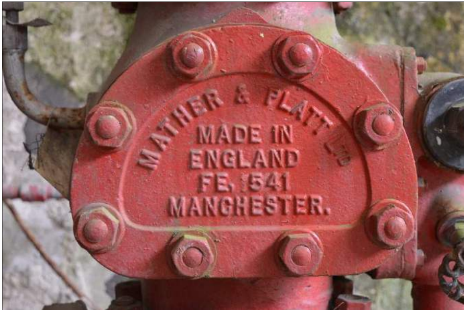
Plate 93 (shot 183): Maker's mark Mather & Platt Ltd, Manchester. Looking southwest
