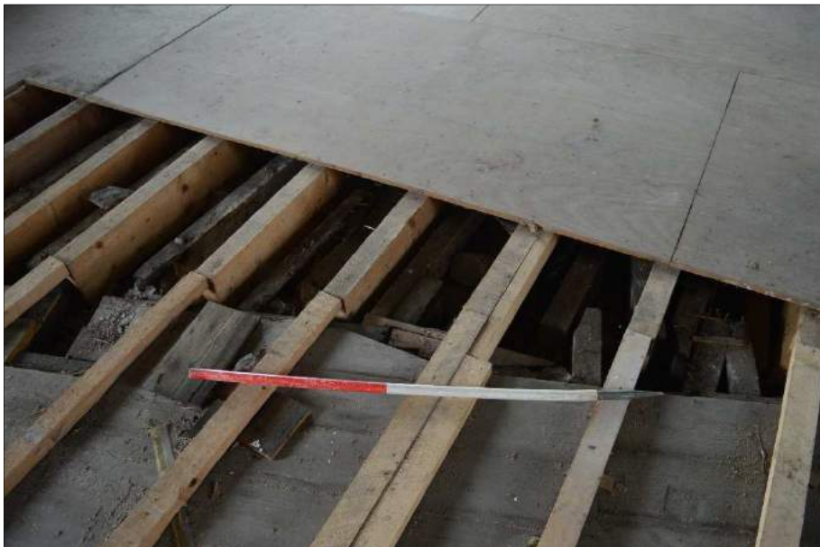
Plate 44 (shot 61): Original floor boards under later joists. Looking east, 1m scale
