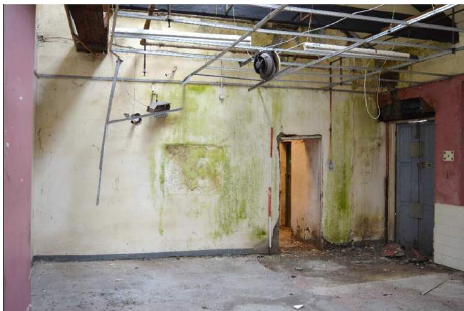
Plate 59 (shot 352): West partition wall. Looking northwest, 2m scale
