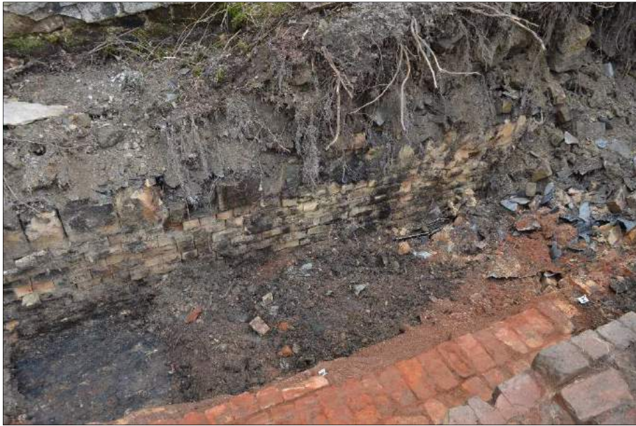
Plate 99: East wall showing facing firebricks 209 and cut stone 208. Looking east-southeast
