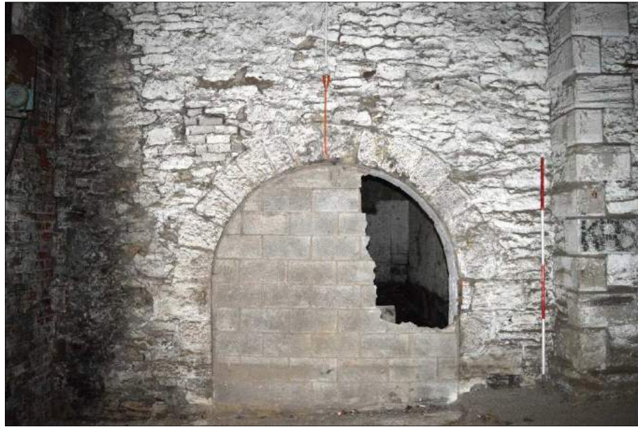
Plate 16 (shot 284): Original north elevation and blocked rounded arched opening. Looking northwest, 2m scale
