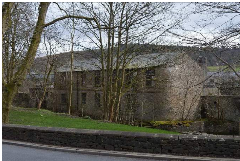
Plate 28 (shot 412): North elevation of Building B, looking southeast
