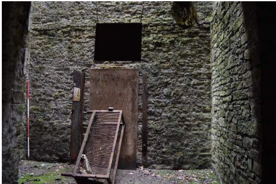
Plate 19 (shot 338): Ventilation shaft seen from 'store room. Small sign near boarded up door says highly flammable. Looking west-southwest, 2m scale
