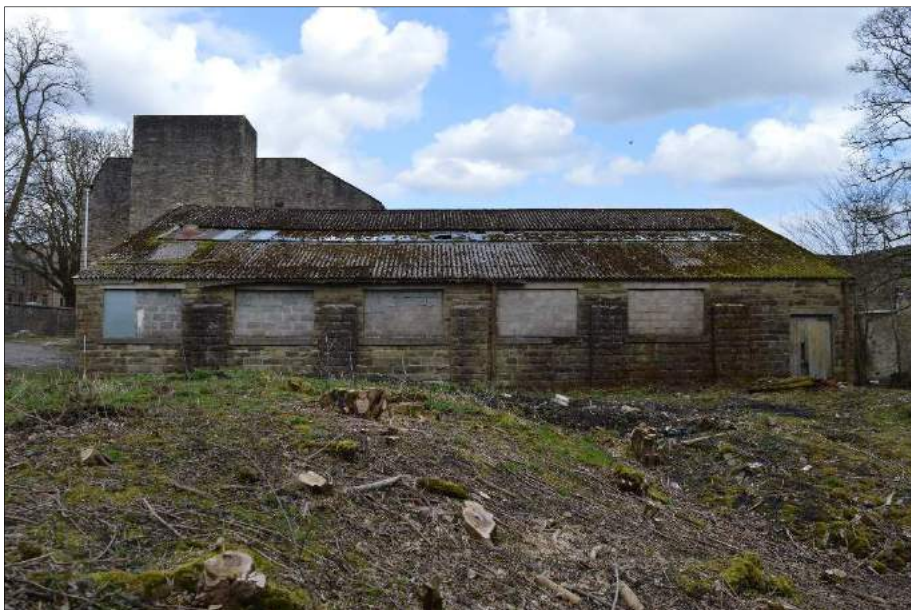
Plate 69 (shot 370): West elevation. Looking east-northeast, 2m scale
