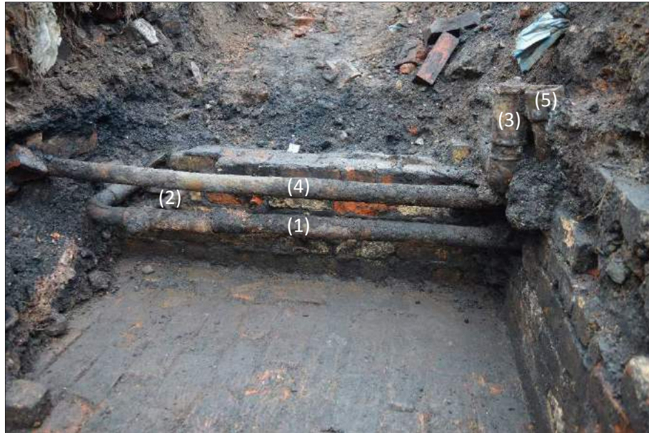
Plate 98: Brick wall 109, surrounded by pipework 110. Looking northwest
