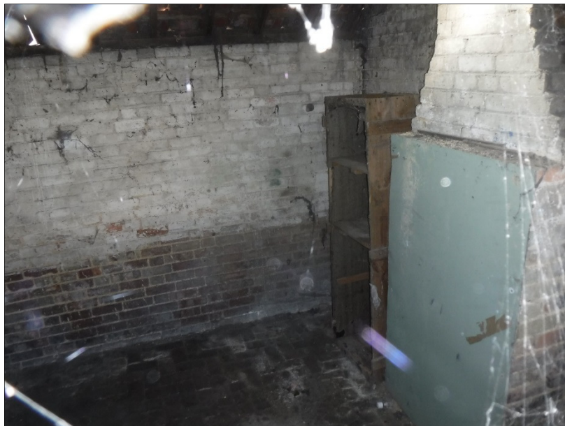
Plate 28 (shot 17): General view of the southernmost room. Looking south
