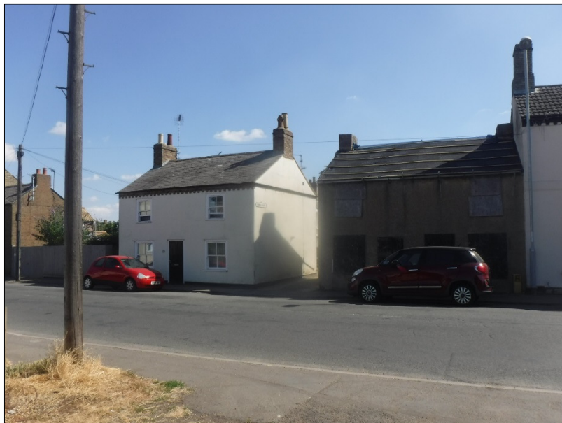
Plate 1 (shot 40): General view of 113 and 115 to the right of shot, also showing 117 to the left. Looking northeast, 1m scale
