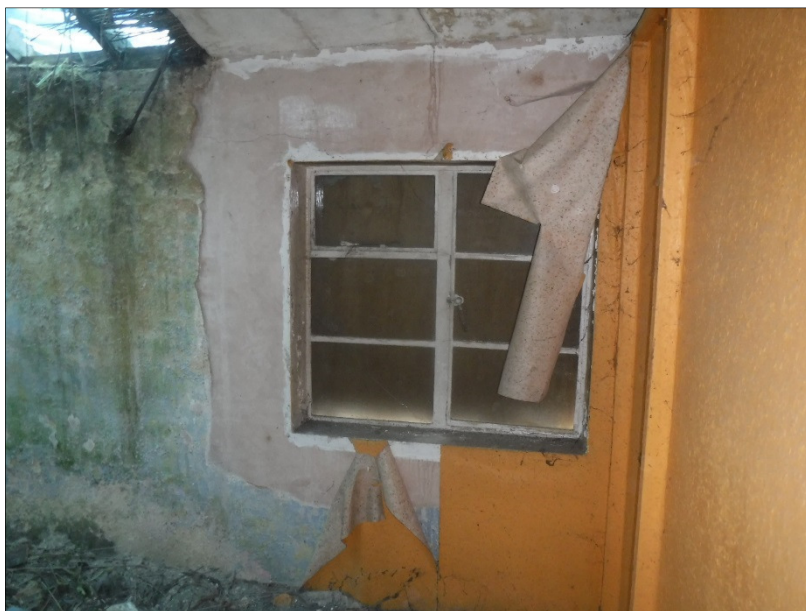
Plate 15 (shot 69): Rear bedroom and window. Looking northeast
