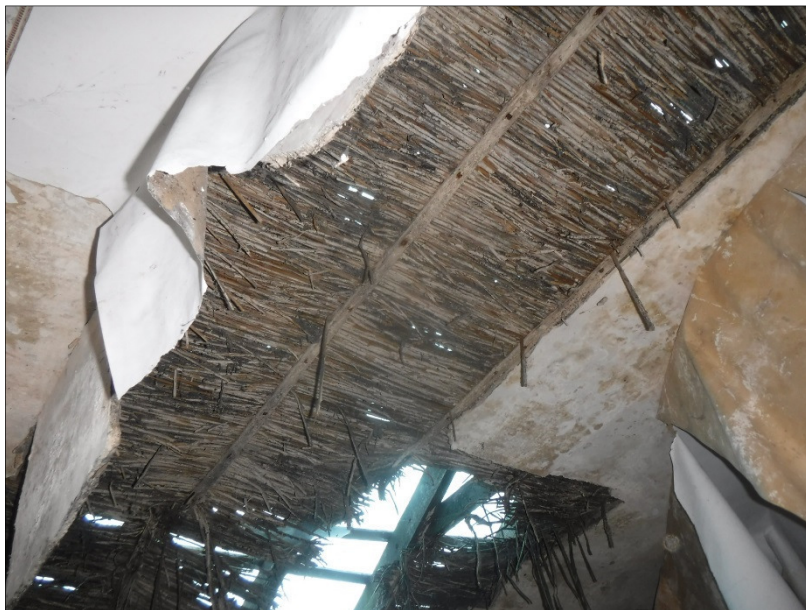
Plate 11 (shot 63): Reed filling above the laths in 113. Looking southeast
