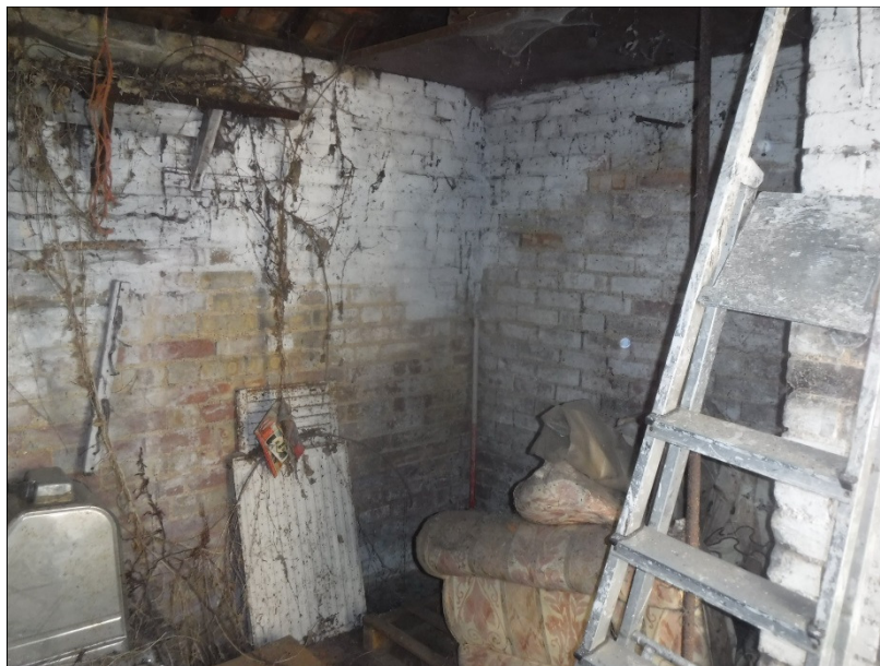
Plate 26 (shot 13): General view of the washhouse. Looking south, 1m scale
