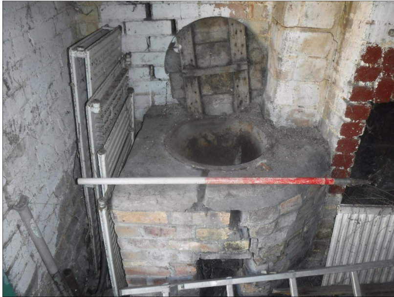
Plate 25 (shot 15): Copper with wooden lid near the fireplace. Looking northeast, 1m scale
