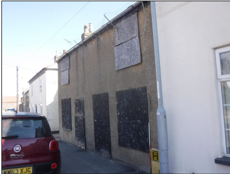
Plate 2 (shot 43): Southwest elevation. Looking northeast, 1m scale
