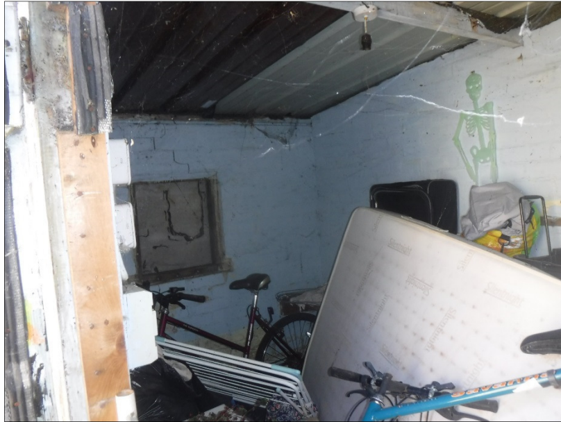
Plate 37 (shot 24): General view of brick lean-to store. Looking east
