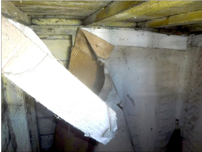
Plate 33 (shot 32): General internal view towards southwest end of shed. Looking south
