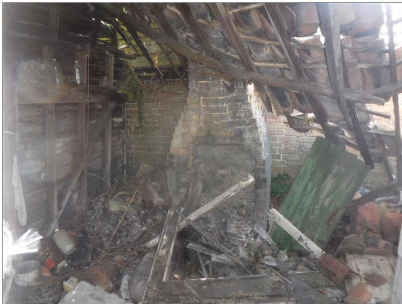
Plate 34 (shot 33): Fireplace within southwest shed, northeast part. Looking southeast
