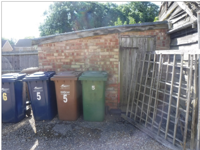
Plate 36 (shot 22): Brick lean-to. Looking southeast, 1m scale
