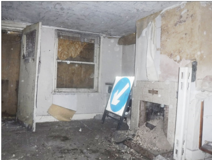
Plate 13 (shot 66): Living room of No 115. Looking northwest
