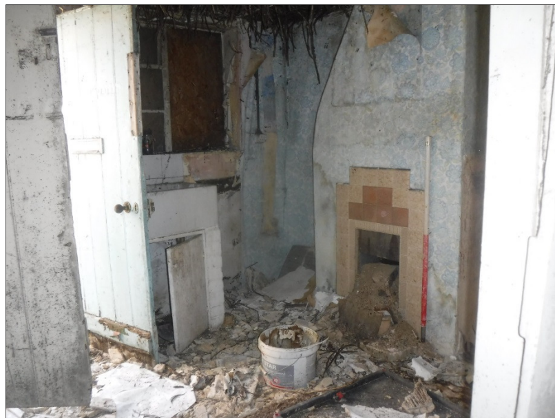
Plate 7 (shot 51): General view of the kitchen in 113. Looking southeast, 1m scale
