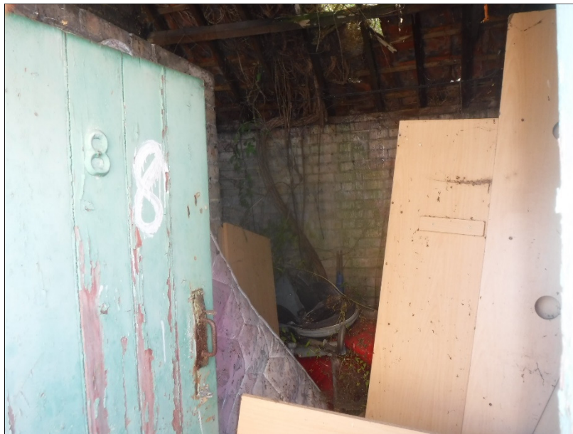
Plate 22 (shot 10): General view of the L-shaped store. Looking southeast
