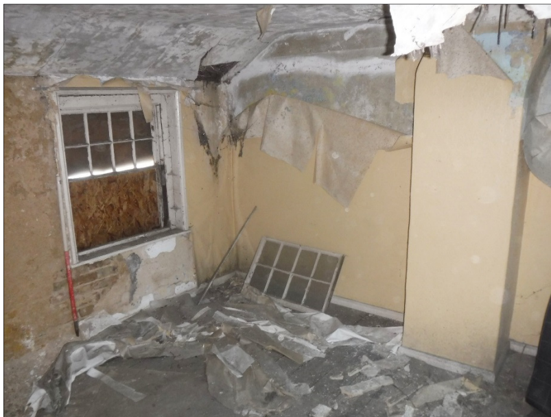
Plate 17 (shot 71): Bedroom fronting High Street. Looking northwest, 1m scale
