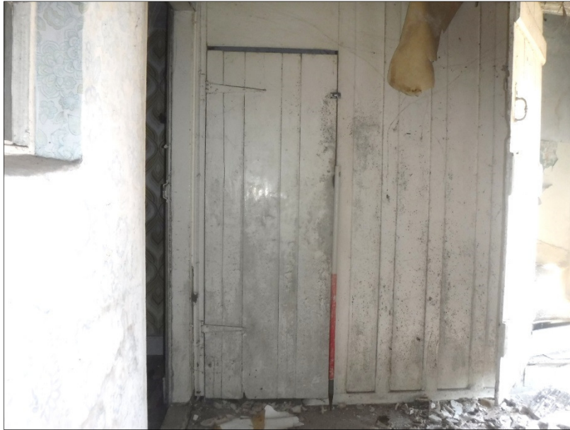
Plate 8 (shot 53): Panelling and under stairs cupboard in 113. Looking northwest, 1m scale
