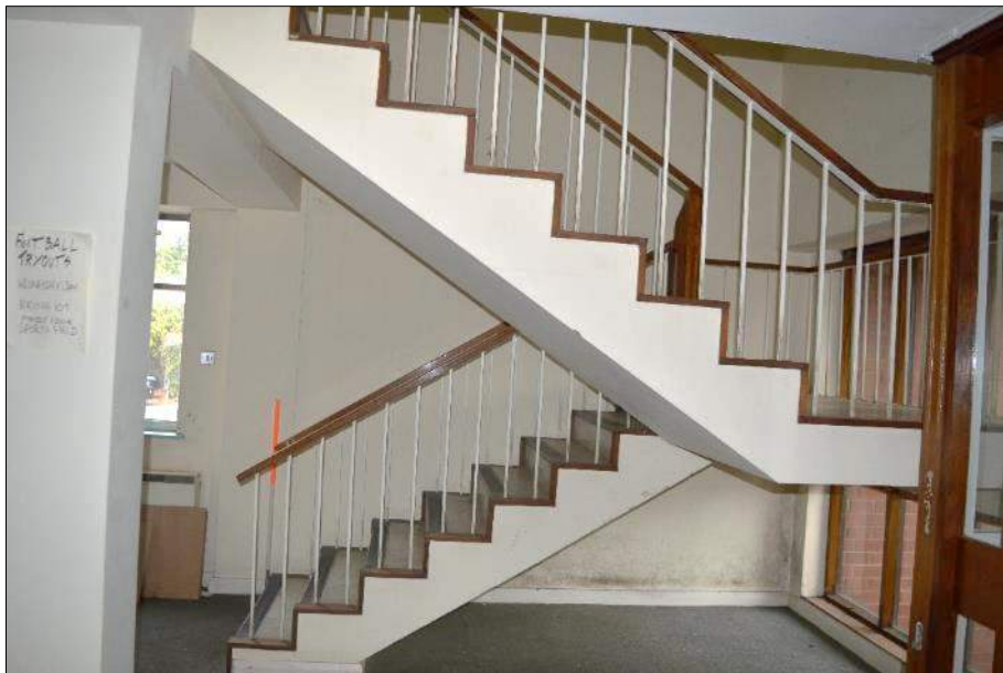
Plate 40 (shot 117): Staircase within entrance area looking south, scale 1m
