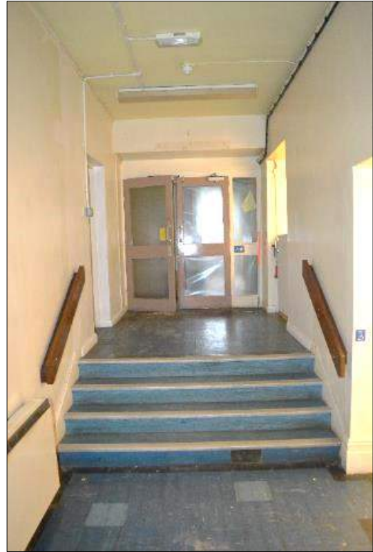
Plate 36 (shot 82): Entrance hall steps in east wing looking east, scale 1m
