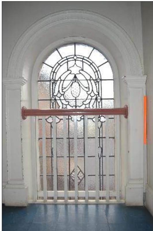
Plate 42 (shot 199): Leaded window in north elevation, looking north, scale 1m
