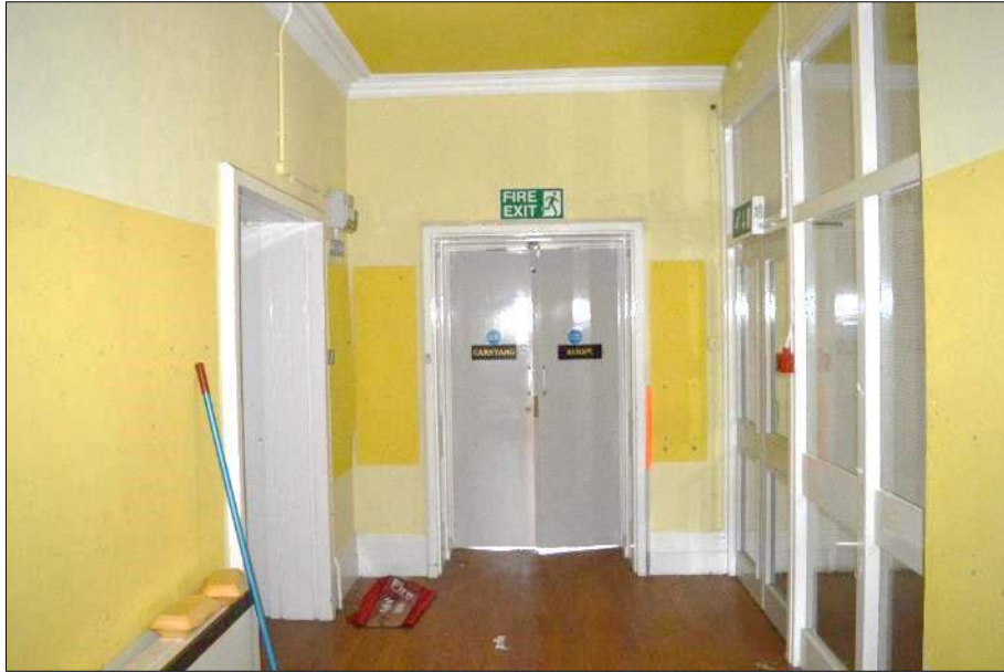
Plate 43 (shot 173): West facing view of corridor looking towards Room 101, scale 1m
