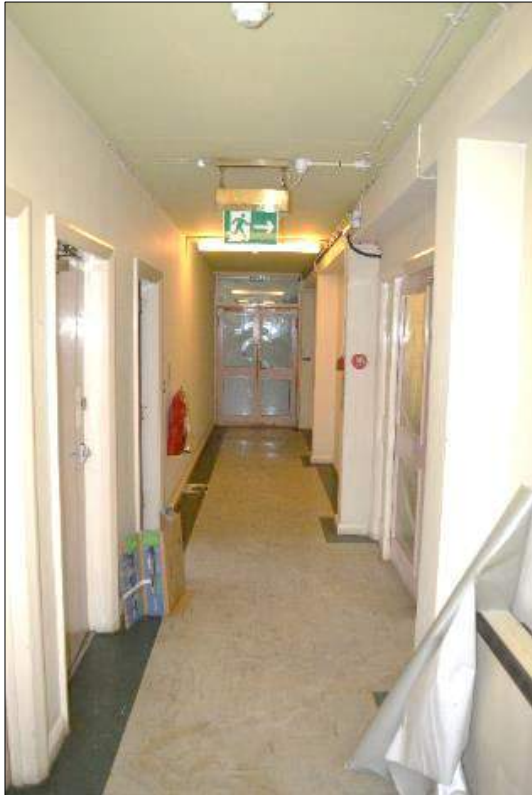
Plate 37 (shot 87): Ground floor corridor in 1960's extension looking south, scale 1m
