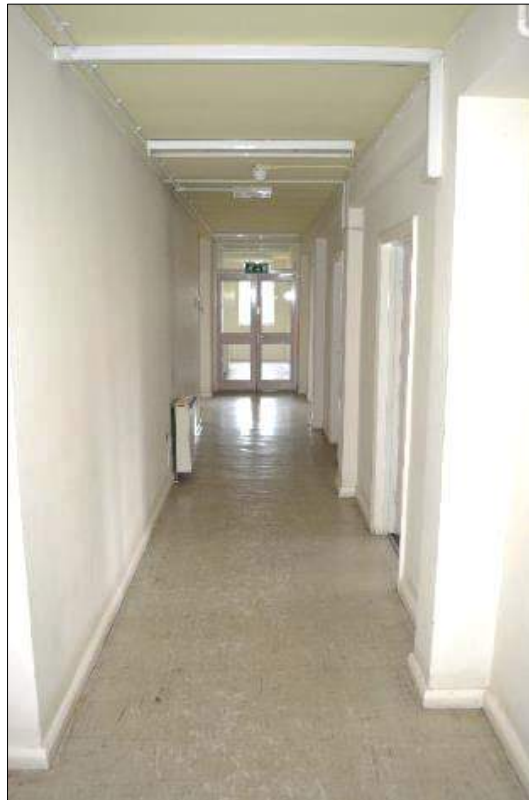
Plate 51 (shot 128): First floor corridor in 1960's extension looking south, scale 1m
