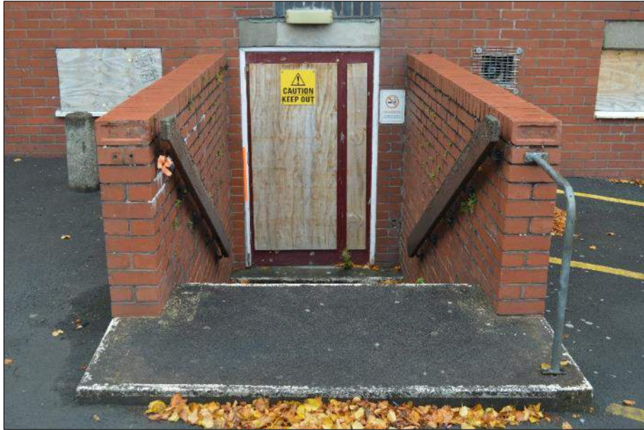
Plate 22 (shot 32): Side entrance of 1960's extension looking north, scale 1m
