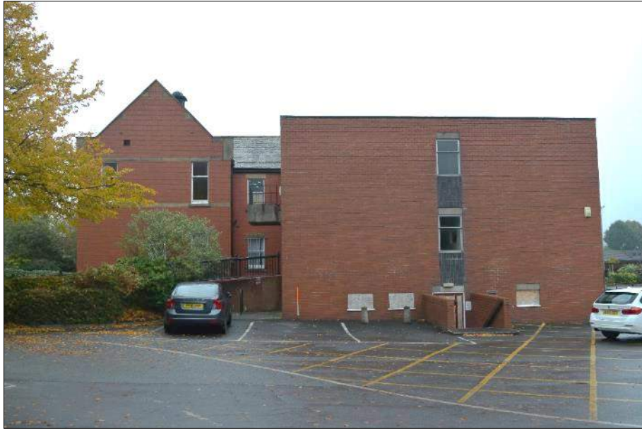
Plate 20 (shot 28): South elevation looking north, scale 1m
