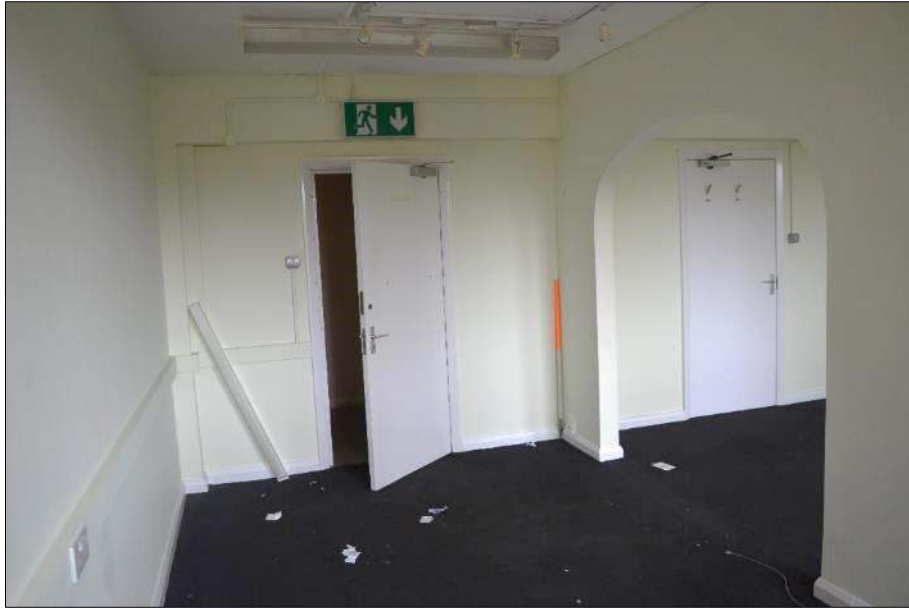
Plate 52 (shot 140): View of Room 117, showing arched opening looking east, scale 1m
