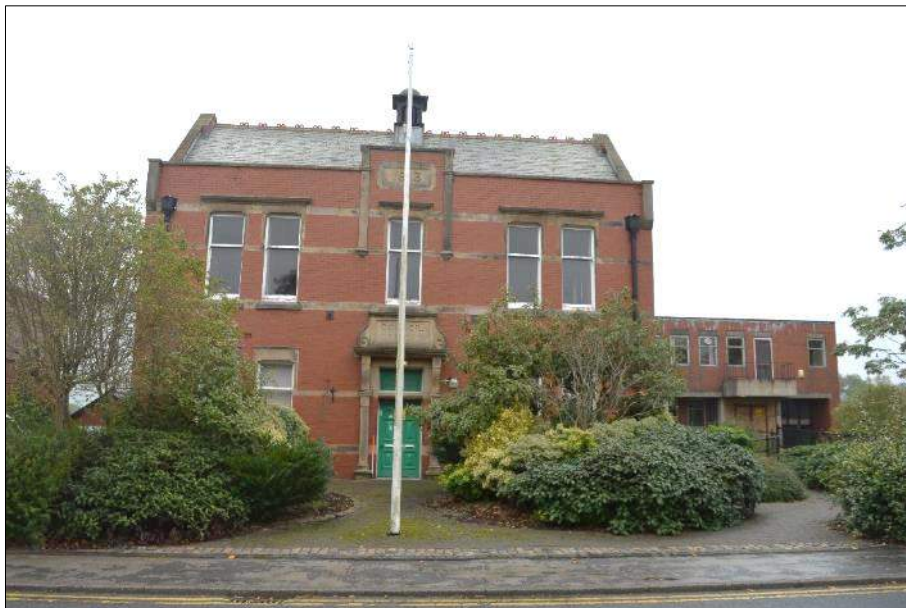
Plate 2 (shot 3): West elevation looking east, scale 1m
