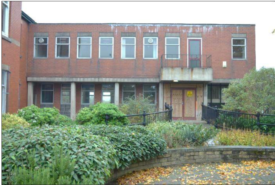
Plate 13 (shot 16): West elevation of 1960's extension looking east, 1m scale
