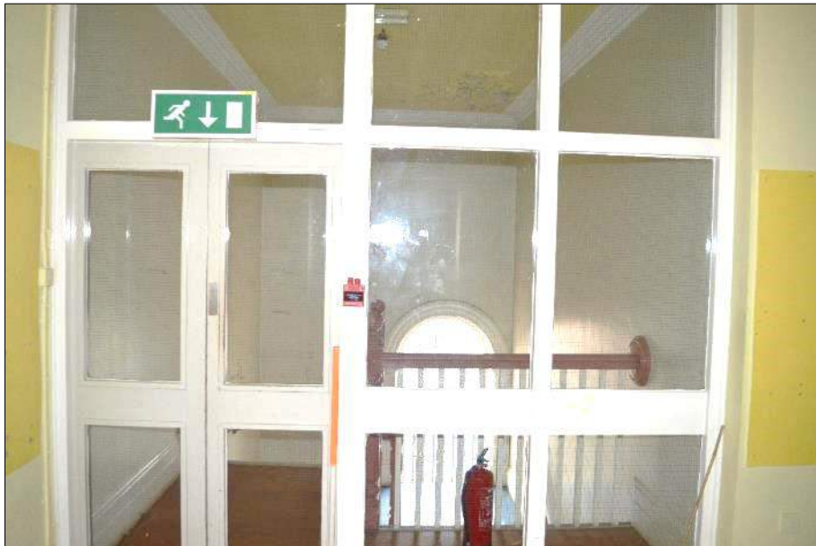
Plate 44 (shot 174): North facing view from corridor looking towards stairwell, scale 1m
