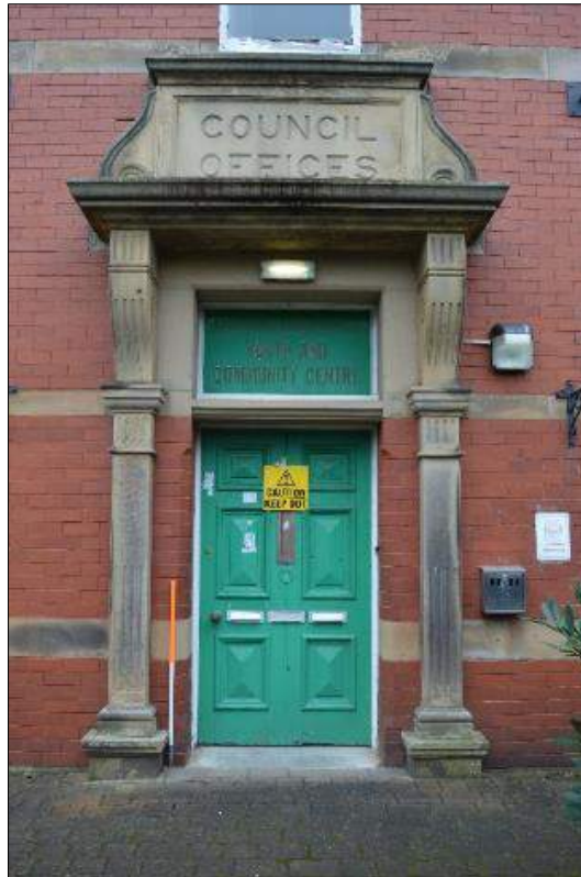
Plate 3 (shot 7): Main entrance looking east, 1m scale
