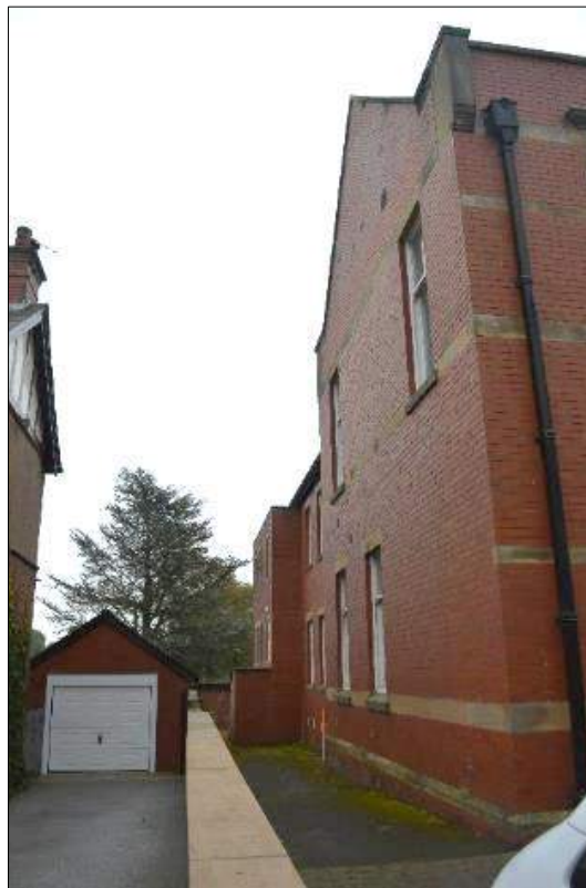
Plate 9 (shot 57): Oblique view of north elevation looking east, scale 1m
