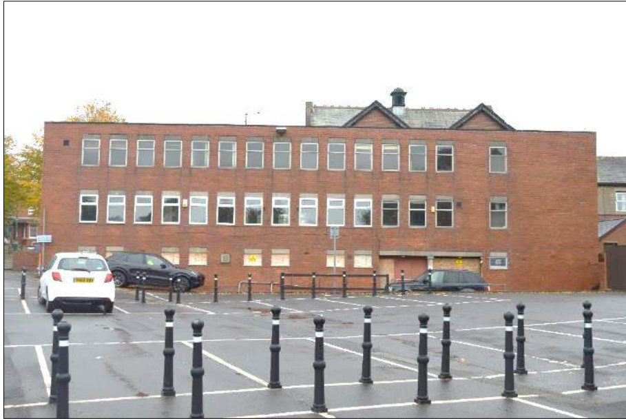
Plate 24 (shot 40): East elevation looking west, scale 1m
