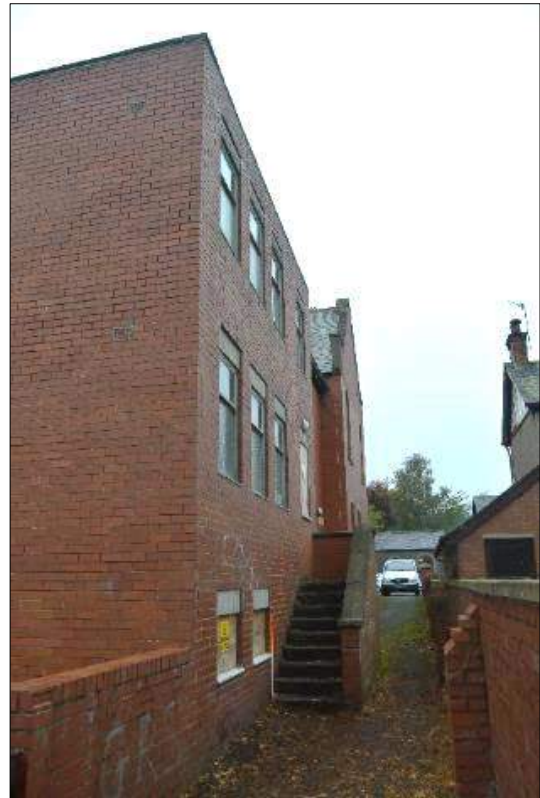
Plate 27 (shot 47): Oblique view of 1960's extension's north elevation looking west, scale 1m
