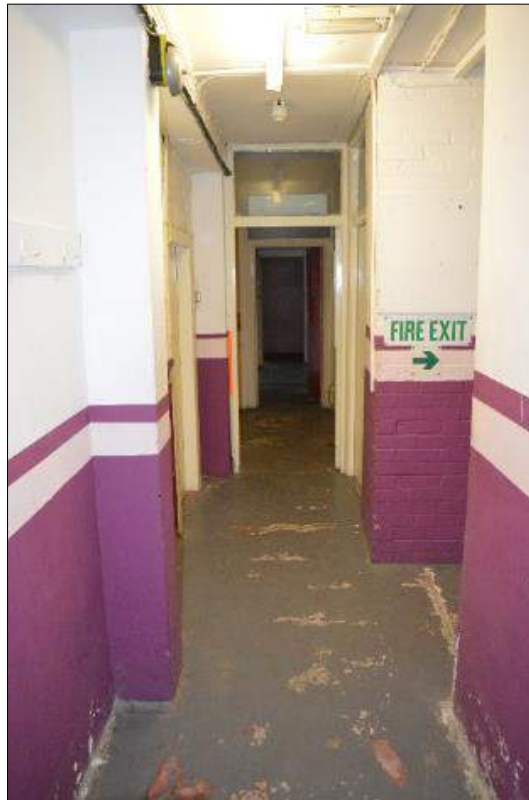
Plate 55 (shot 241): Basement corridor looking north, scale 1m
