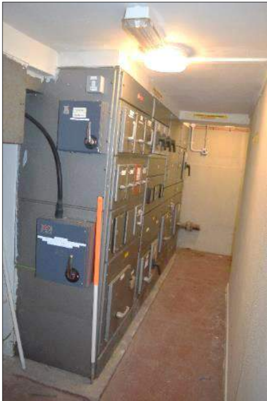
Plate 46 (shot 224): Meter room looking north, scale 1m
