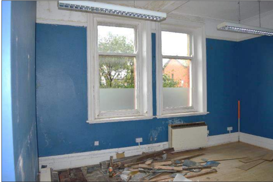
Plate 31 (shot 61): General view of room G17 looking northeast, scale 1m
