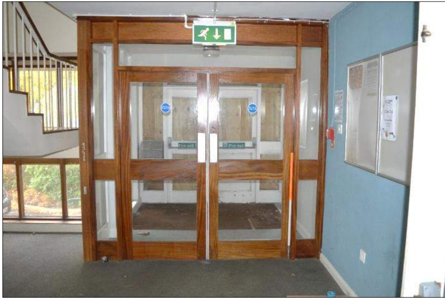
Plate 39 (shot 111): 1960's extension entrance area looking west, scale 1m
