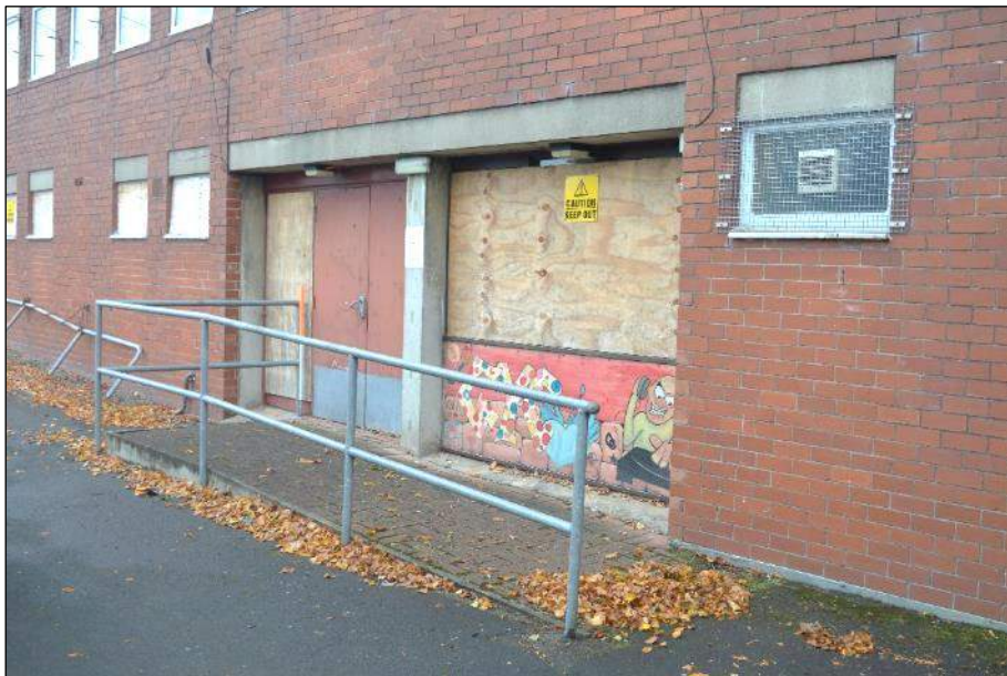
Plate 25 (shot 42): Rear entrance to 1960's extension, looking southwest, scale 1m
