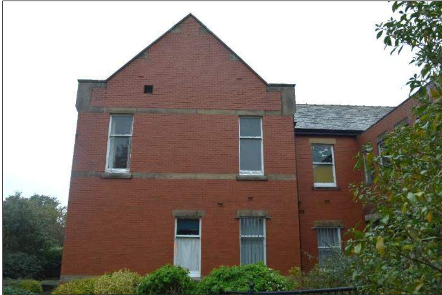
Plate 8 (shot 13): South elevation of original building looking north, scale 1m
