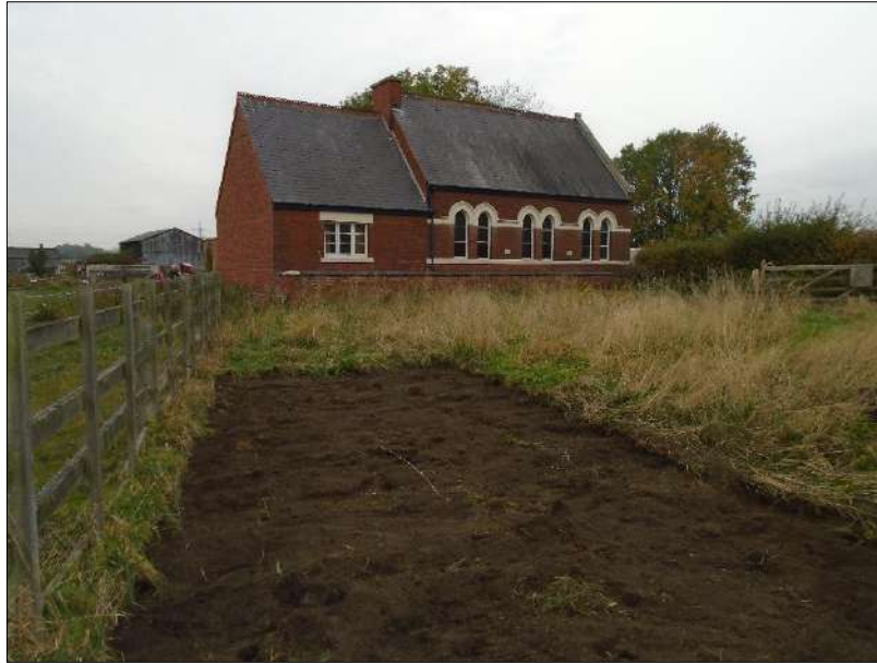
Plate 2: Area to the northeast stripped of turf. Looking southwest
