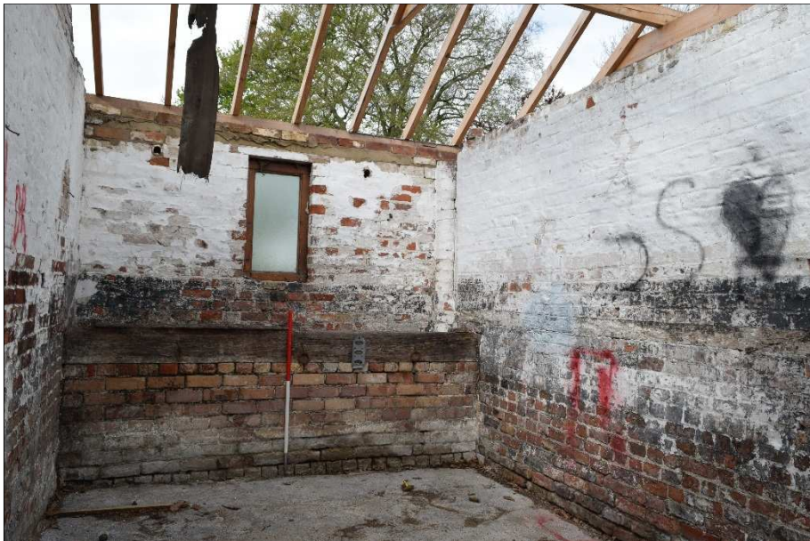
Plate 20 (shot 40): General view of southern stable box. Looking northeast, 1m scale
