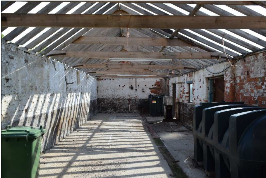
Plate 30 (shot 23): General internal view of Building B. Looking east, 1m scale
