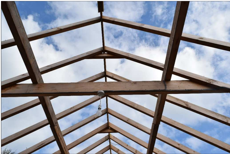
Plate 22 (shot 41): Roof structure above the centre bays. Looking north
