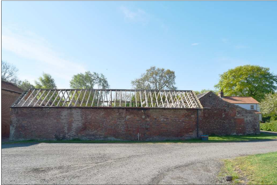
Plate 26 (shot 3): North elevation of Building B. looking south, 1m scale
