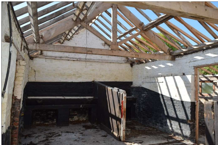
Plate 12 (shot 31): View of south stalls. Looking southwest, 1m scale
