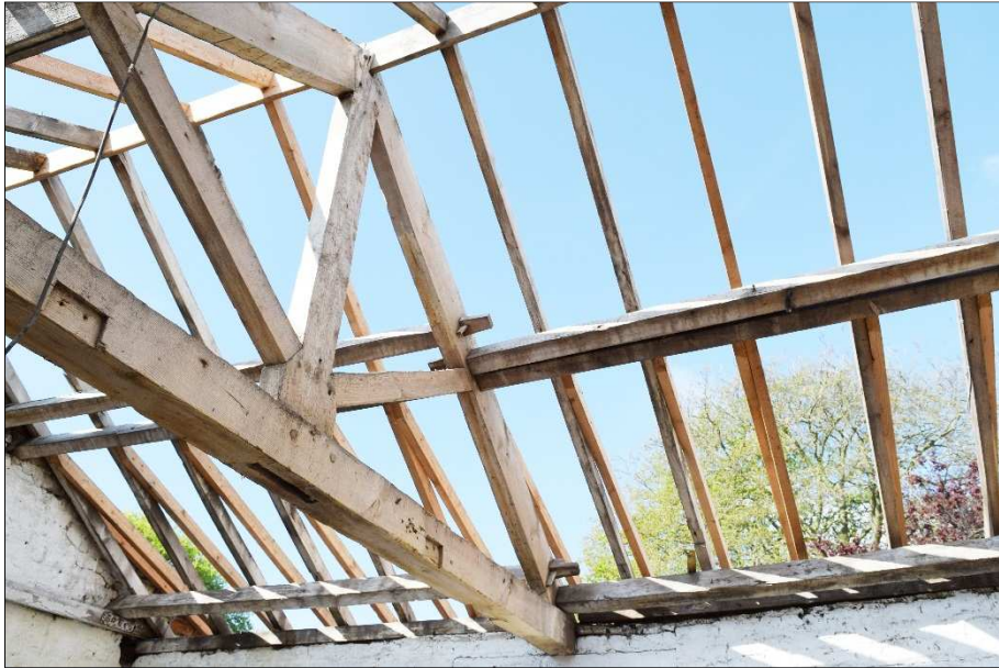
Plate 17 (shot 35): King post structure with pegged purlins
