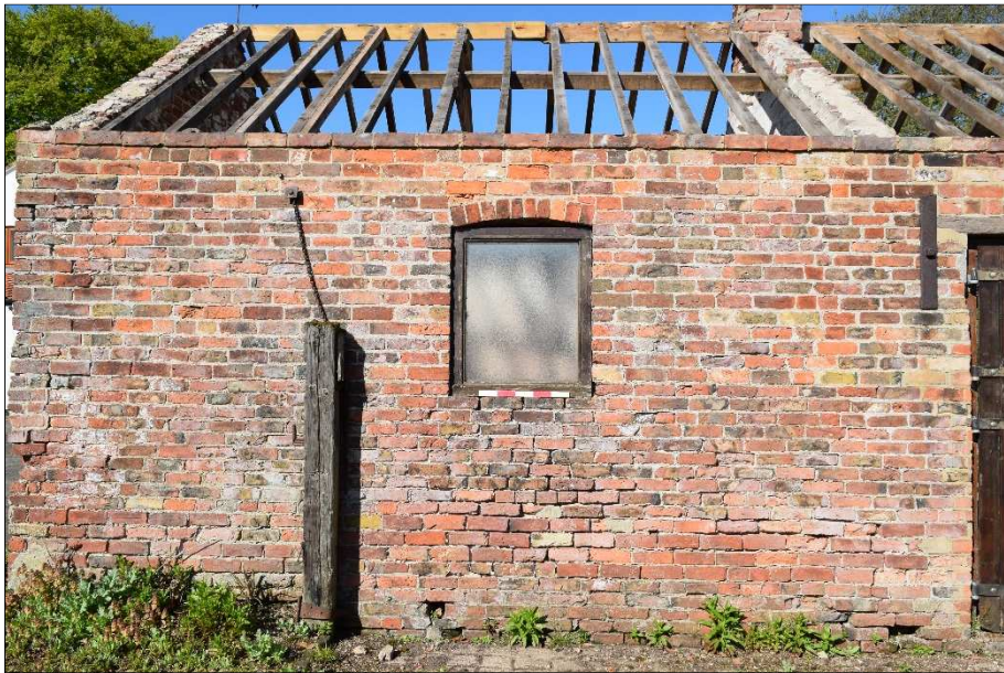
Plate 6 (shot 14): East-facing elevation of the south bay, showing window with segmental arch. Looking west, 0.5m scale
