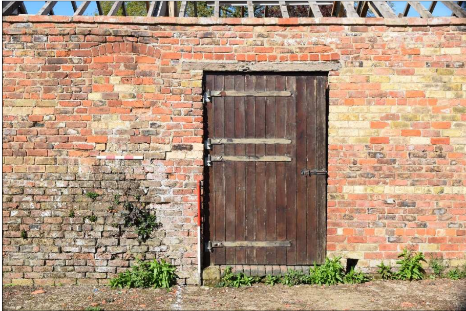
Plate 5 (shot 15): Representative shot of stable door, showing blocked window to the left and a small drain on the right hand side of the door. Looking west, 1m scale
