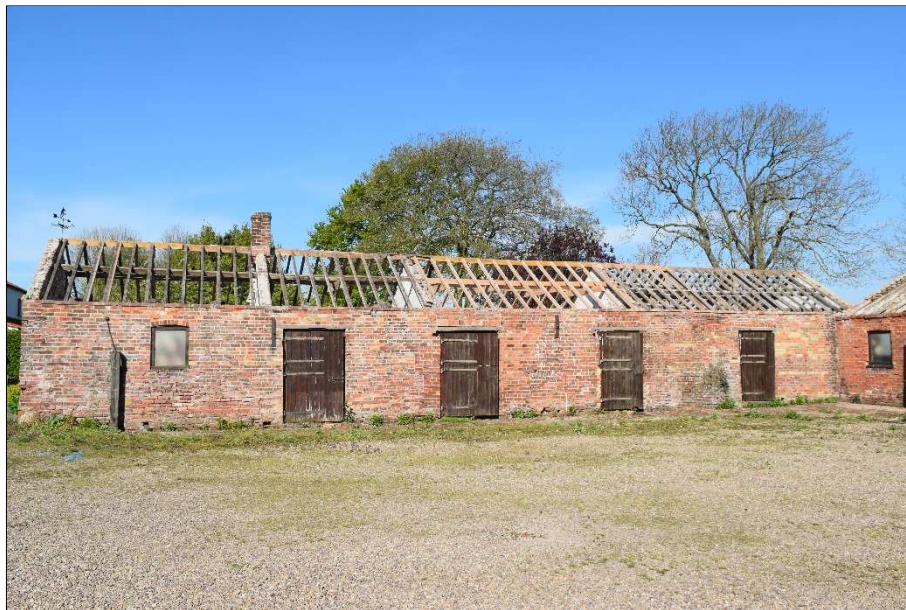
Plate 4 (shot 13): East-facing elevation. Looking northwest, 1m scale
