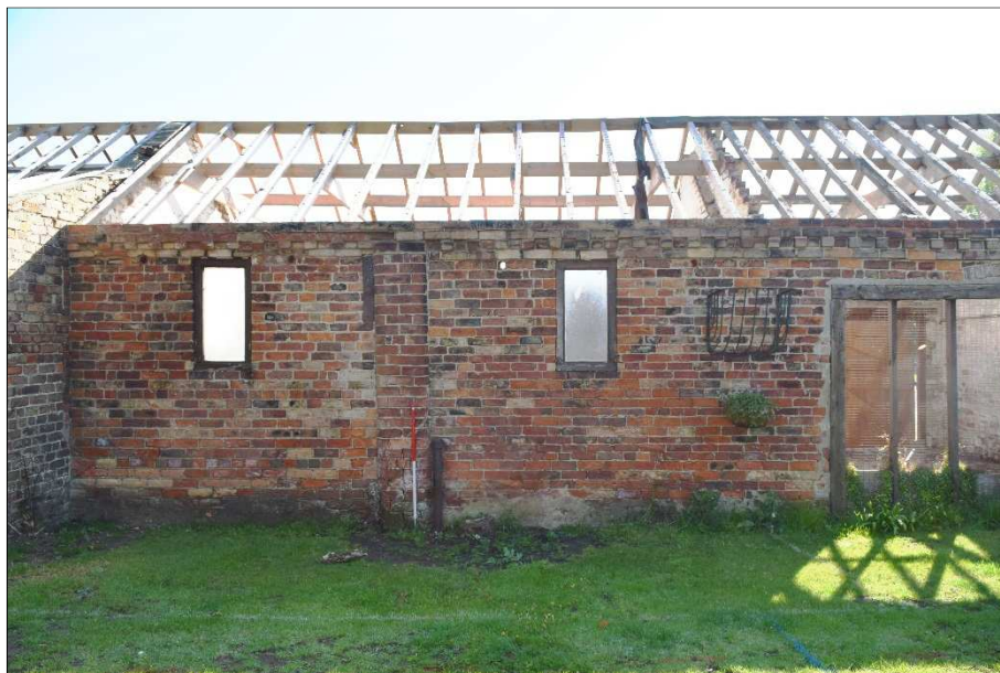
Plate 8 (shot 7): Former harness room to the right with modified opening and later windows to centre bays. Looking east, 1m scale
