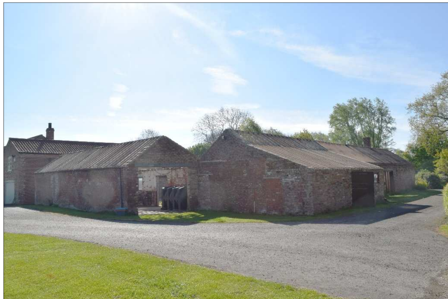
Plate 1 (shot 1): General view of Building A to the right and Building B to the left. Looking southeast, 1m scale
