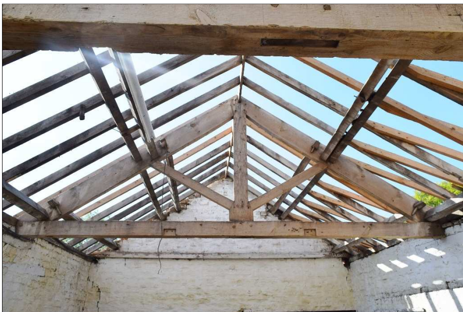
Plate 16 (shot 33): King post roof truss in the northern bay. Looking south
