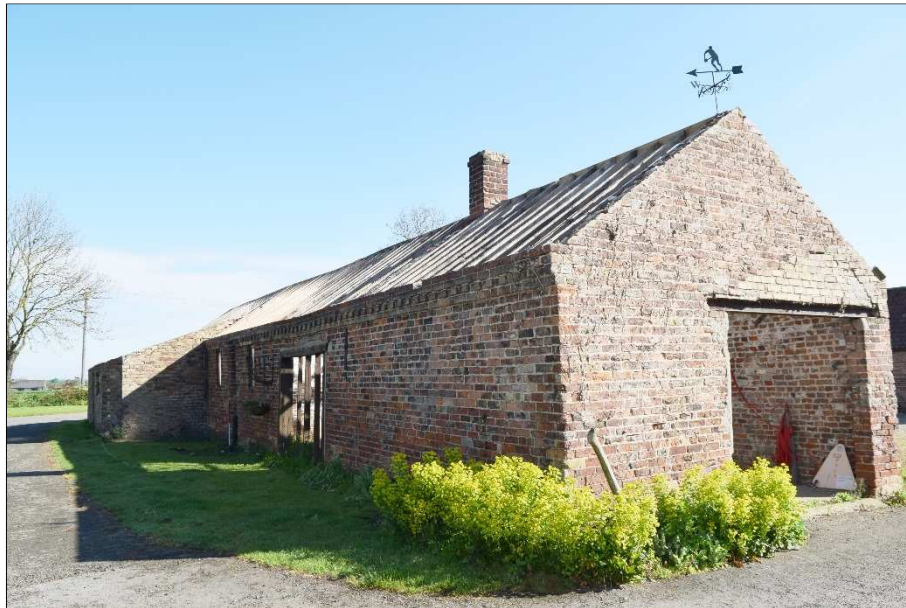
Plate 7 (shot 6): South and west elevations of Building A. Looking northeast, 1m scale
