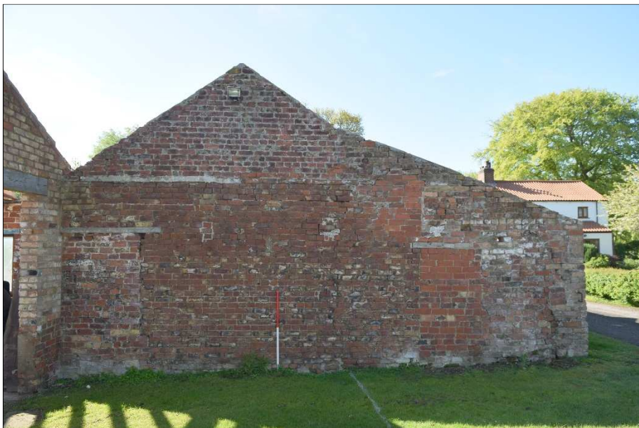
Plate 3 (shot 4): North-facing elevation showing blocked openings. Looking south, 1m scale
