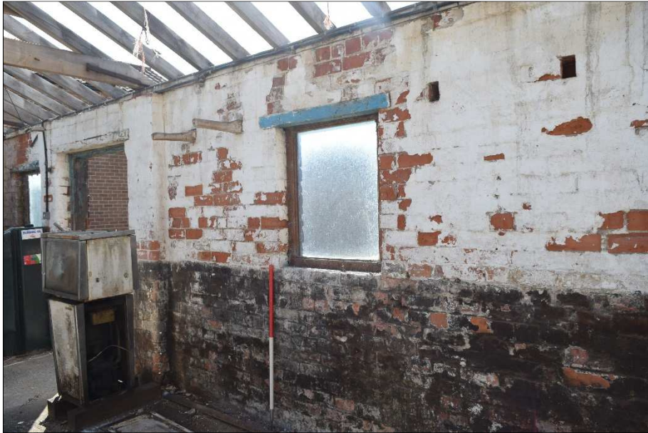
Plate 32 (shot 26): Saddle-trees on the south wall, notice the holes to the right where these have been removed. Looking southeast, 1m scale
