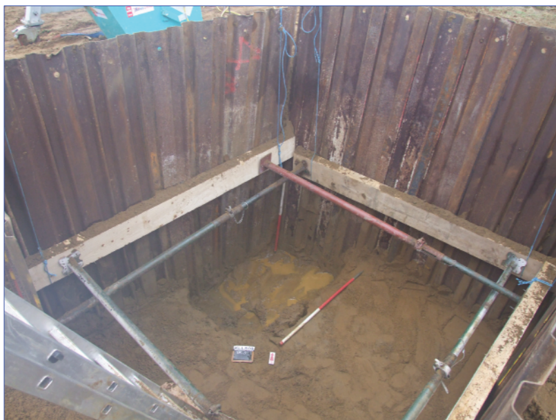
Plate 8: Trench 3 following machine-excavation and shoring, and hand-dug slot, looking south
