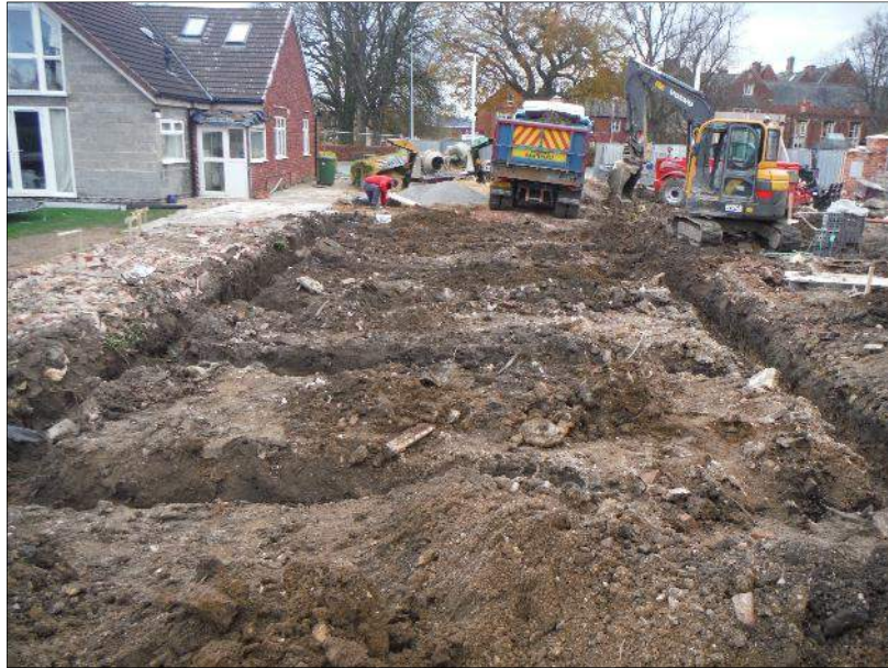
Plate 9: Plot 3 foundation trenches, looking east
