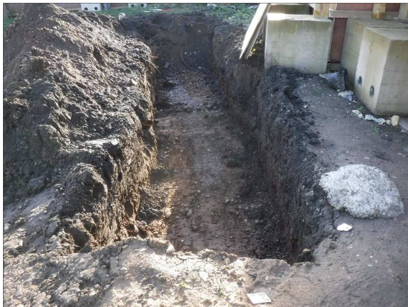
Plate 5: Trench 5, looking southeast 1m scale
