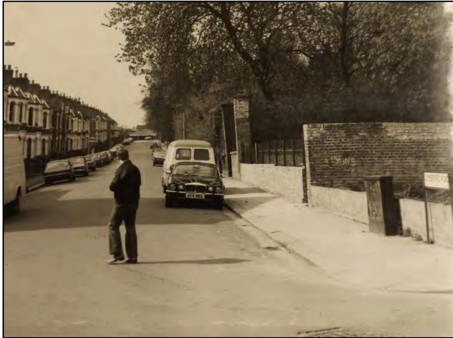
Plate 4: Limesford Road, looking west from the corner of Ivydale Road c.1982, note tilting pillars
