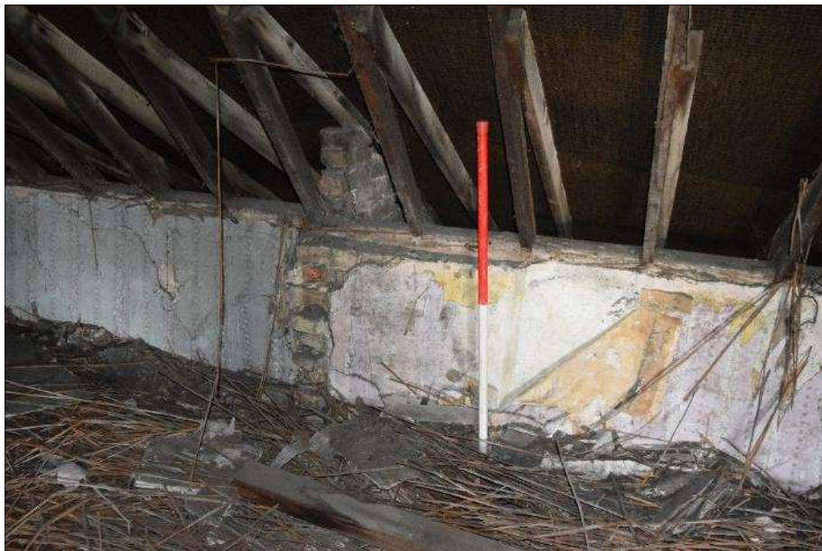
Plate 16 (shot 92): Stump of removed brick partition. Looking south, 1m scale
