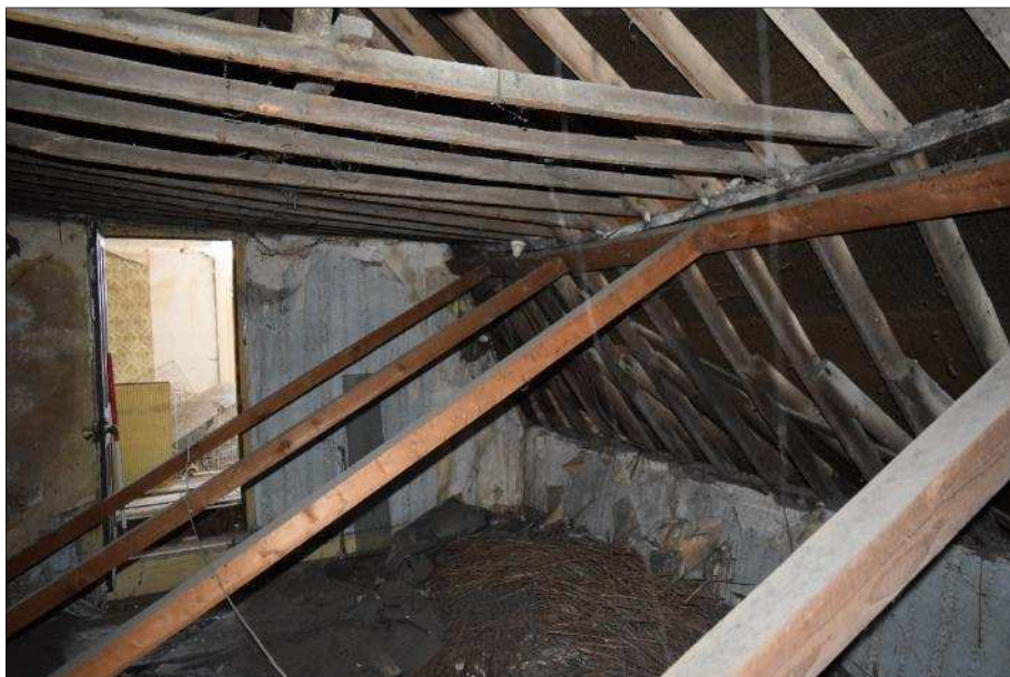
Plate 19 (shot 23): General view of later supports. Looking north-northeast, scale 1m
