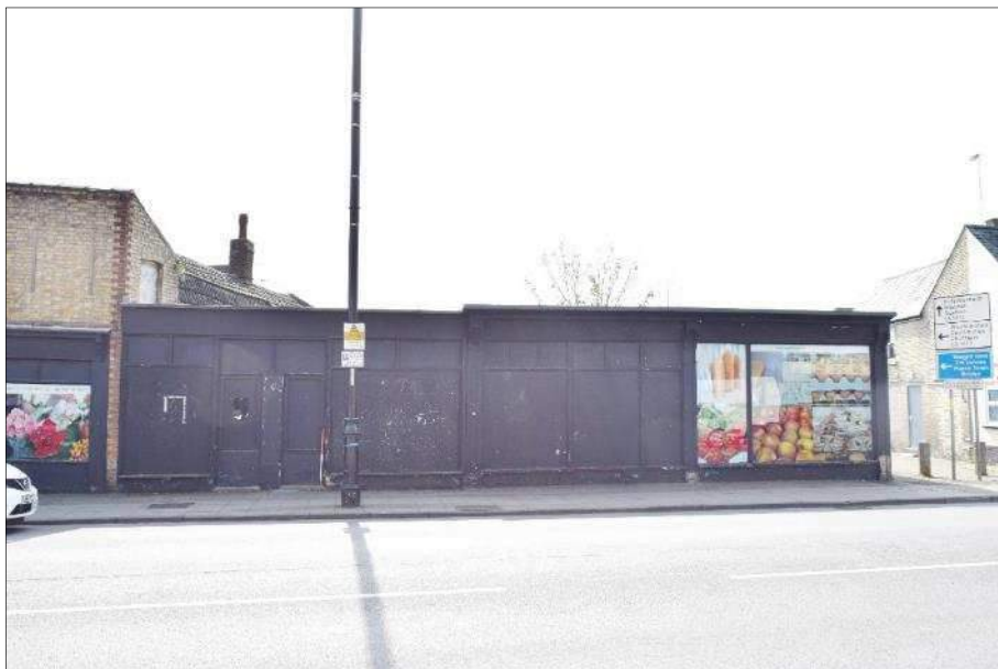
Plate 39 (shot 84): North elevation, shop frontage with black painted fenestration. Looking south, 1m scale
