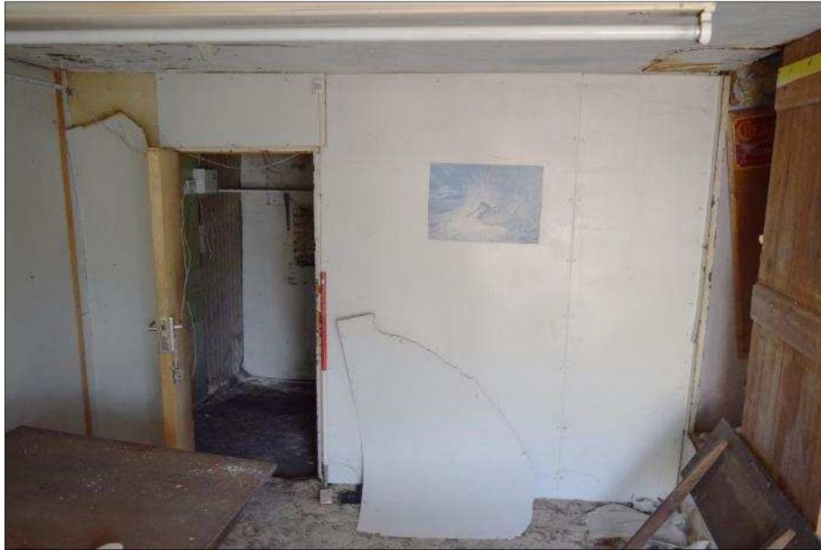
Plate 22 (shot 18): Modern stud wall and door. Looking east-southeast, 1m scale
