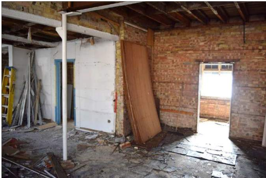
Plate 54 (shot 56): General view of the south wall with access to F and modified north-south partition. Looking south-southeast, 1m scale
