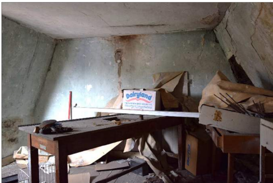
Plate 10 (shot 1): General view of first floor. Looking northeast, 1m scale
