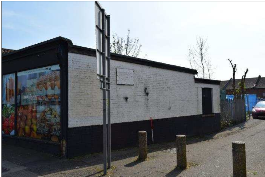
Plate 40 (shot 86): West elevation with extension E visible to the right. Looking south, 1m scale
