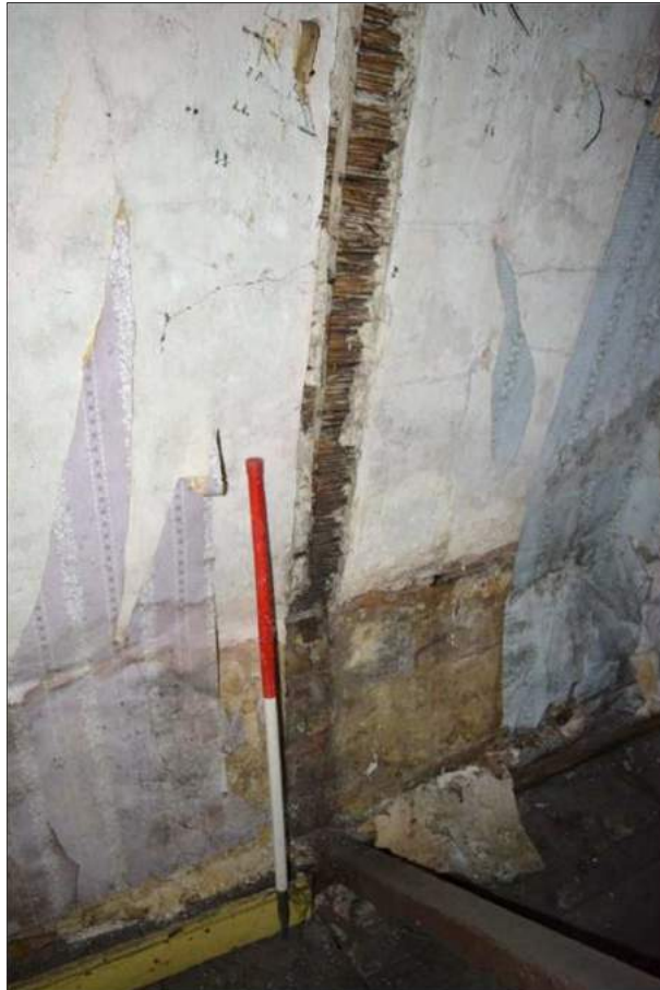
Plate 17 (shot 93): Scar from removed partition, exposing reeds behind the plaster. Looking west-southwest, 1m scale
