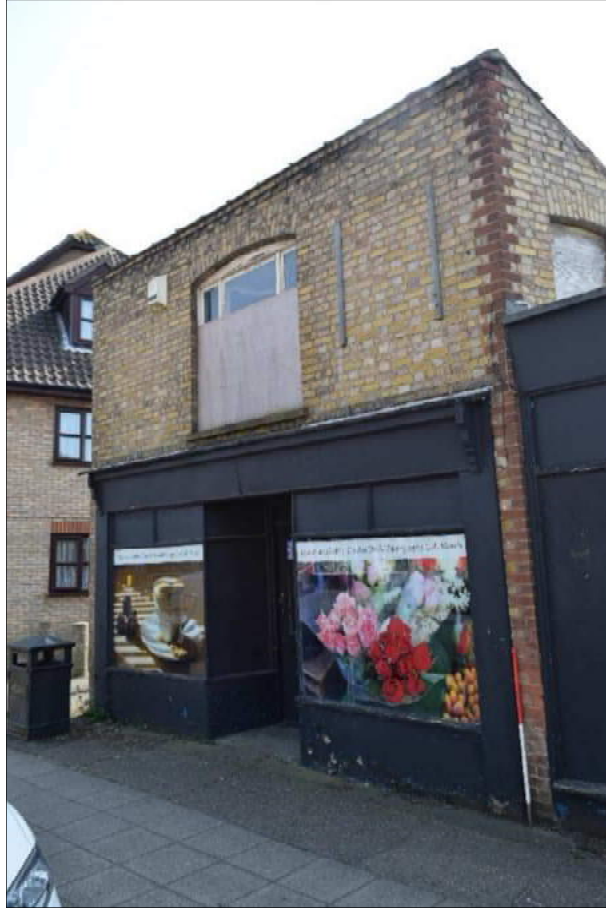
Plate 33 (shot 85): General view of north elevation. Looking southeast, 1m scale
