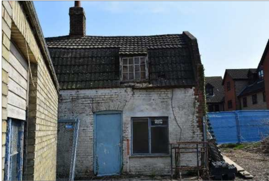
Plate 6 (shot 67): East elevation and representative view of doors and windows. Looking east, 1m scale
