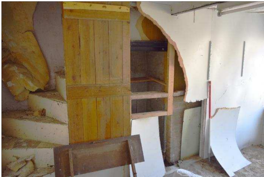
Plate 23 (shot 14): Staircase to first floor south room, fireplace behind modern stud and boards. Looking south, 1m scale
