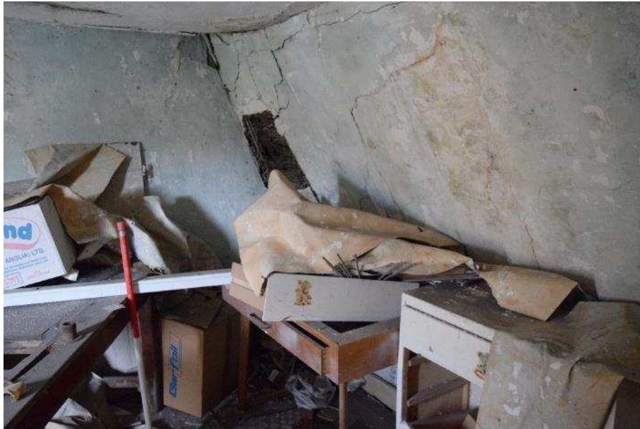
Plate 11 (shot 8): View of plastered ceiling and walls, an inspection hole revealing reeds behind the plaster. Looking southeast, scale 1m
