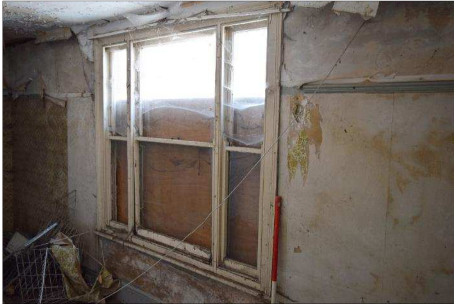
Plate 38 (shot 26): Original sash window in Structure C. Looking northwest, 1m scale
