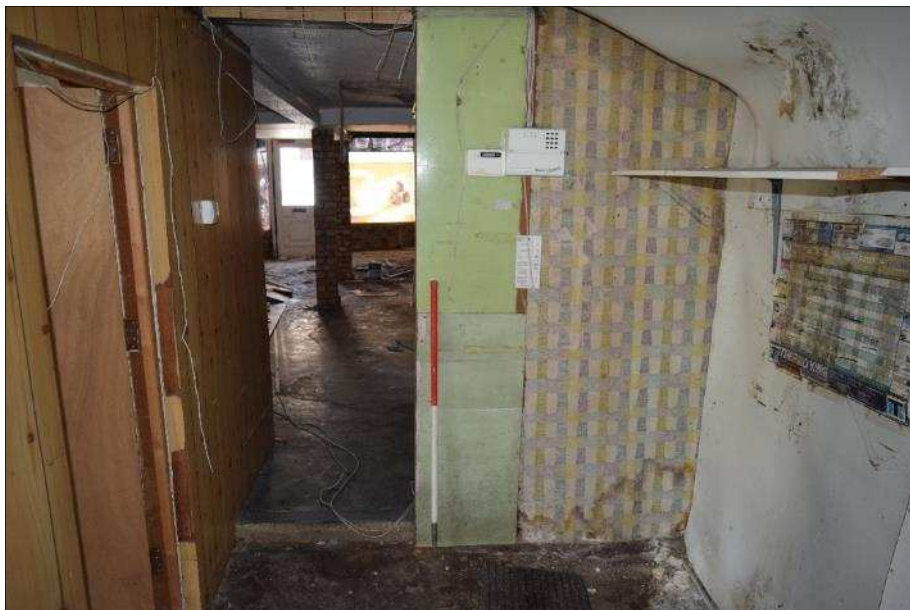
Plate 25 (shot 21): View of Structure B ground floor, looking north-northeast, 1m scale
