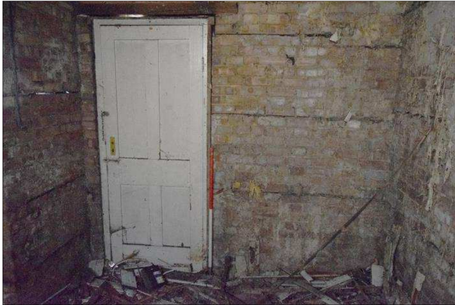
Plate 53 (shot 61): Extension E, general view. Looking east, 1m scale
