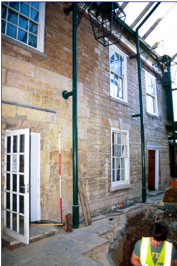
Plate 6: (026) Eastern elevation of the Western Range (South Block) illustrating the changes in wall fabric associated with phases of development. Looking north-west
