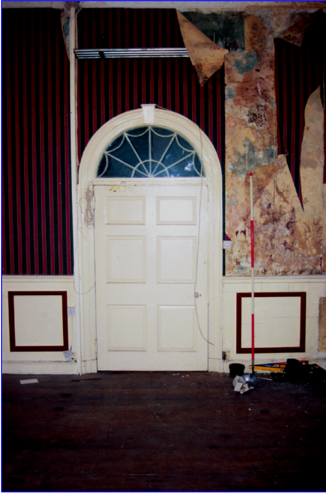
Plate 15: (036) The courtroom is accessed via a six panel door with an Adam Style fanlight header, framed by architrave with keystone detail on both sides of the door frame. This shot also demonstrates the level of water damage to the interior of the building. Looking east.
