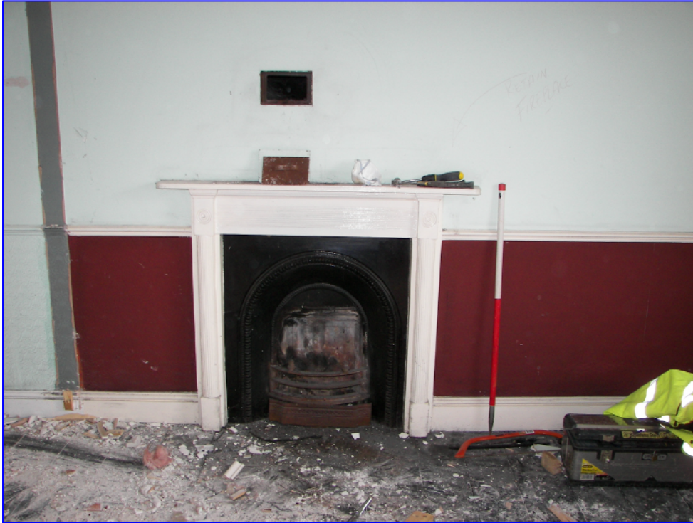
Plate 9: (shot 113) Room 16 retains a mid 19 th century cast iron arched register grate that has a Regency style fire surround with concentric bosses and reeded moulding. Looking east.
