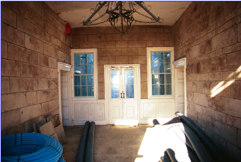
Plate 16: (030) The ashlar lining applied to the carriage arch in 1789. The northern end is filled by a 19 th century brick wall, door and windows, with imitation stone dressing over panelling applied the interior wall. Looking south.
