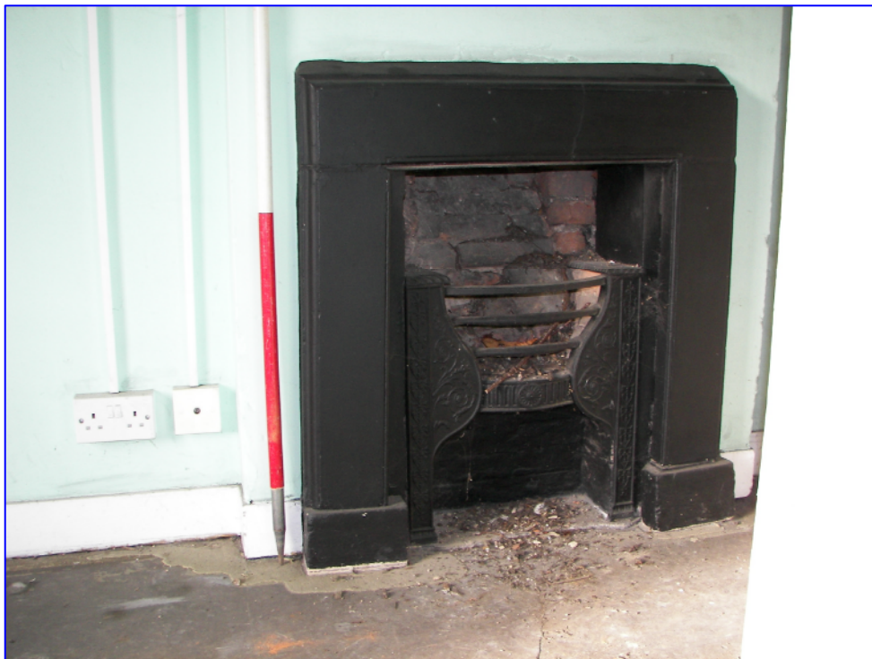
Plate 10: (123) Room 18 retains a late 18 th early 19 th century cast iron hob grate with a plain stone surround. The same style of fireplace has been retained in rooms 19, 20 and 21. Looking north-north-west.
