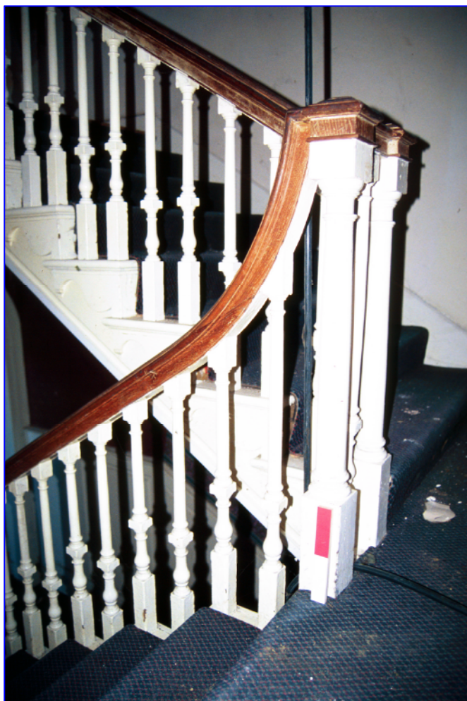
Plate 13: (097) Constructed in an open strung mid Georgian style, the eastern staircase has slender turned balusters standing on the treads with columnar newel posts and ramped handrail. Looking south-west.
