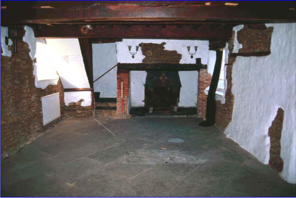
Plate 21: (047) Room 8, in the Western Range. At the northern end of the room is a broad 17 th century style fireplace with a heavy timber bressumer supported on 2 1/4 inch brick piers. Adjacent to the fireplace is the staircase to the garret room above. Large timber cross beams support the joists for the garret floor. Looking north.
