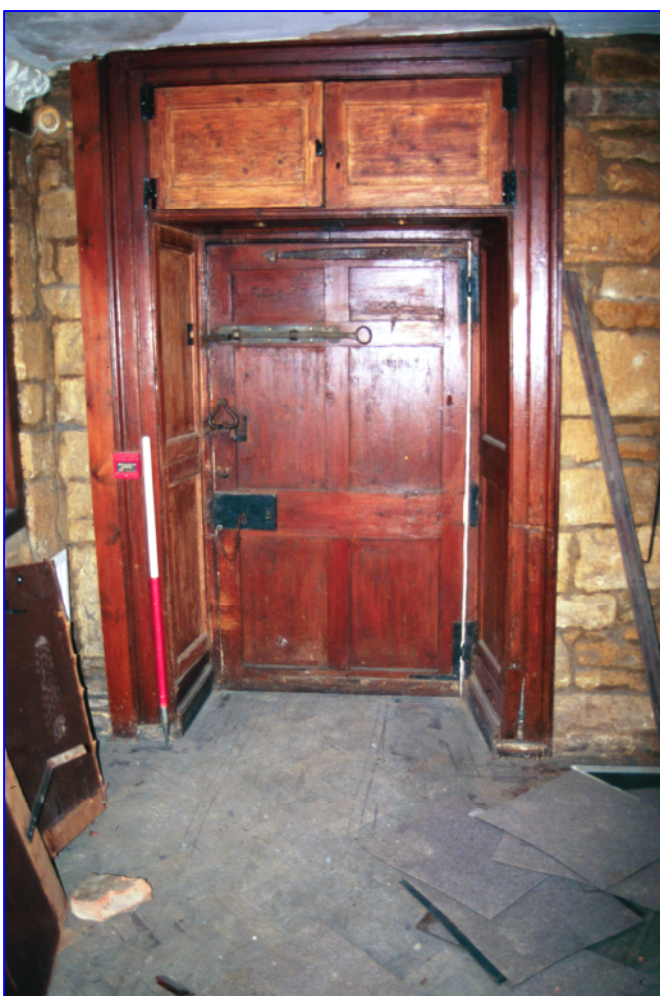
Plate 20: (055) Room 6, mid 18 th century style six panelled door with L shaped hinge and contemporary iron work. The door is set within panelled jambs below a built in cupboard. Looking east.
