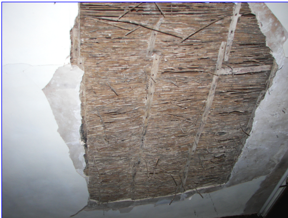
Plate 19: (057) The reeded ceiling exposed in Room 6.
