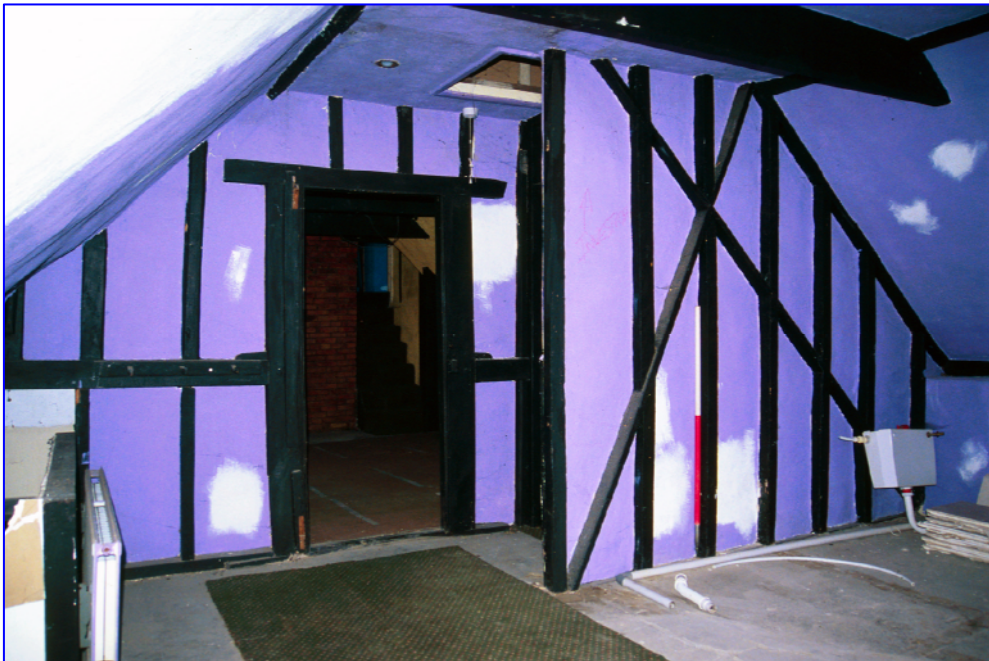
Plate 26: (085) Room 15. The 18 th century type doorframe in the southern wall of this room is constructed in heavy timbers that form part of the roof superstructure. It has an expanded lintel that is secured to the jambs with pegged mortice and tenon joints supporting timber studding to the apex of the roof. An original latch hoop is still attached to the north side of the frame. A partition wall of timber uprights with cross bracing may have enclosed what may have been the original internal staircase access. Looking south-east.
