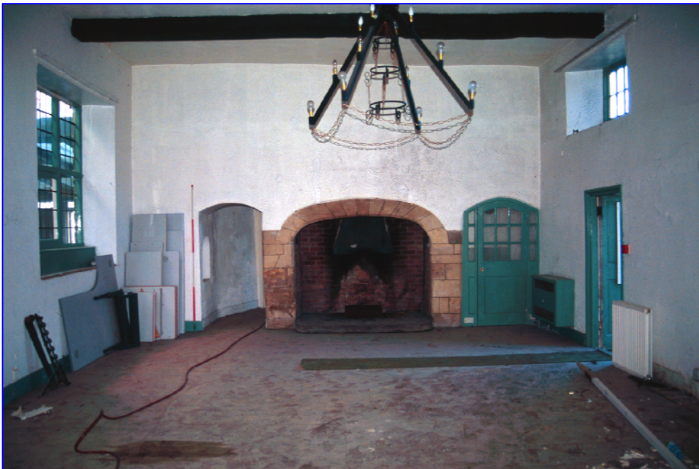
Plate 24: (038) Room 2. In the north wall is a large 18 th century basket arched fireplace with integral moulded stone surround and buttresses over an integral stone slab. There is an arched recess to the east of the fireplace with a half glazed nine pane door flanked by narrow three light sashes. The arch to the west passes through a former oven set into the corner of the building with an external curved wall. Looking north.
