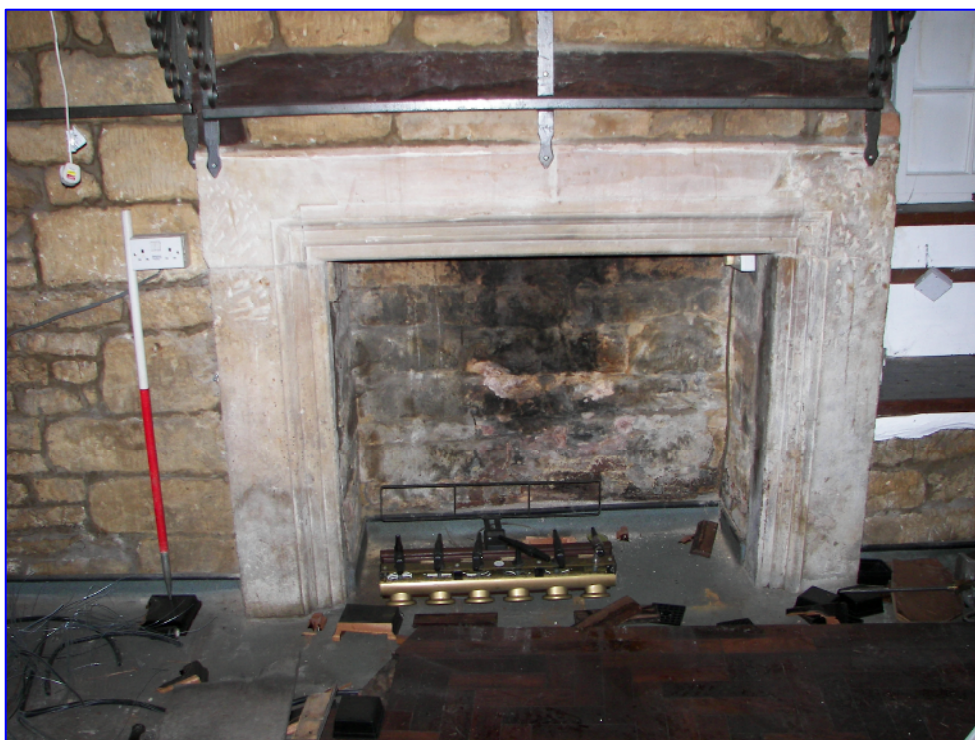
Plate 18: (056) Room 6 in the Western Range, 17 th century open fireplace with a stone surround. Looking west.
