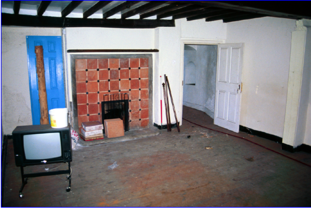
Plate 25: (041) Room 3 has a beamed ceiling with a large cross beam supporting squared timber joists, with a further beam set into the chimney breast crossing a recess on its eastern side. There is a tile backed modern retro fireplace incorporating iron studs and a small grate fitted to the chimney breast on the south wall. The floorboards are also a relatively recent addition to the building and the internal doors are modern replacements. Looking south-east.
