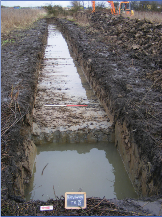
Plate 4: Trench 3 after machine excavation, looking east from west end of trench.
