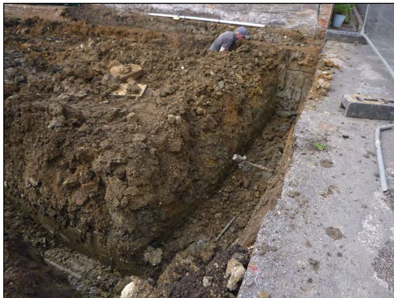
Plate 1: Unit 1, representative section, looking southwest
