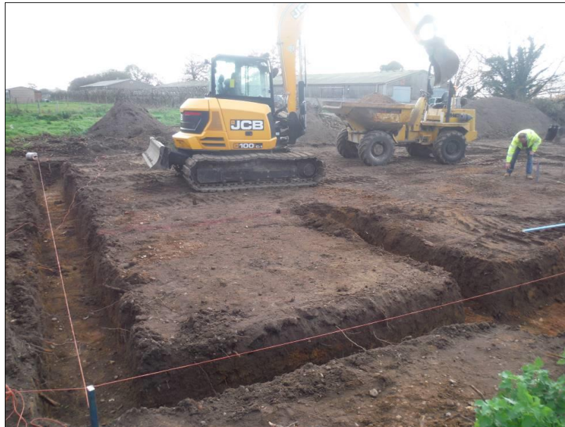
Plate 1: General shot of the works in Plot 1 looking southwest
