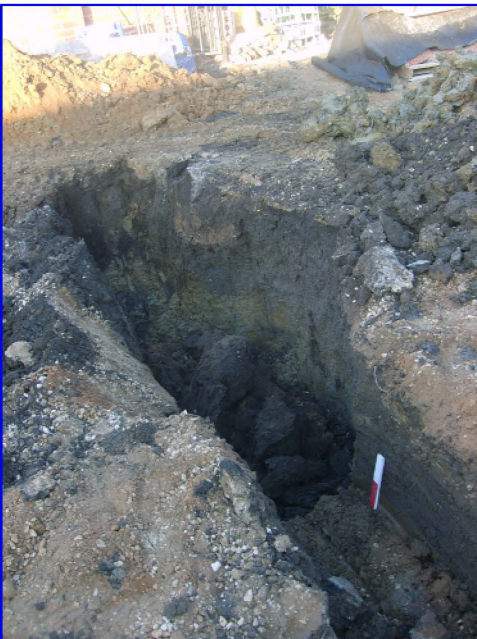
Plate 2: The eastern end of the drainage trench, looking north-west.
