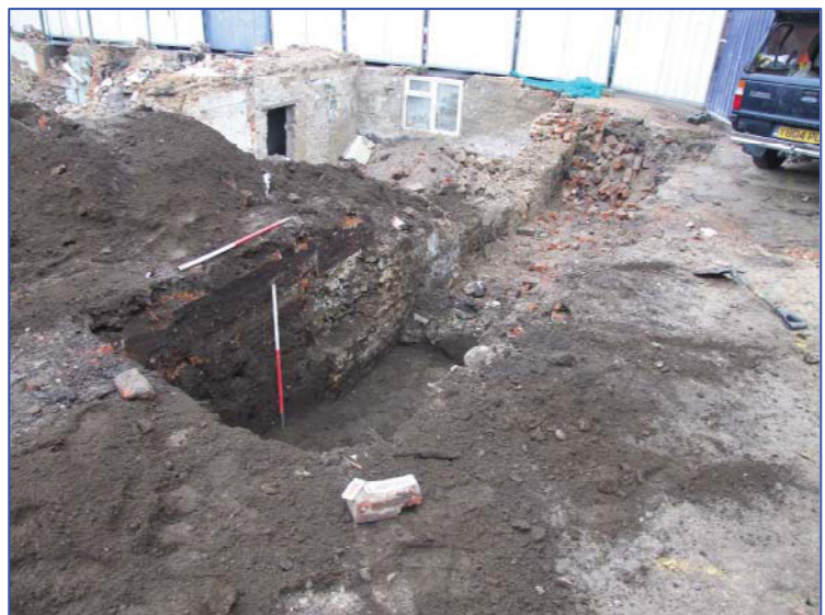
Plate 5: West facing section of Trench 2 showing the extent of the backfilled cellar in the southern part of the trench. Shot taken looking south-east.
