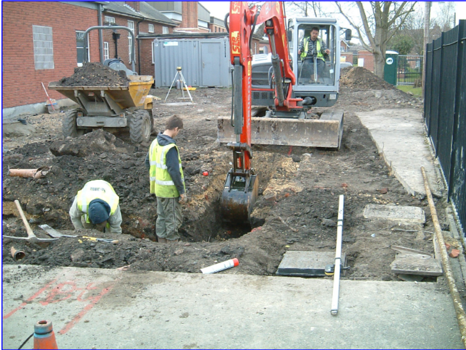
Plate 1: General working shot of the development area looking north-west.
