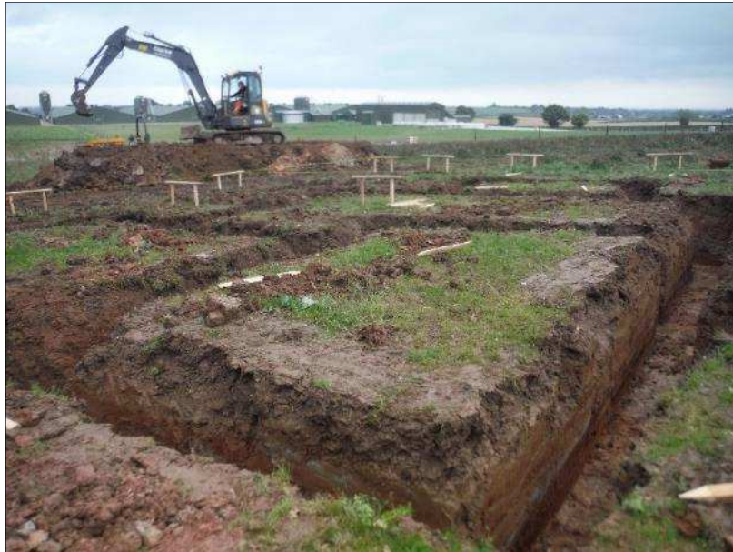
Plate 1: The house footings, looking northeast
