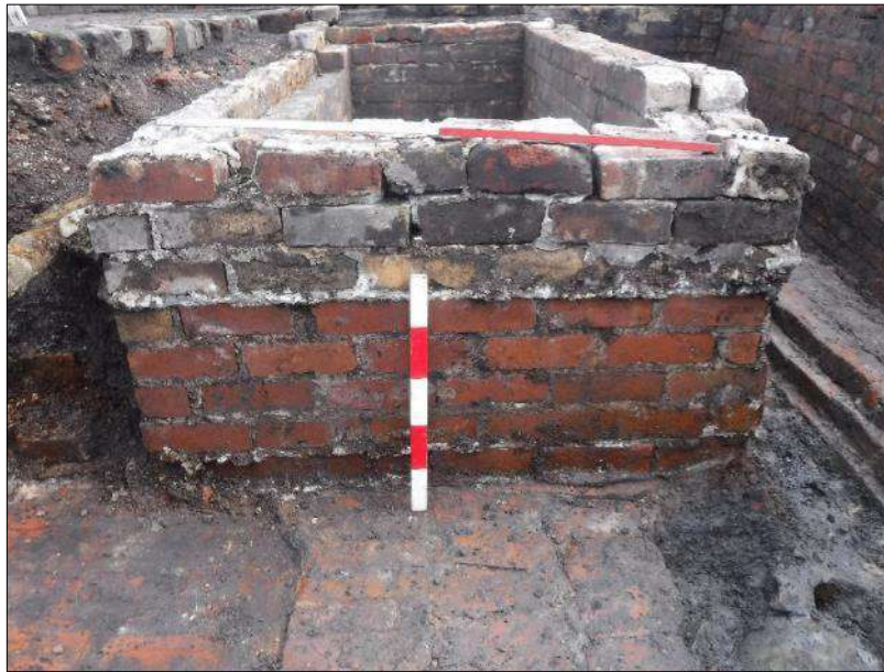
Plate 56: southwest facing elevation of structure 315, showing distinct construction phases, 1m and 0.5m scales
