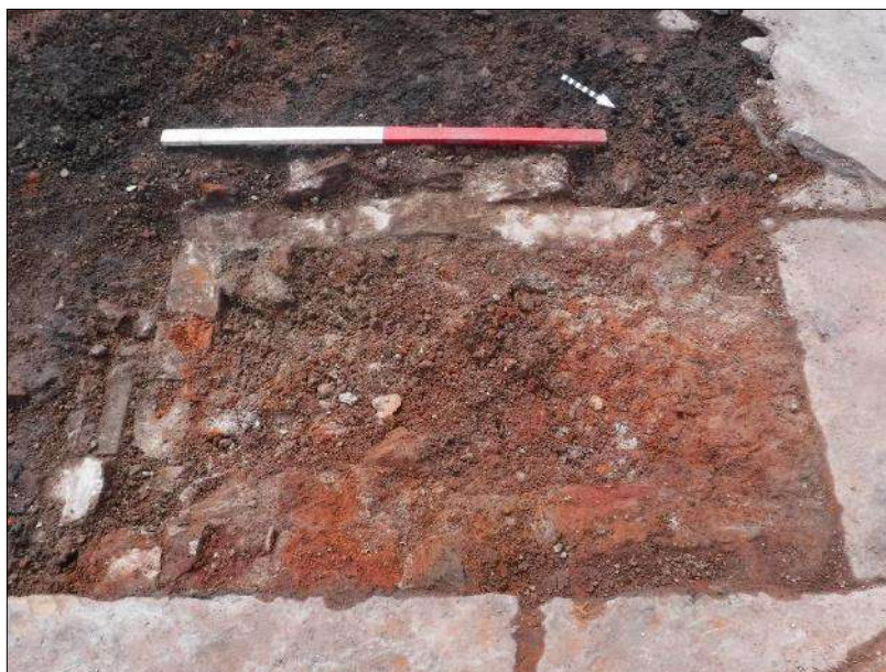
Plate 32: Foundation 129, 130 of newel within stair tower, 1m scale
