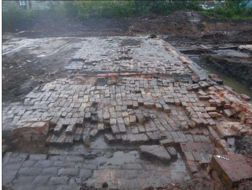
Plate 60: Boiler house showing unbonded brick surface 269 within southeastern bay, looking northeast, 2m and 1m scales
