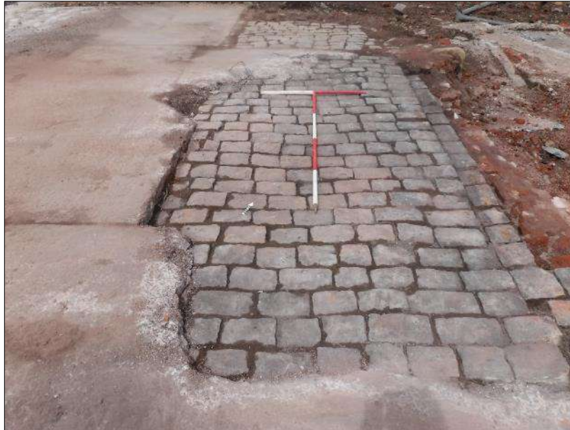
Plate 38: Road surface 120, looking northwest, 2m and 1m scales
