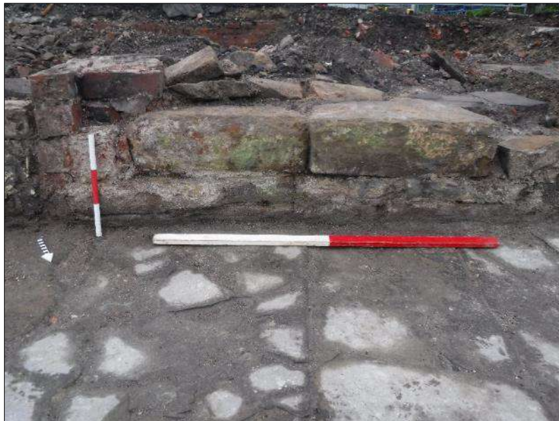
Plate 4: Northeast facing elevation of wall 209, looking southwest, 1m and 0.30m scales
