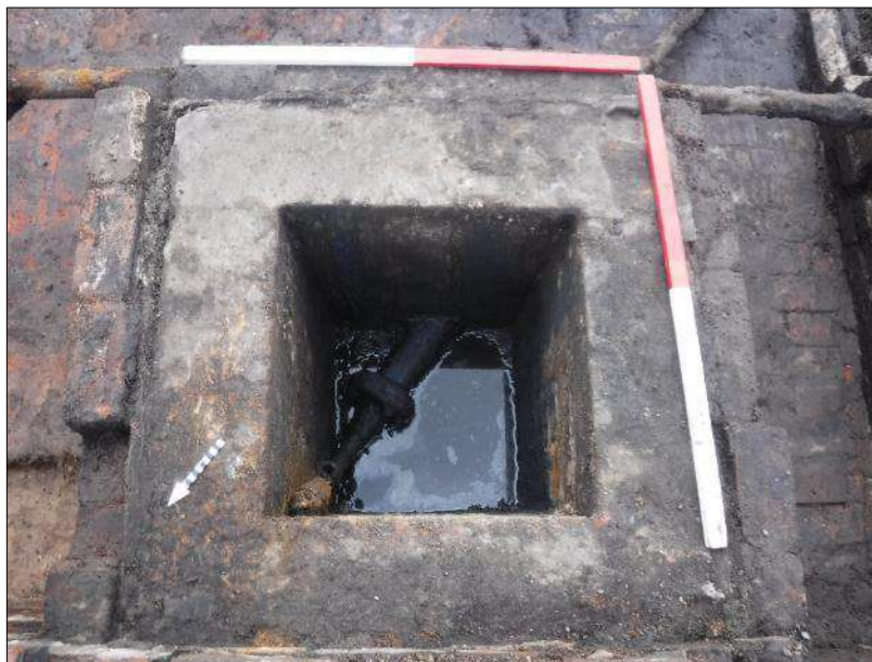
Plate 58: Post excavation shot of structure 319, showing pipe 335, 1m scales
