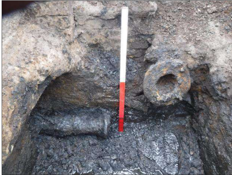
Plate 44: Detail of pipework at northeastern end of cold well, looking northeast, 1m scale
