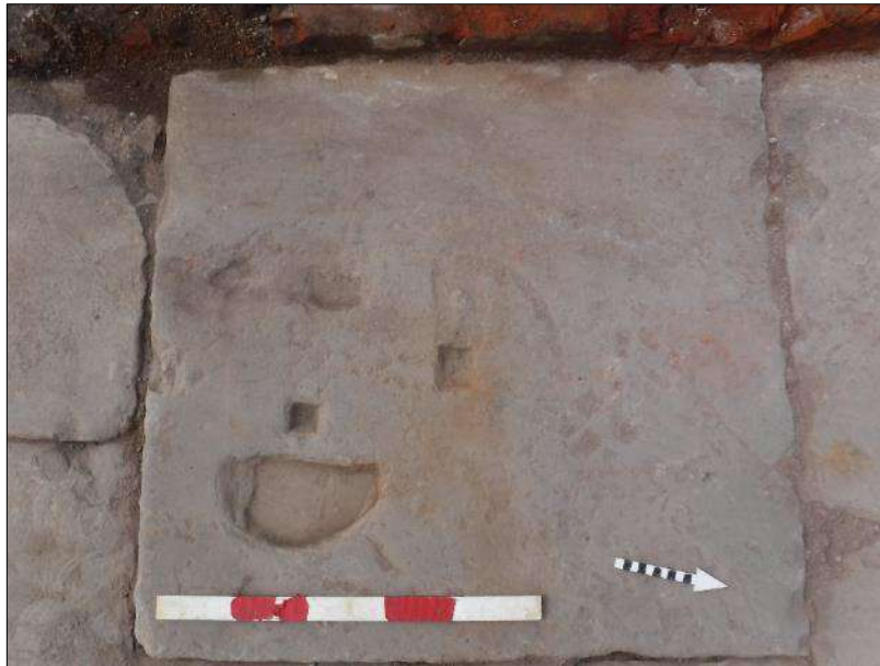
Plate 26: Example of features associated with machine bases, cut into flagged floor 158, 0.50m scale
