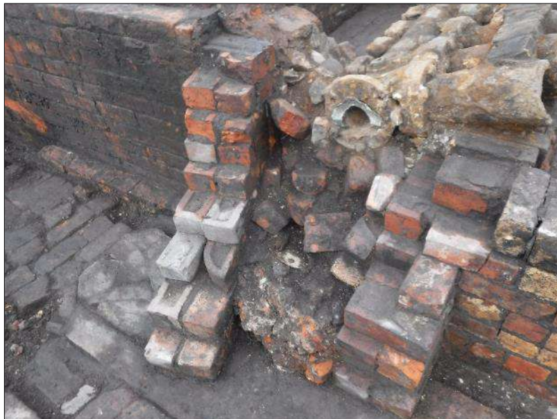
Plate 70: Southwestern flue exiting boiler house through wall 325, looking south
