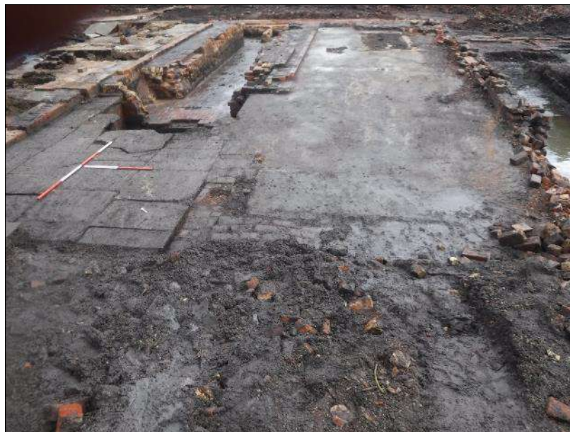
Plate 59: Boiler house showing concrete floor surface 328 within southeastern bay, 2m and 1m scales
