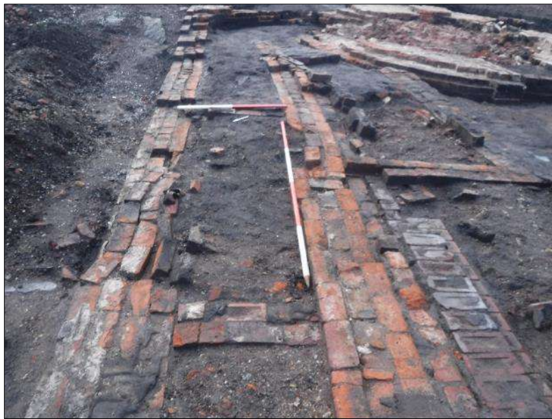
Plate 66: Overall view of flue system connected to chimney 249, 2m and 1m scales
