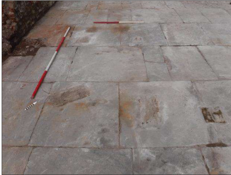
Plate 23: Detail shot of flagged floor surface 158 showing timber inserts, 2m and 1m scales
