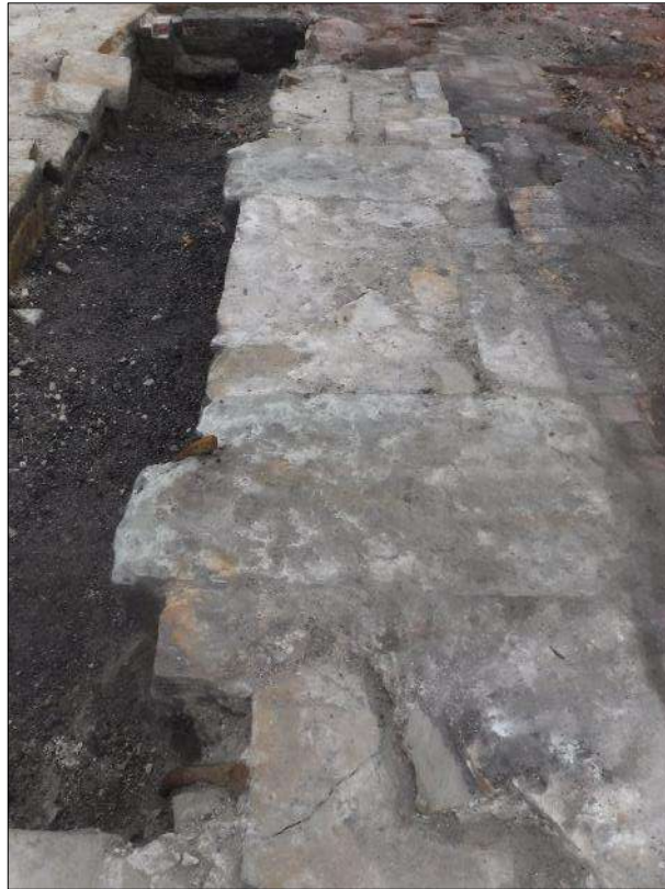
Plate 42: Masonry 181 within engine house showing sandstone slabs 184 and 185, looking northwest
