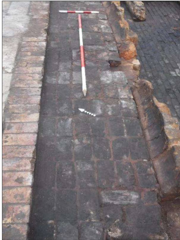
Plate 48: Bench 298 showing boiler mounting blocks 299 to the right, looking northeast, 2m and 0.5m scales
