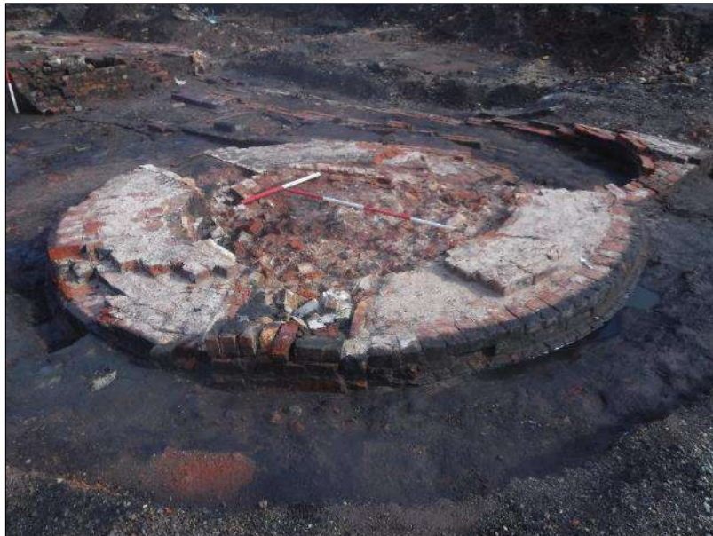
Plate 62: General shot of Chimney 249 and flue system leading to boiler house beyond, looking north, 2m and 1m scales
