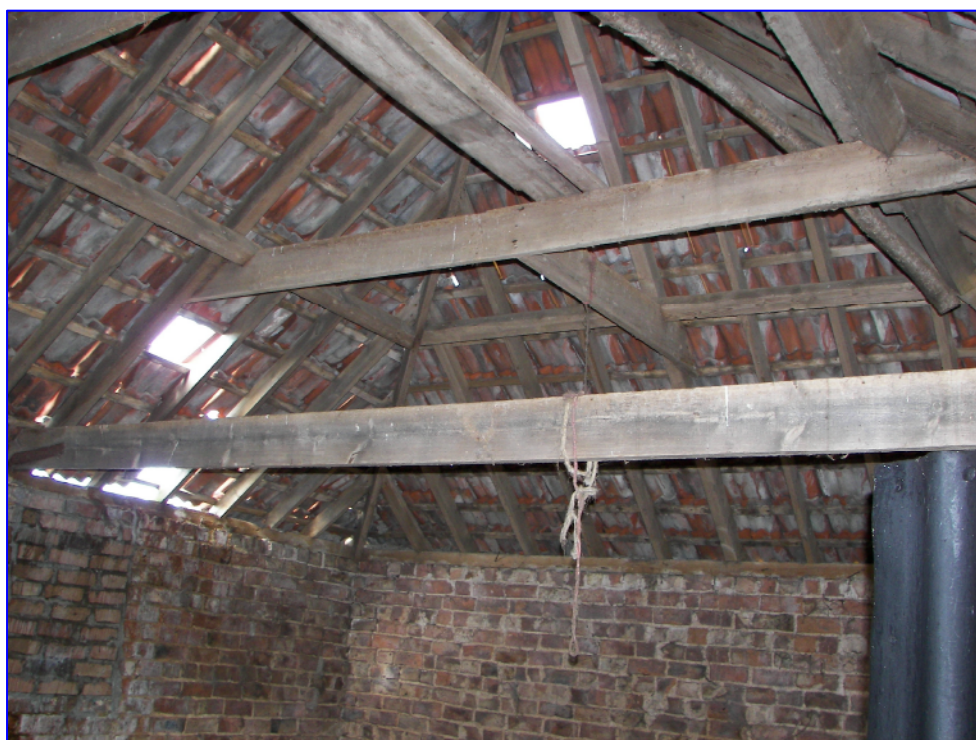
Plate 14 (Shot 25): General shot of the hipped roof construction looking south-west.
