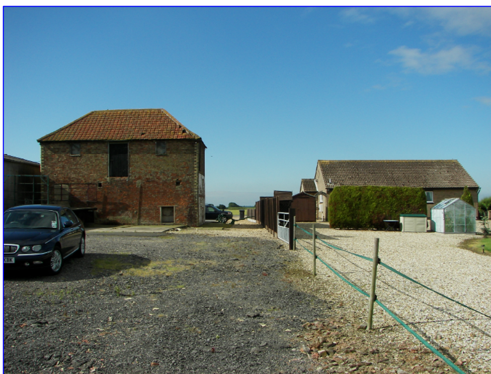
Plate 8 (Shot 13): The north-east facing elevation looking south-south-west and showing the rear aspect of the barn and surrounding buildings.
