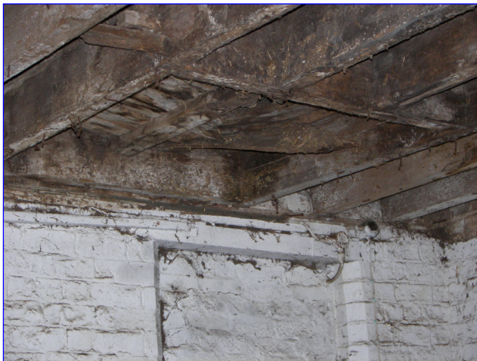
Plate 11 (Shot 31): A blocked opening in the first floor joists that formerly housed an internal staircase. The opening is located in the north-east corner of the barn over the blocked external doorway, the shot was taken looking north-east.
