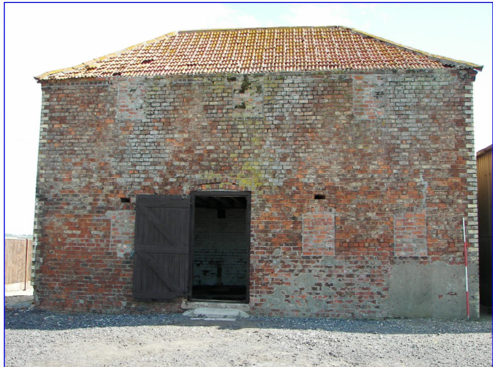
Plate 2 (Shot 5): The south-west facing elevation showing the blocked in windows on the ground and first floors. Looking north-east.
