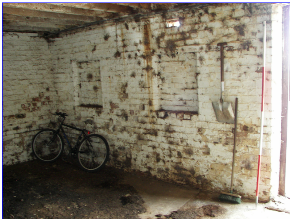
Plate 10 (Shot 20): The north-east facing interior ground floor elevation viewed looking south.
