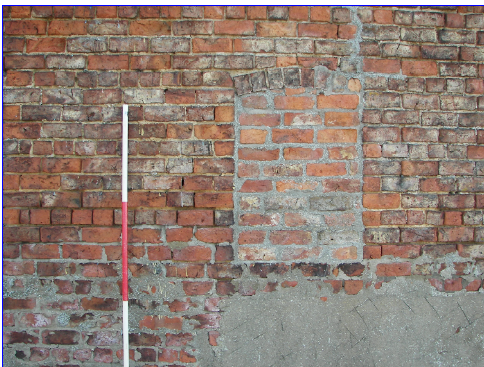
Plate 3 (Shot 6): Detail shot of a blocked in window on the ground floor of the south-west facing elevation, looking north-east.
