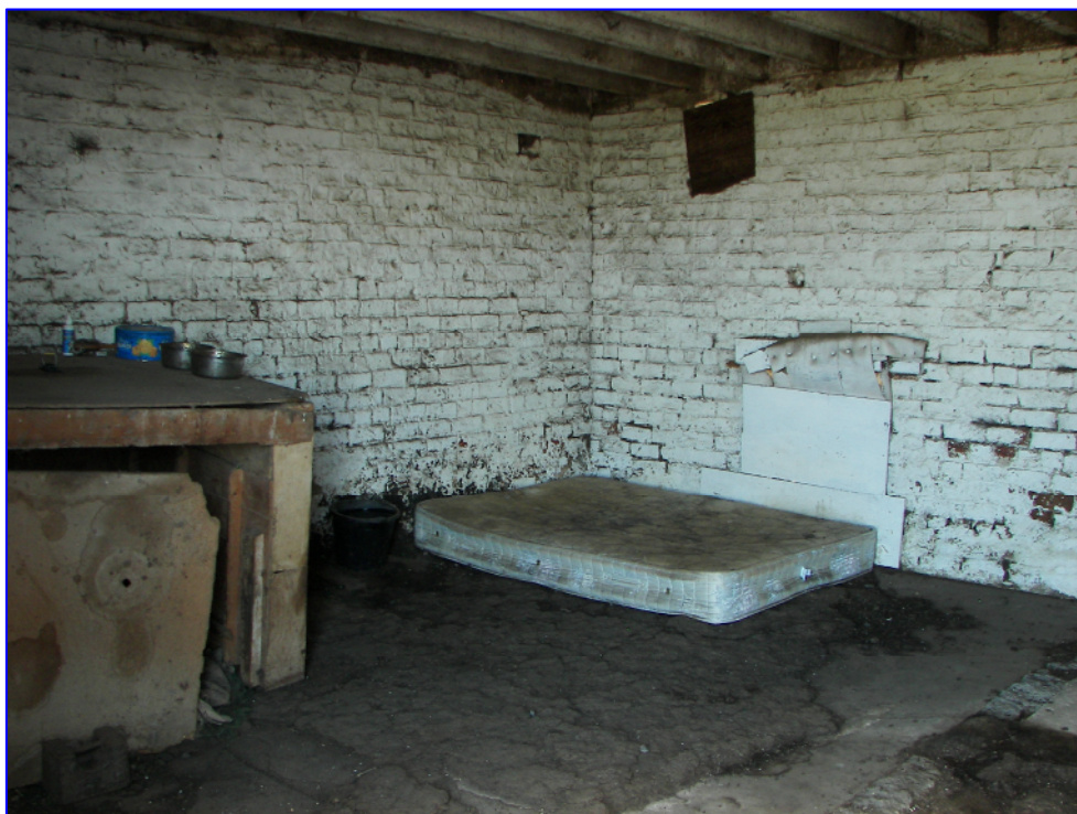
Plate 9 (Shot 17): The ground floor interior of the barn, looking north.
