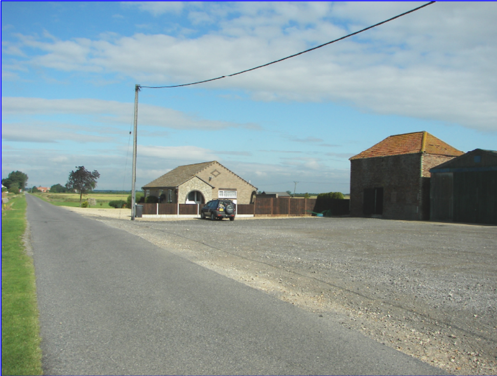
Plate 1 (Shot 2): The setting of the barn, viewed looking north-west along the adjacent lane.
