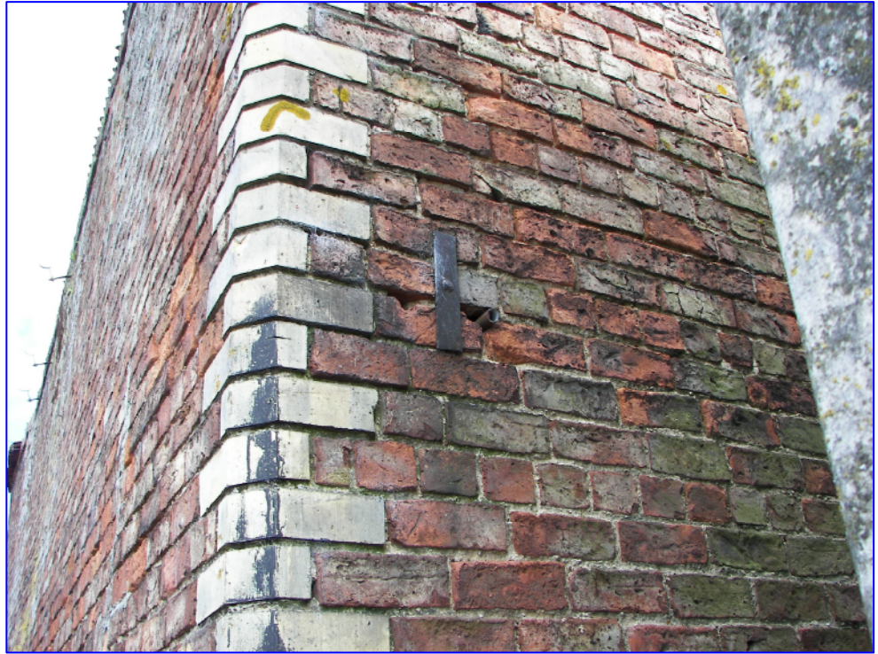
Plate 5 (Shot 24): Shot taken looking north-east of the south-west corner of the barn showing the polychrome detailing using single cant bricks in a gault fabric at the corners of the barn. To the right is a simple tie plate.
