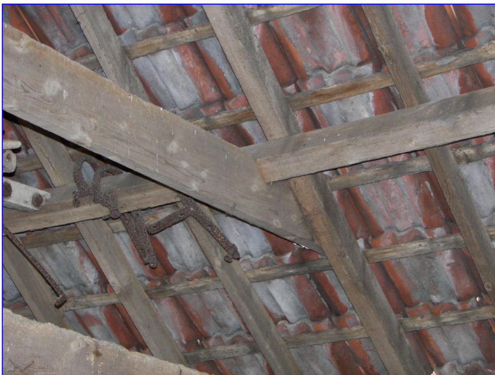
Plate 13 (Shot 30): Detail of the clasped purlin construction of the roof timbers, viewed looking south.
