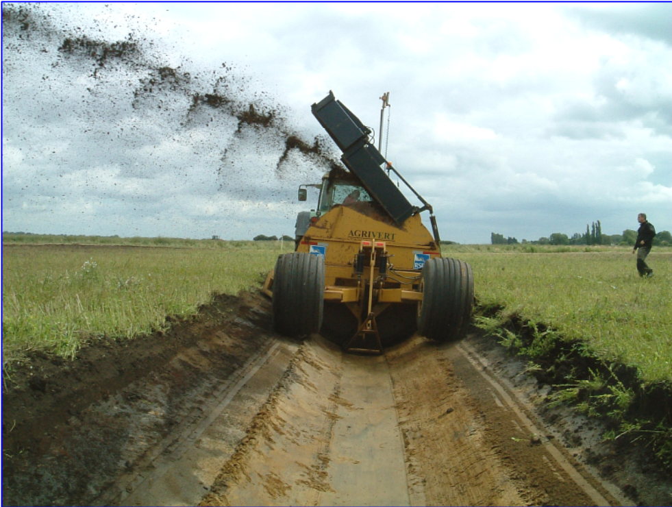
Plate 1: A shot looking east along Area 1, showing the RSPB ditch-cutting machine at work
