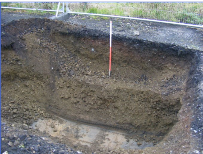
Plate 6: West facing section of Soakaway B, looking north-east
