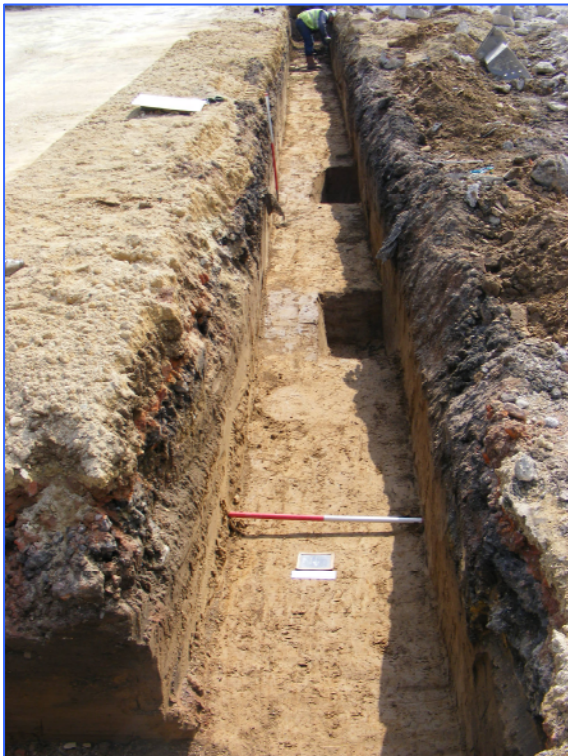
Plate 2: Shot taken looking south from the north-west corner of the foundation trenches, and showing sections through ditches [108] and [110]
