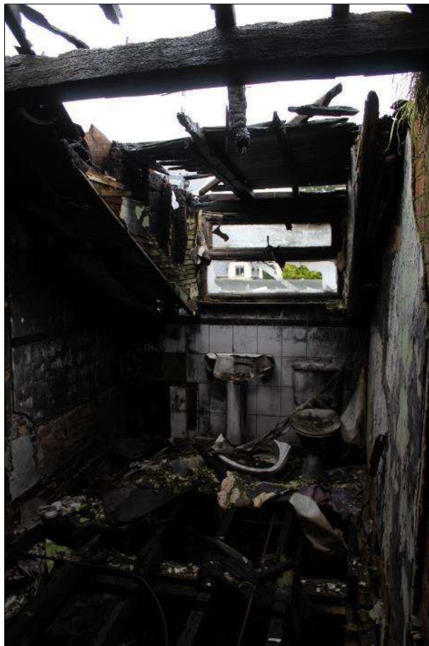
Plate 18 (shot 74): General view of first floor bathroom, looking north
