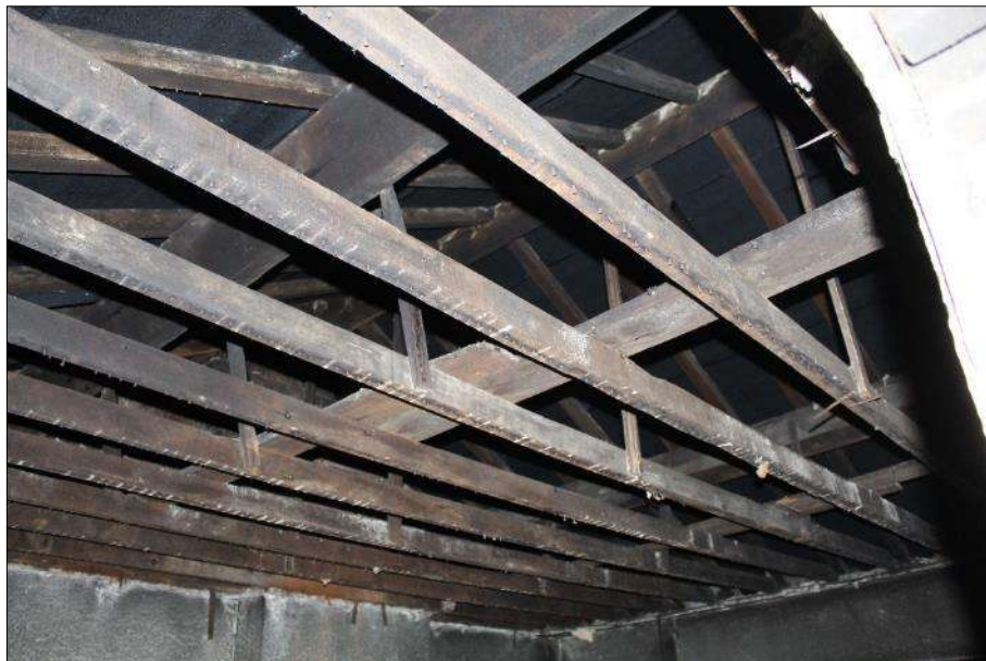
Plate 12 (shot 71): Representative view of the roof above Structure A. Looking southwest
