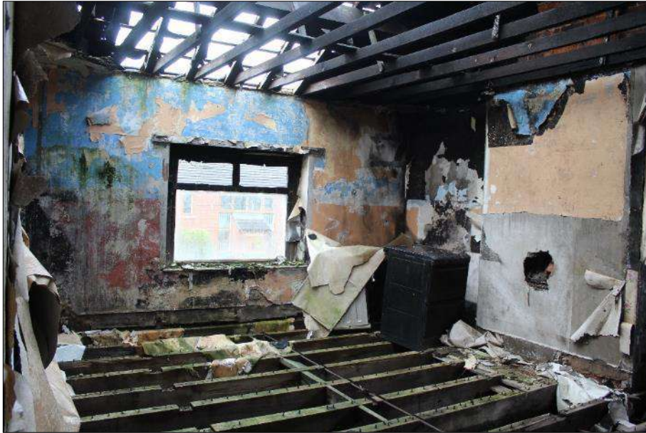
Plate 9 (shot 66): General view of upstairs northern room, looking northwest
