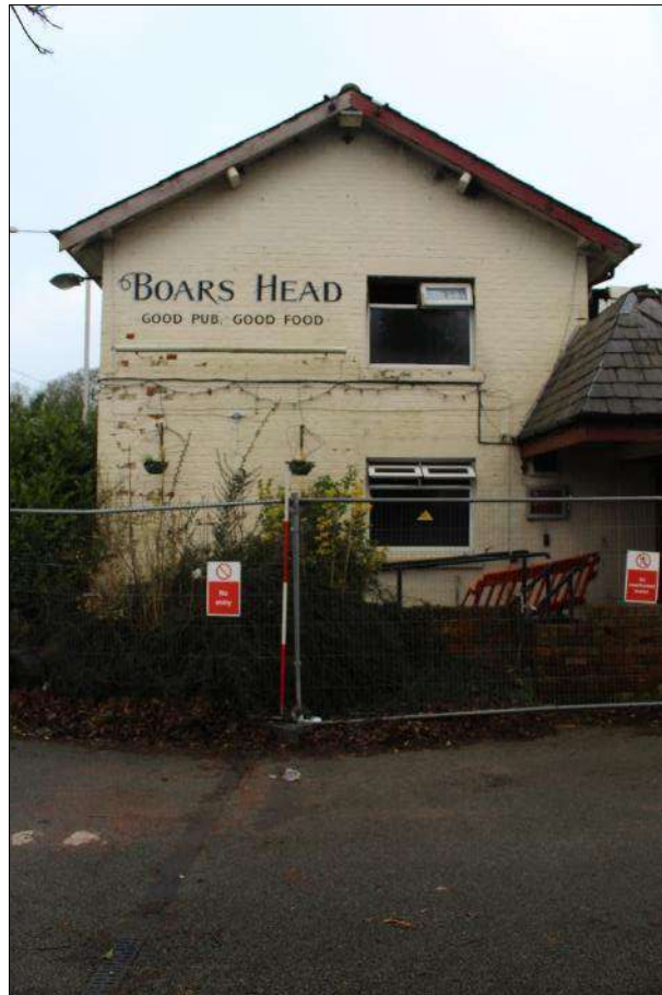
Plate 4 (shot 8): South elevation, looking north, 2m scale
