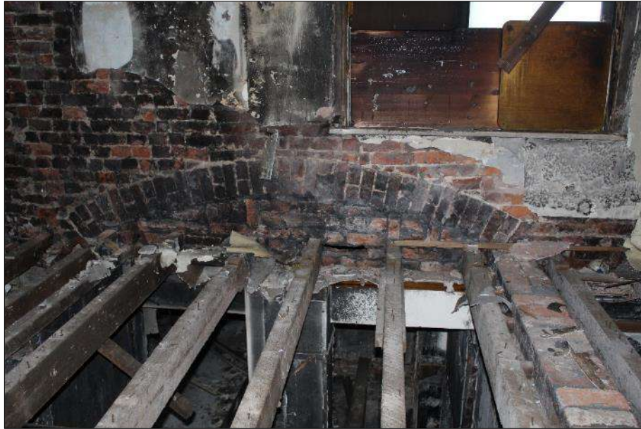
Plate 19 (shot 84): Segmental arch on the northeast wall. Looking east-northeast
