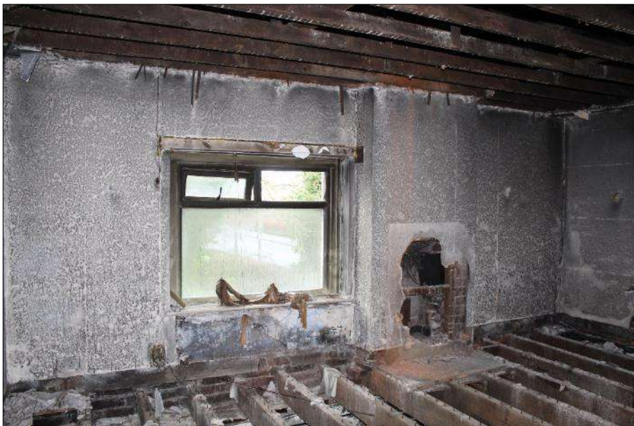
Plate 10 (shot 69): General view of southern room, looking southwest
