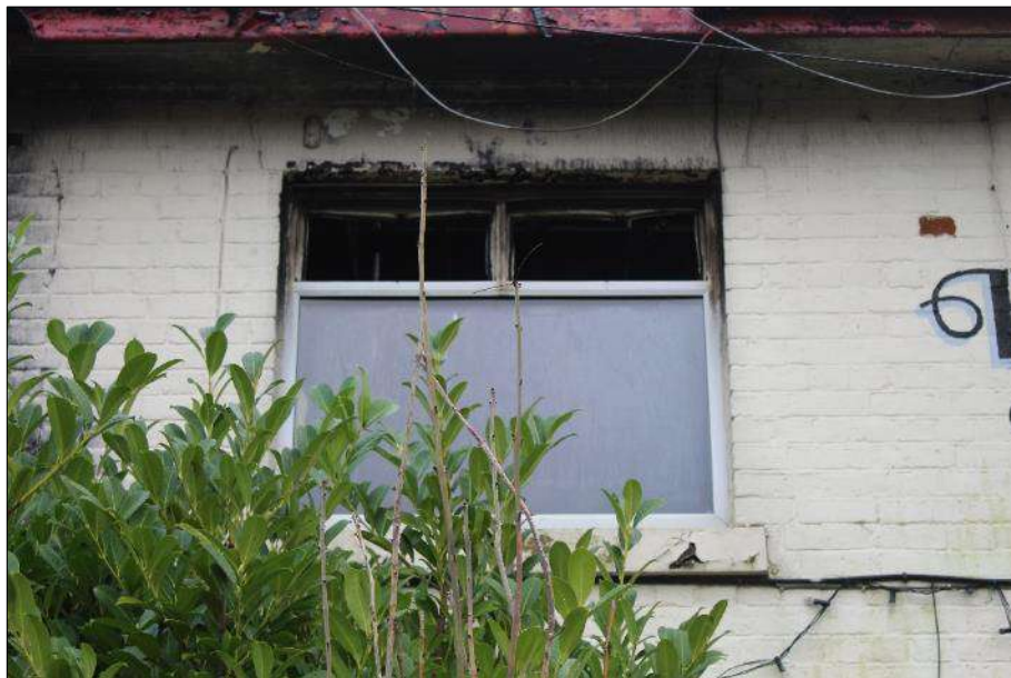
Plate 3 (shot 6): First floor window in front elevation, looking east
