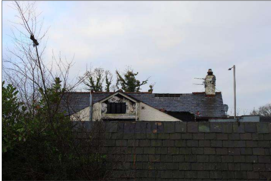
Plate 14 (shot 28): General view of gabled end of Structure B, looking west
