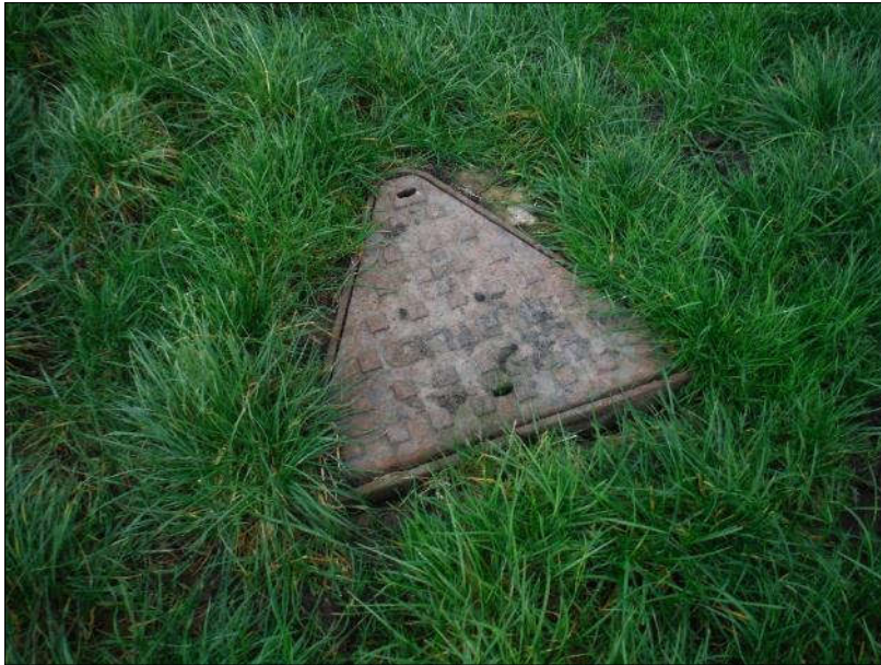
Plate 9: Triangular metal lid of a concrete inspection chamber within Field 6
