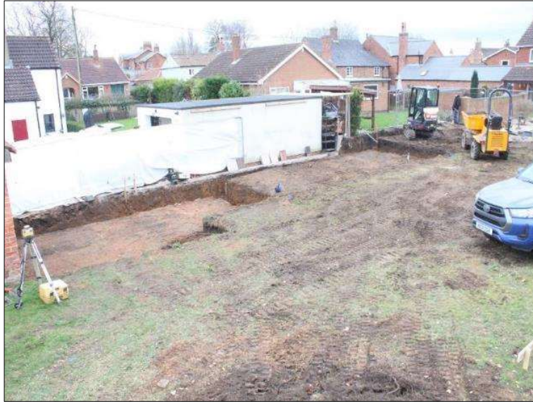
Plate 3: Extension foundations. Looking southwest. Scale 1m
