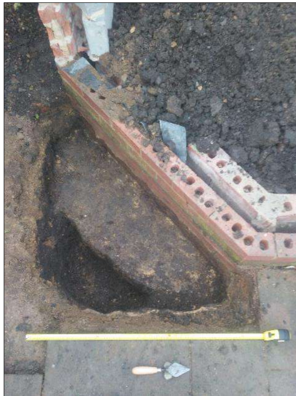
Plate 1: Hand excavated trench showing concrete wall foundation 004, looking west, scale 1m
