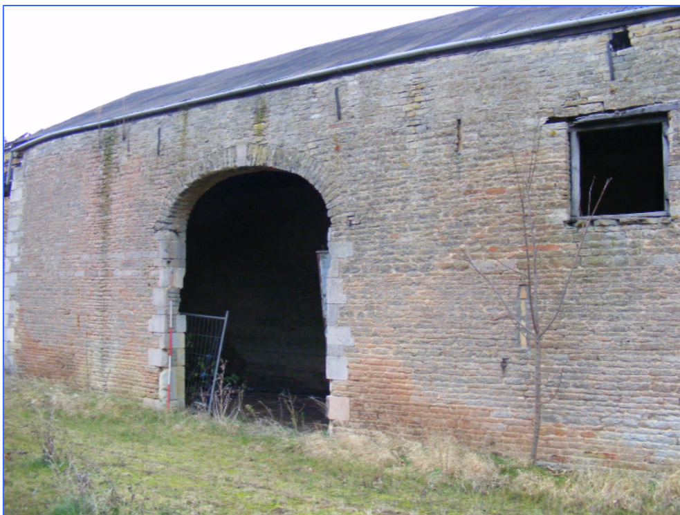
Plate 43 (Shot 65): West elevation of Building G, looking north-east, showing the large doorway typical of threshing barns.
