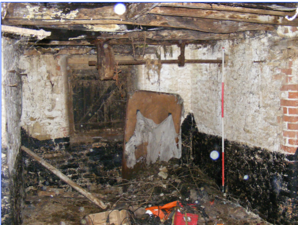
Plate 42 (Shot 69): Interior of Building F, ground floor, looking west.
