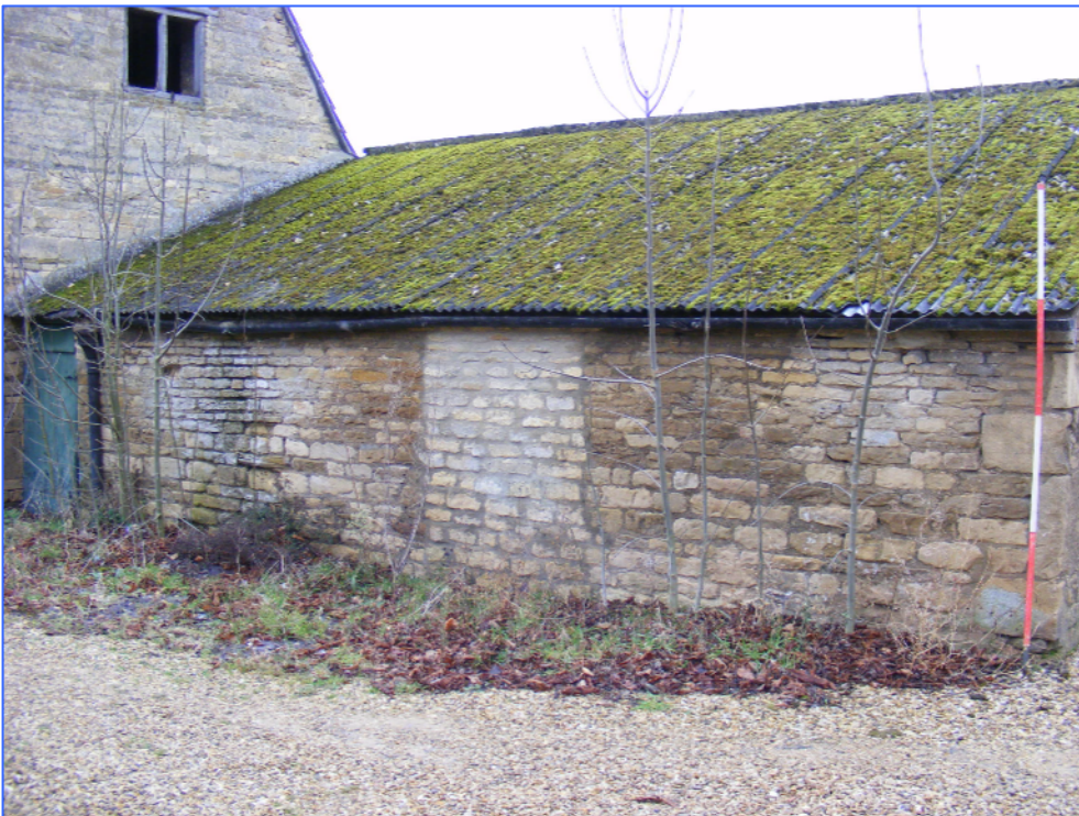
Plate 22 (Shot 37): South elevation of Building C, looking north-west.
