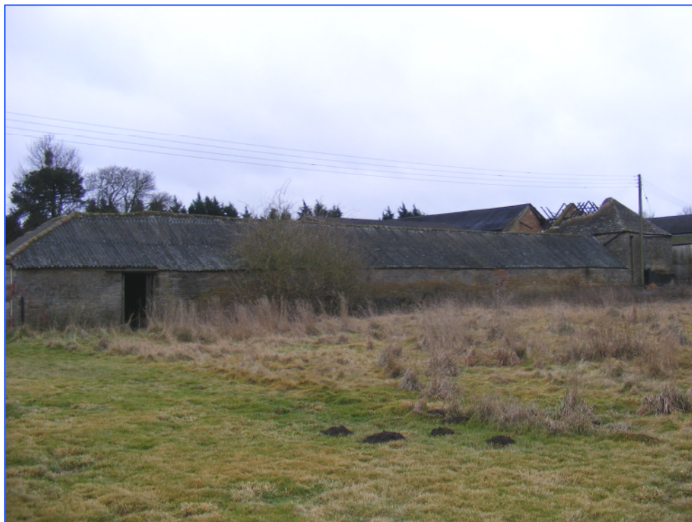
Plate 28 (Shot 4): North elevation of Buildings D (to left of shot) and E, looking west-north-west.
