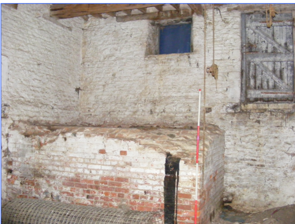
Plate 12 (Shot 73): Brick plinth, possible former machine stand at south end of Building A barn, looking south-south-east. Note also the doorway and pitching hole in the wall to the rear.
