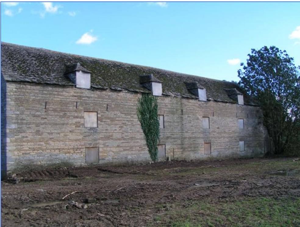
Plate 8 (Shot 119): West elevation of Building A barn, looking east-south-east.
