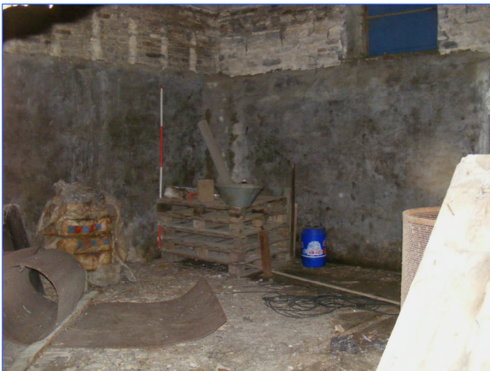
Plate 4 (Shot 86): Interior of the oast house, looking north. Note the scars defining the former joists of the first floor to the left of shot.
