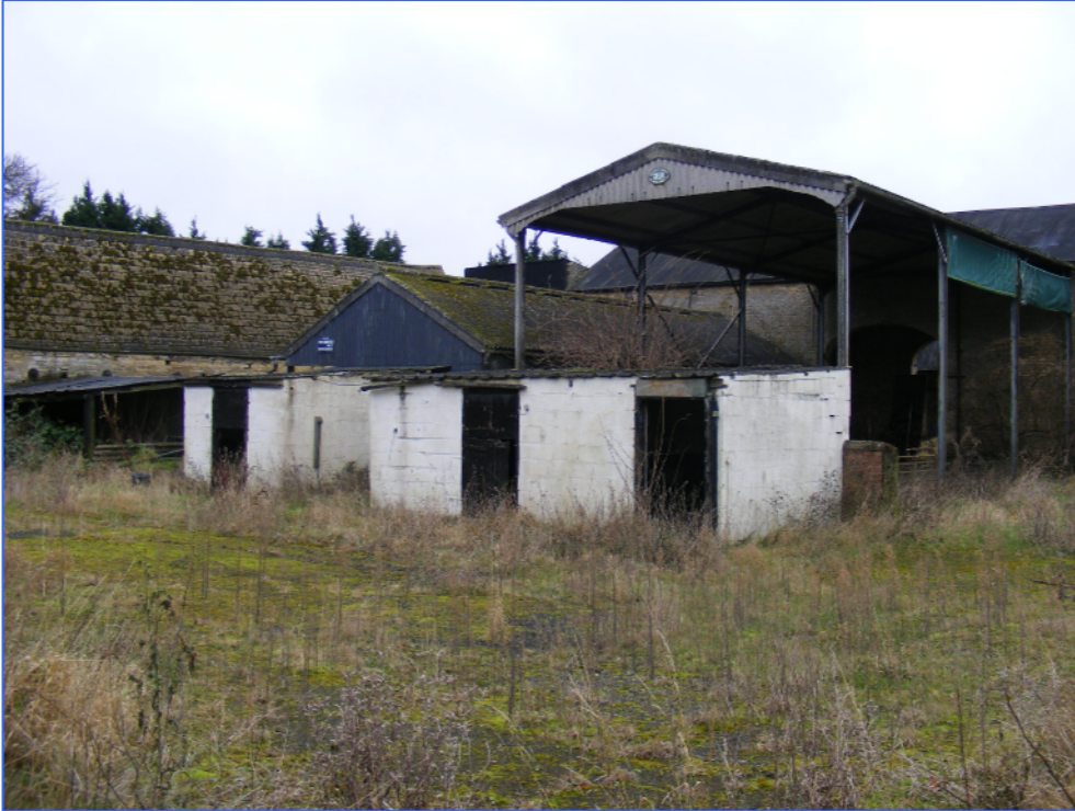
Plate 49 (Shot 18): Modern steel framed barns I and J, with modern breeze block outbuildings to their front. Looking south-west.
