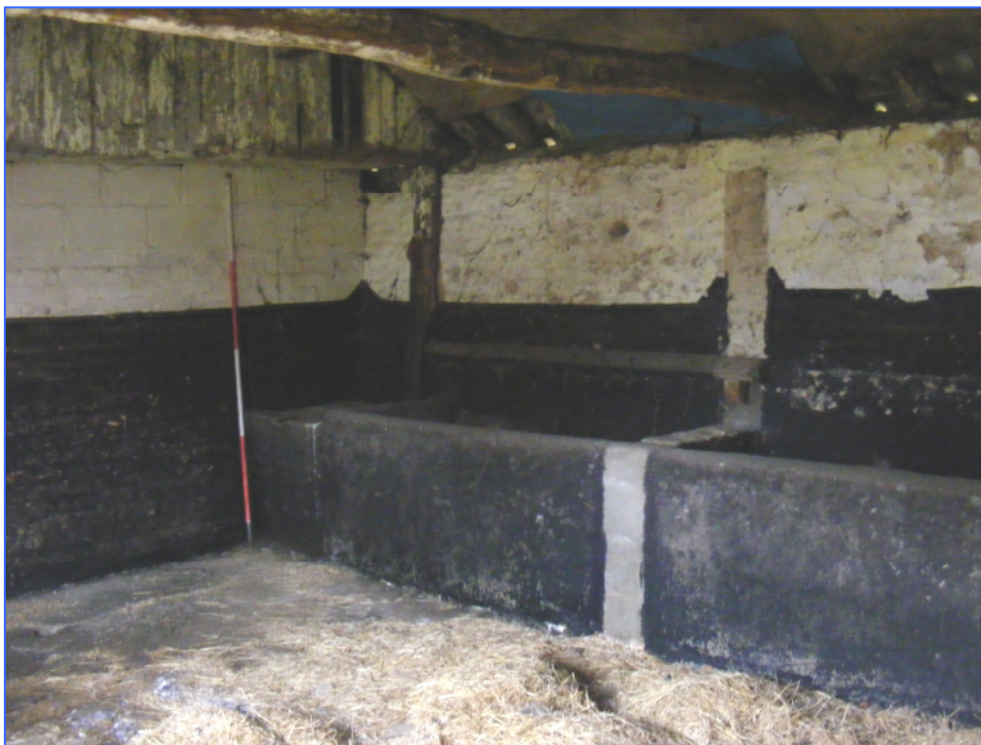
Plate 37 (Shot 25): Room E5, looking north-west. Note the scar in the middle of the shot indicating a probable former partition.
