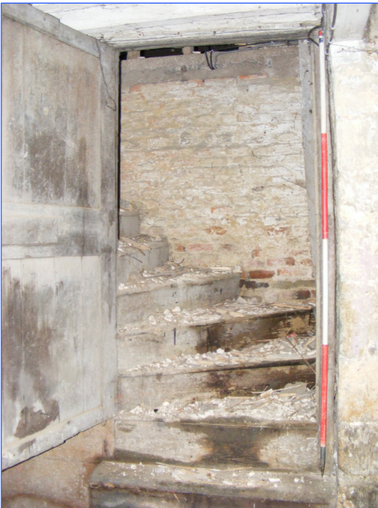
Plate 20 (Shot 47): Staircase in Building B, looking east.
