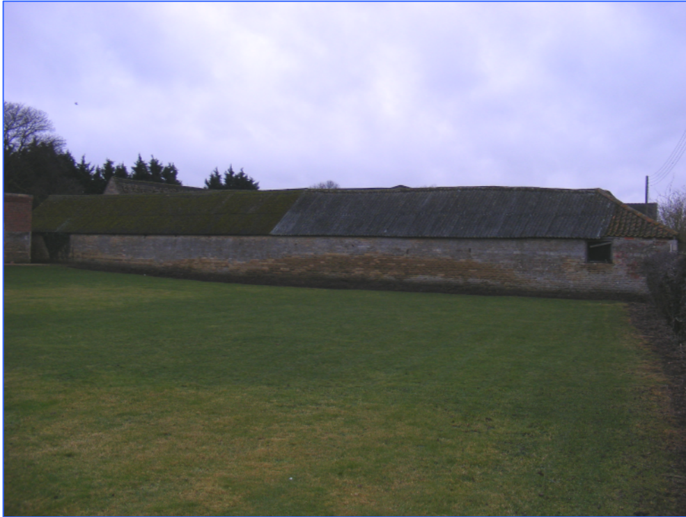
Plate 27 (Shot 3): East elevation of Building D, looking south-west.
