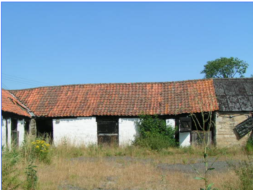
Plate 30 (Shot 155): West elevation of Building D, north end, looking east-north-east.
