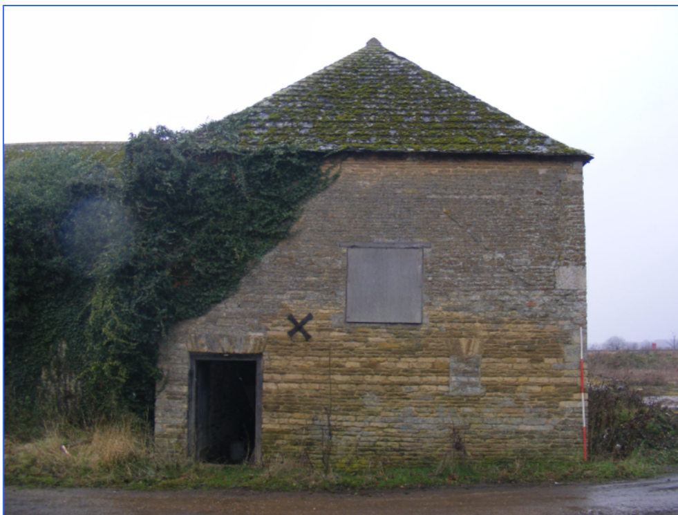
Plate 3 (Shot 90): East elevation of oast house, looking west-south-west. Note the faint roof scar on the north side of this elevation.
