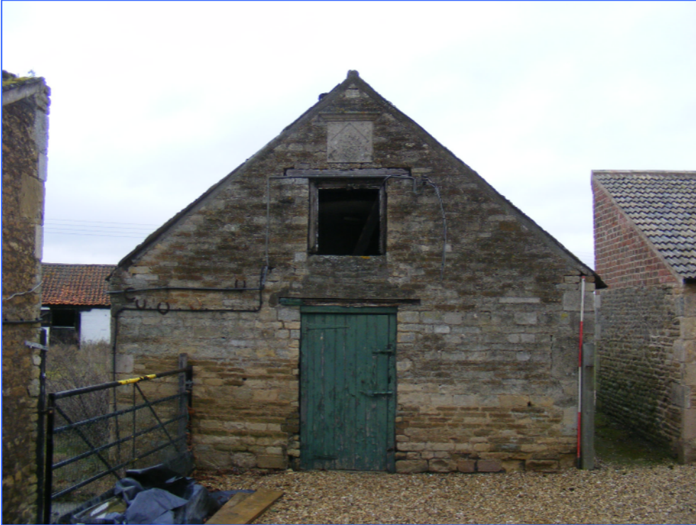
Plate 25 (Shot 1): South elevation of Building D, looking north.
