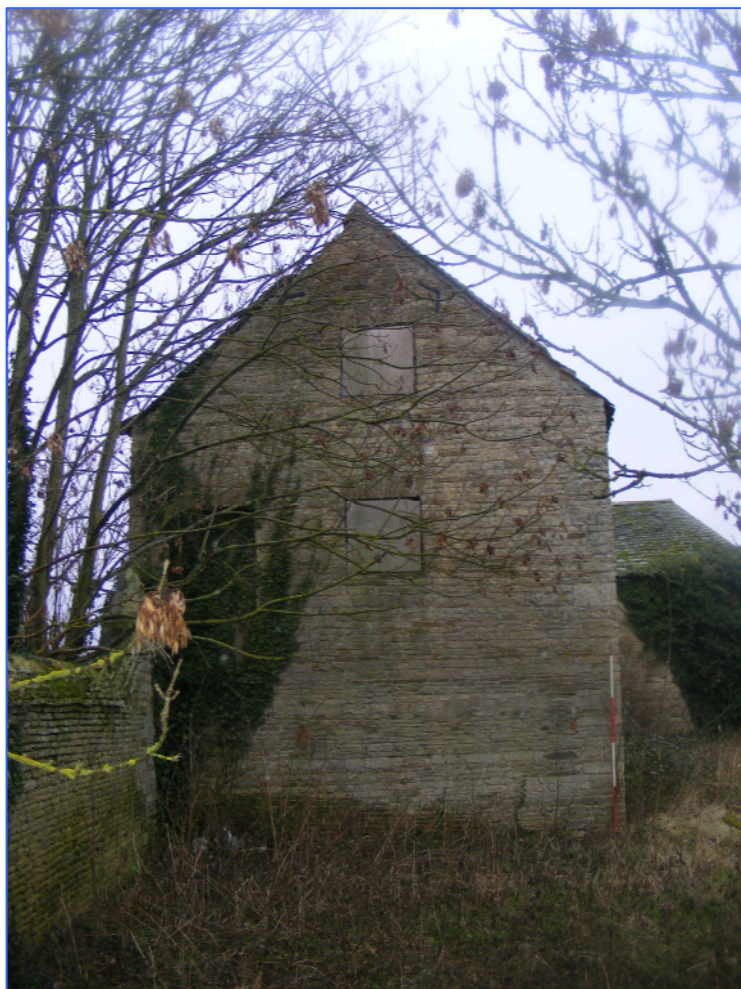
Plate 10 (Shot 89): South elevation of Building A barn looking north-north-west.
