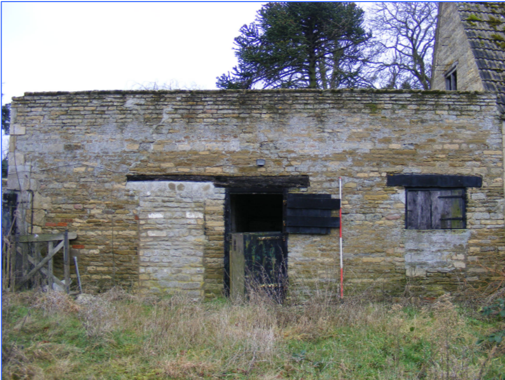
Plate 23 (Shot 38): North elevation of Building C, looking south.
