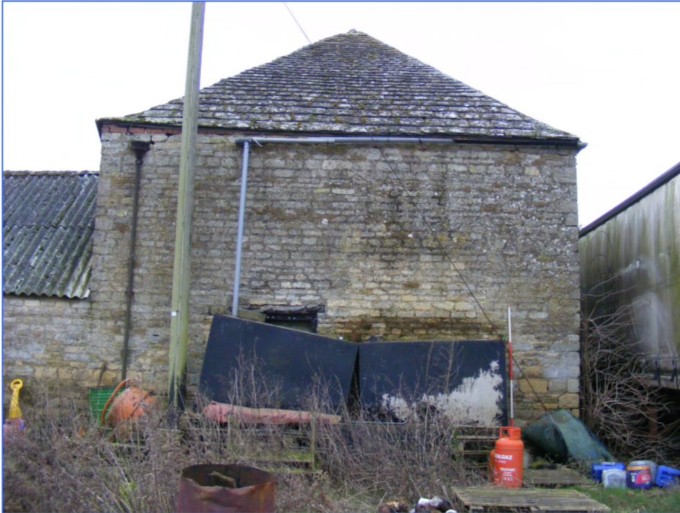
Plate 41 (Shot 66): North elevation of Building F, looking south-south-east.
