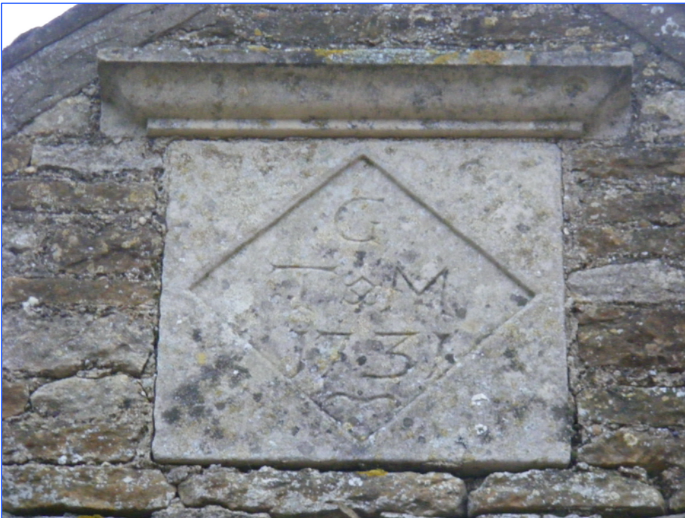
Plate 26 (Shot 2): Detail of datestone in south elevation of Building D, looking north.
