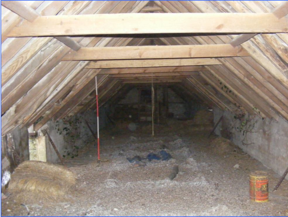
Plate 13 (Shot 47): First floor of Building A barn, looking south-south-east.
