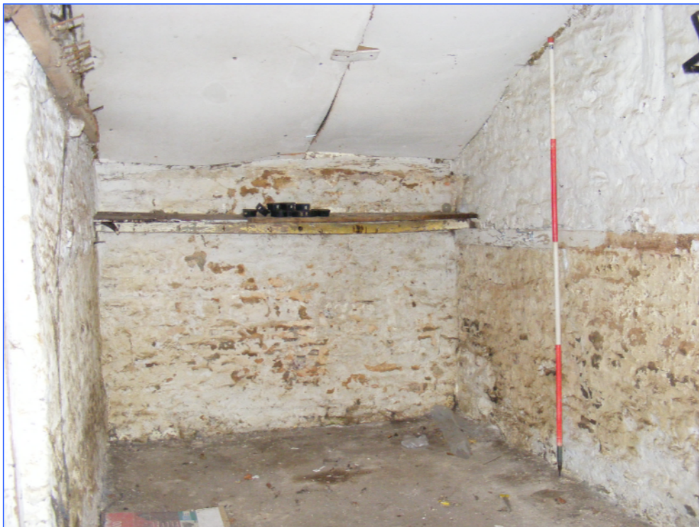
Plate 24: (Shot 39): Central room (C2), in Building C, looking south-south-east.
