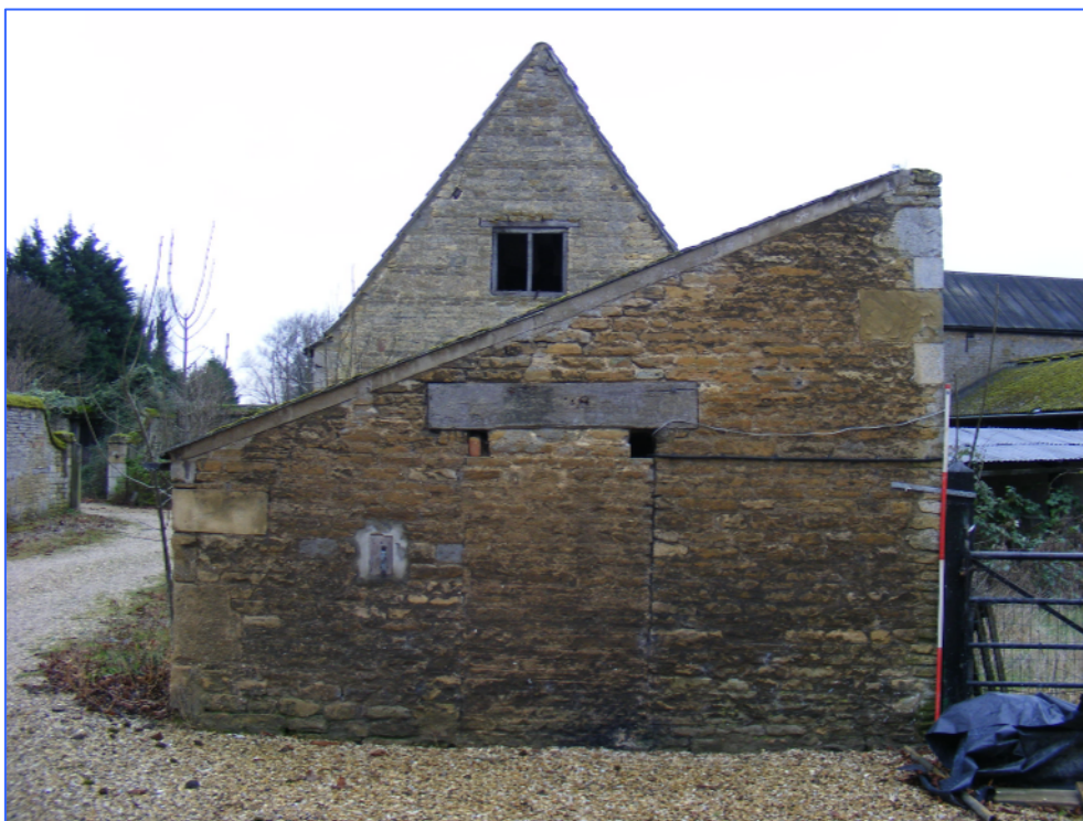
Plate 17 (Shot 36): East elevations of Buildings C (foreground) and B (background), looking west.
