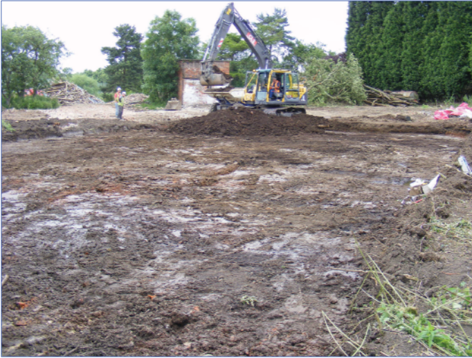
Plate 1: The house footprint after machine stripping, looking north.
