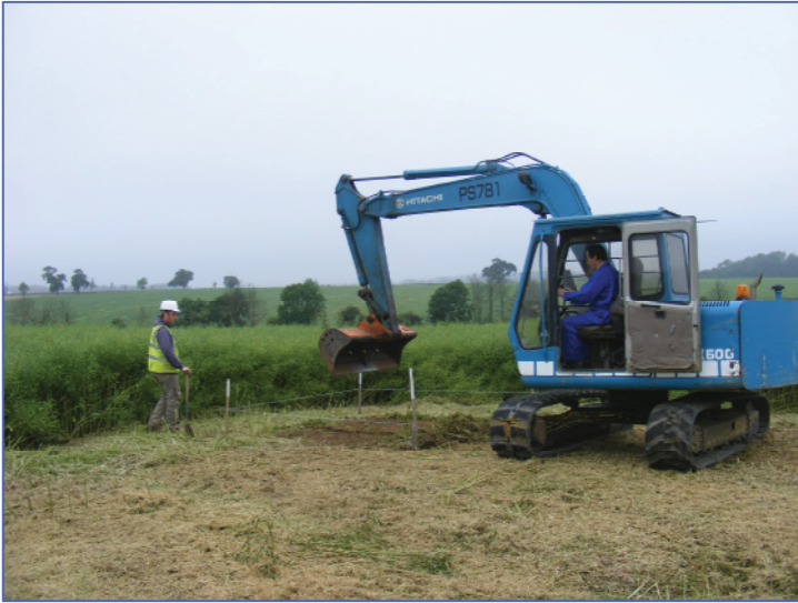
Plate 1: General view of the proposed development area during machining, looking north-west
