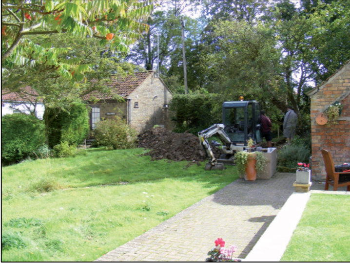
Plate 1: General view of the site, looking east-south-east
