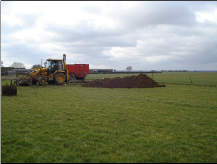
Plate 1: General view of the excavation area, looking south-west
