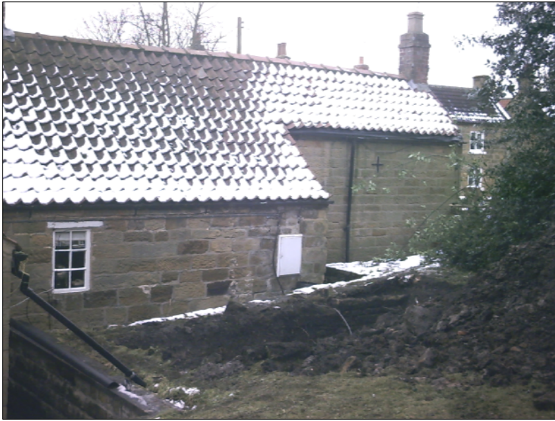
Plate 1: Overall shot of site during groundworks, looking south-west
