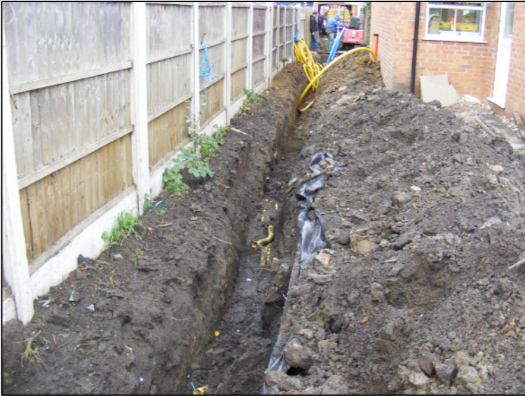
Plate 1: Working shot looking north along service trench towards St. Catherine's Grove
