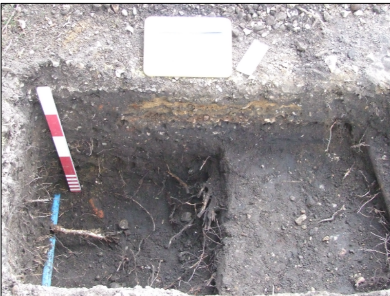
Plate 3: North-west facing section in Test Pit 3 showing water service [303] to the left and disused gas service [306] to the right, looking south-east
