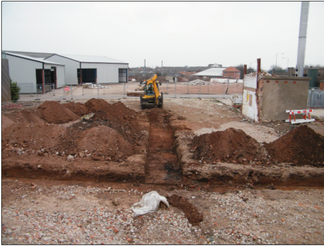
Plate 1: General view of the site during excavation, looking north
