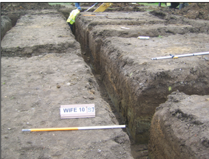
Plate 3: Detail of foundations in central part of the site, looking east
