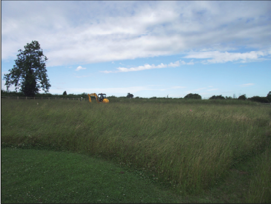
Plate 1: General shot of excavation area taken from northern corner of landscaped area, looking north-west
