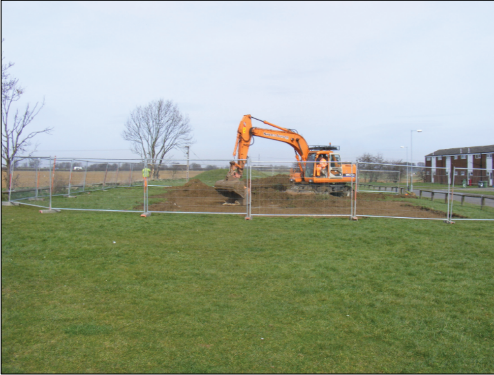
Plate 1: General site shot, looking north during groundworks
