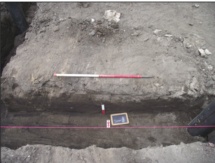
Plate 3: Representative section of ring beam foundation. Looking south
