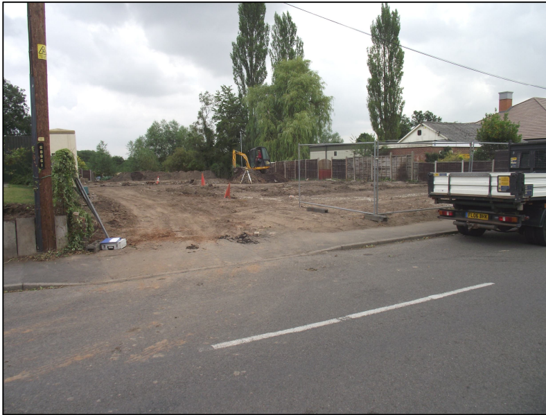
Plate 1: General view of site looking east-north-east from Main Street
