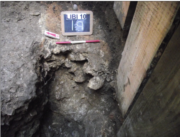
Plate 5: Close up of wall foundation cut [221] in Test Pit 2, looking east
