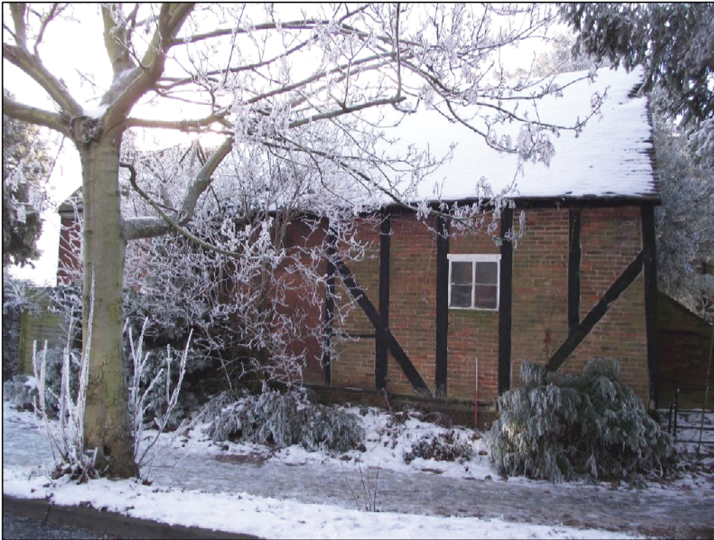
Plate 5 (Shot 4): North elevation showing later added window. Looking south
