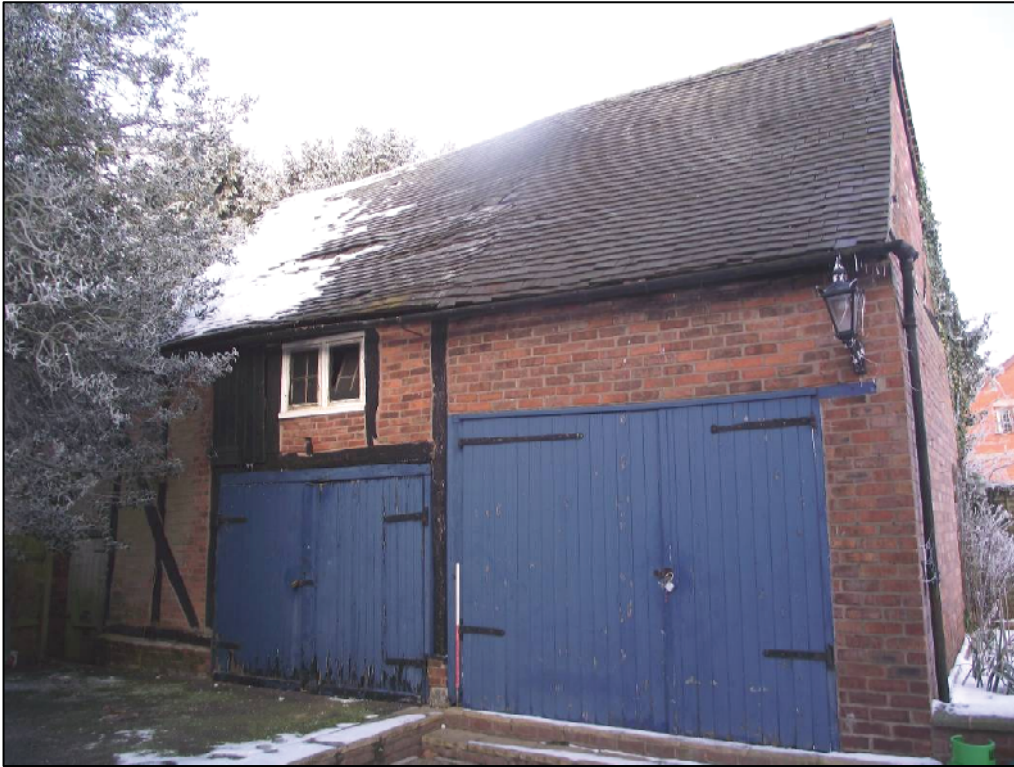
Plate 1 (Shot 1): South elevation of building, looking north-west. Note two phase construction, with earlier part to the left
