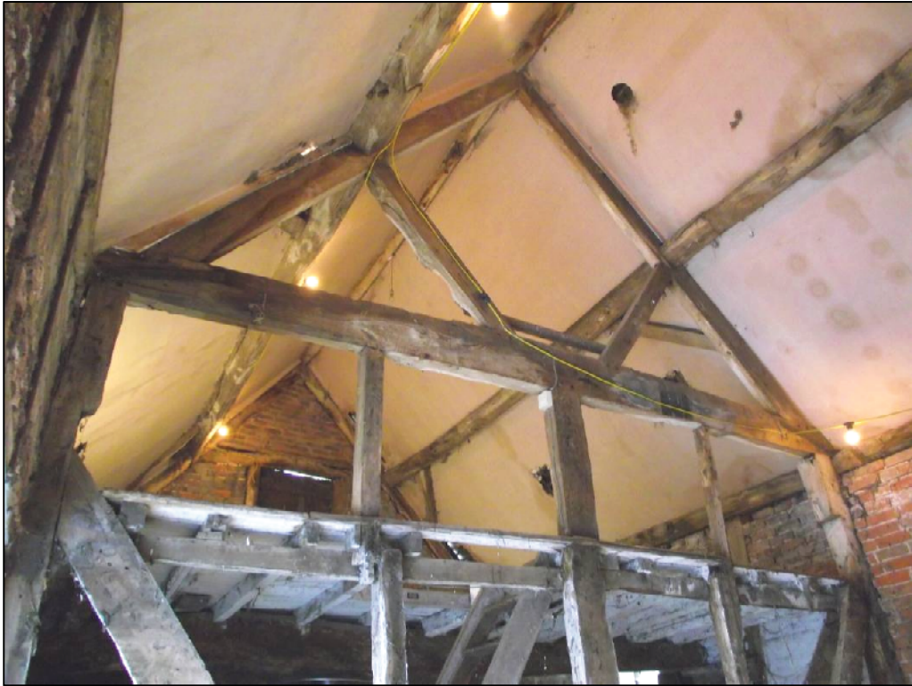
Plate 9 (Shot 19): Tie beam roof truss and hayloft, looking west-north-west
