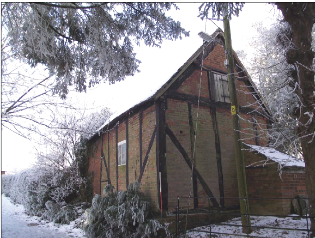
Plate 2 (Shot 5): North-west corner of the coach house showing timber framed construction of north and west elevations. Looking east-south-east
