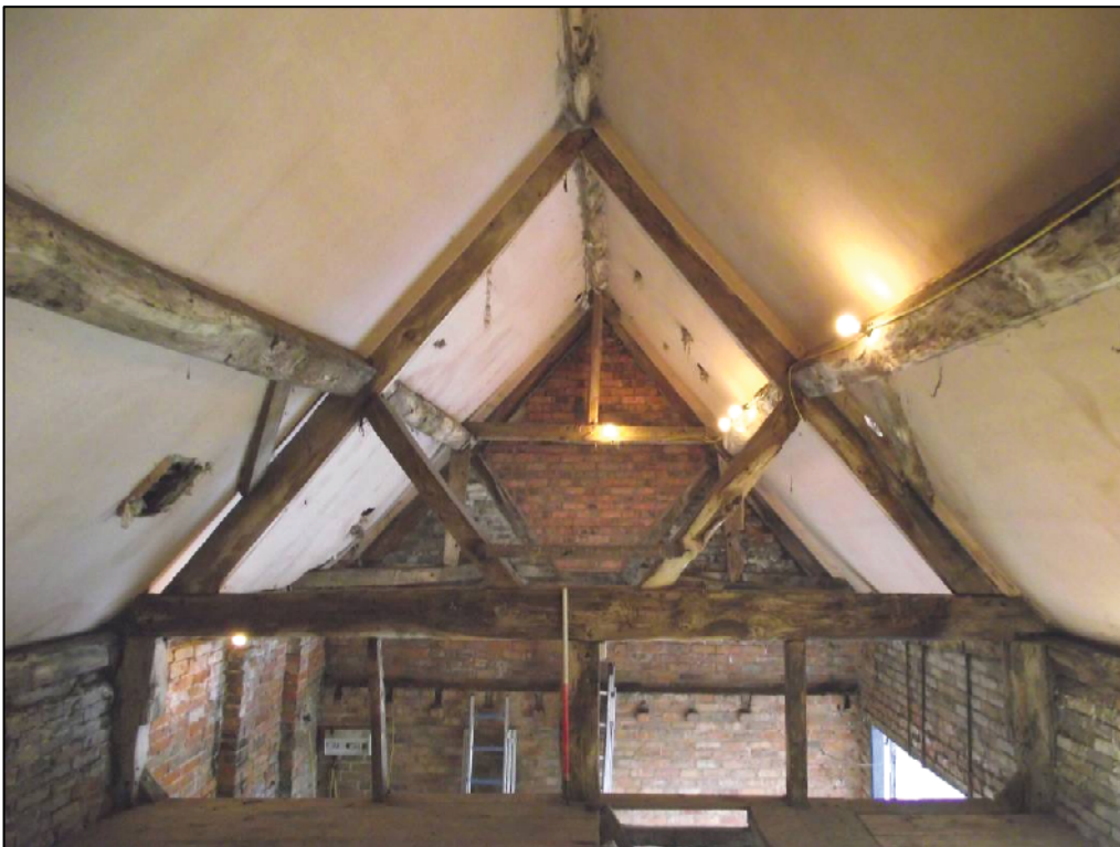
Plate 8 (Shot 17): Interior roof shot of roof trusses, looking east
