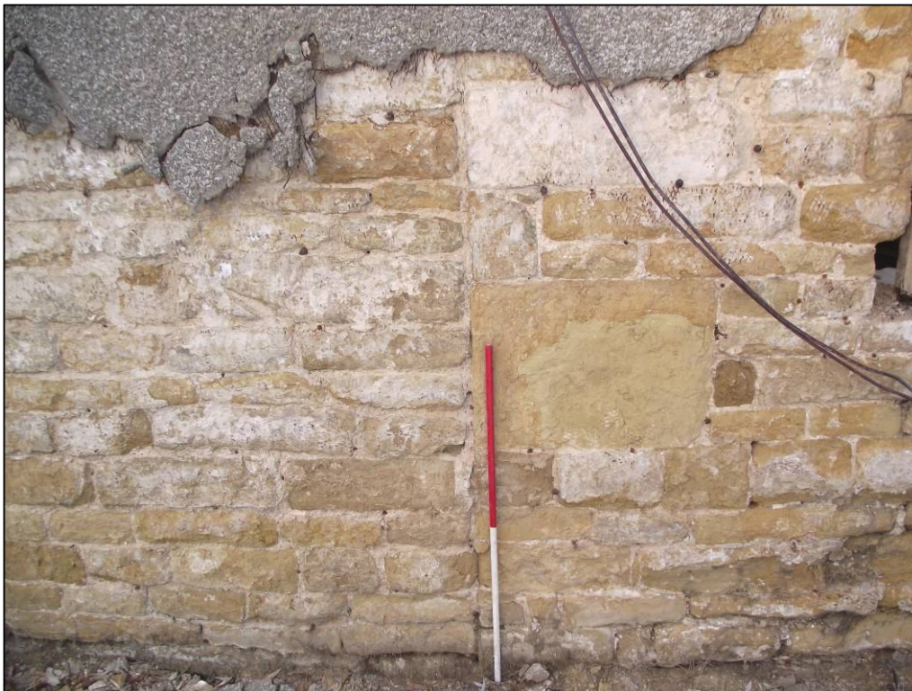
Plate 3 (Shot 14): Detail of east elevation showing joint between two early building phases of the chapel. Notice the large quoins to the right representing the corner of the early chapel
