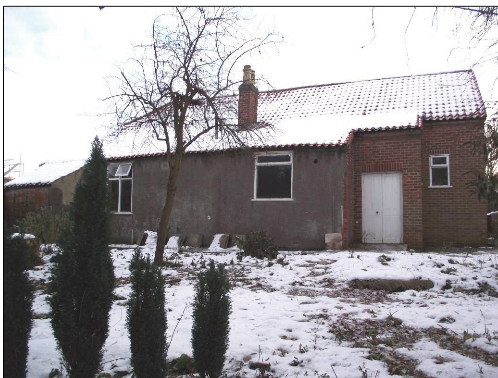
Plate 6 (Shot 8): West elevation of chapel, looking east-north-east
