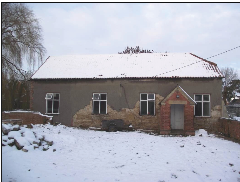
Plate 2 (Shot 1): East elevation of the chapel, looking east
