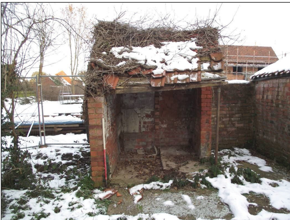
Plate 8 (Shot 11): Derelict brick outbuilding adjacent to the coal store. Looking north
