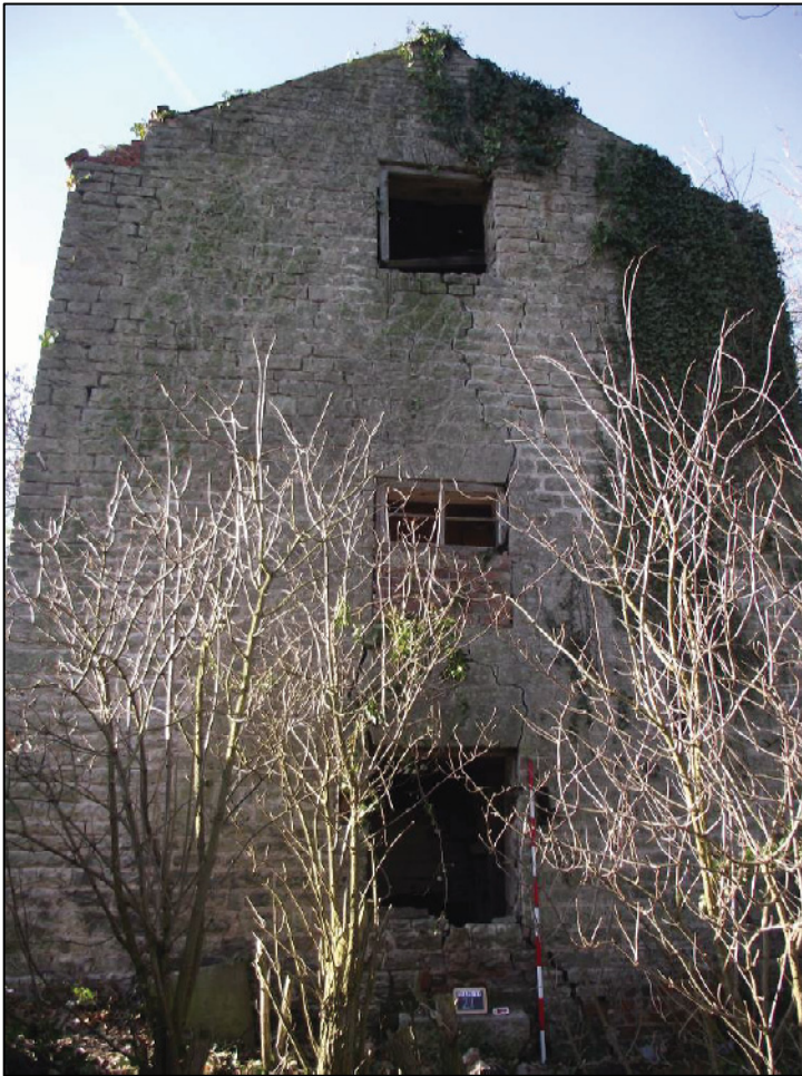
Plate 13 (Shot 21): East elevation, looking west-north-west
