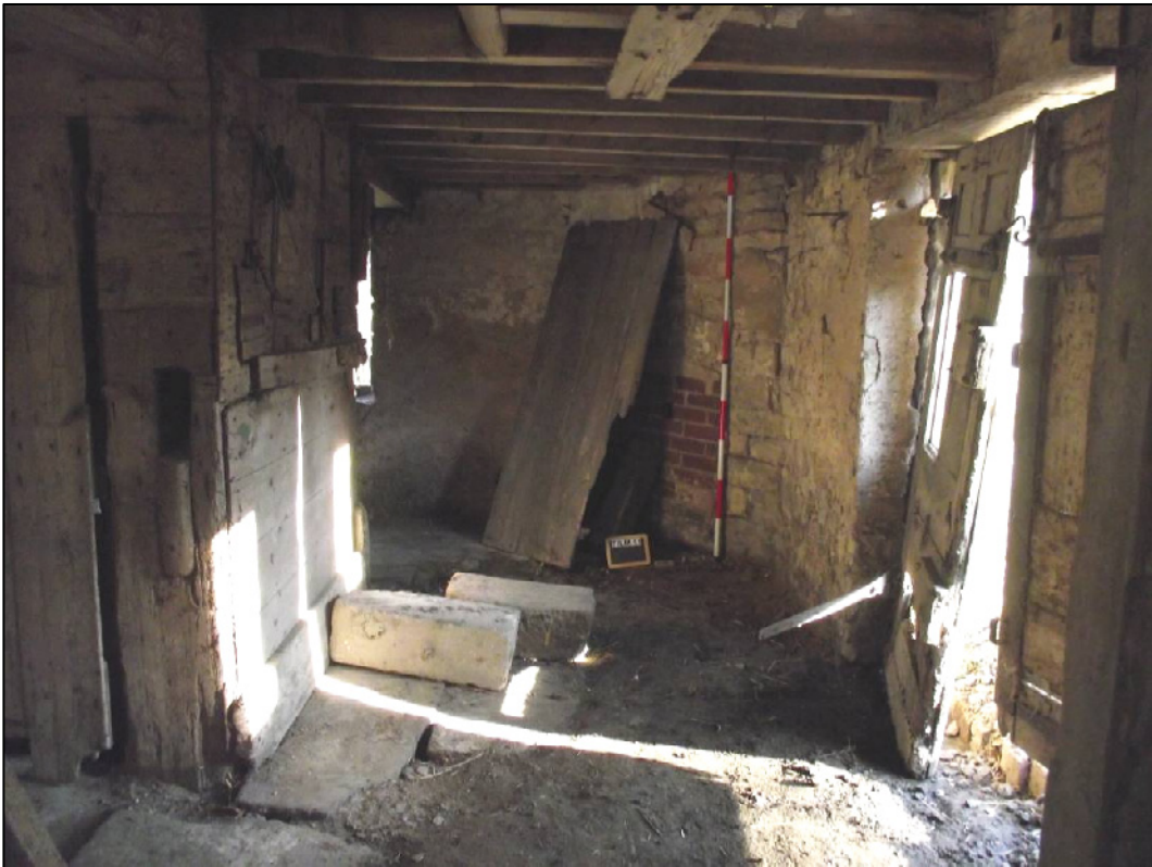
Plate 15 (Shot 30): General shot of south and east elevation showing a brick repair in the south-east corner and the south partition wall of the cog house to the left. Looking east. A flour sack would have hung from the hooks on the cog-house wall and was filled by a chute inside the cog-house (Plate 23)
