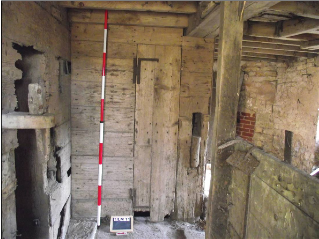
Plate 19 (Shot 38): Door of the cog-house with graffiti (see Plate 20). Looking east
