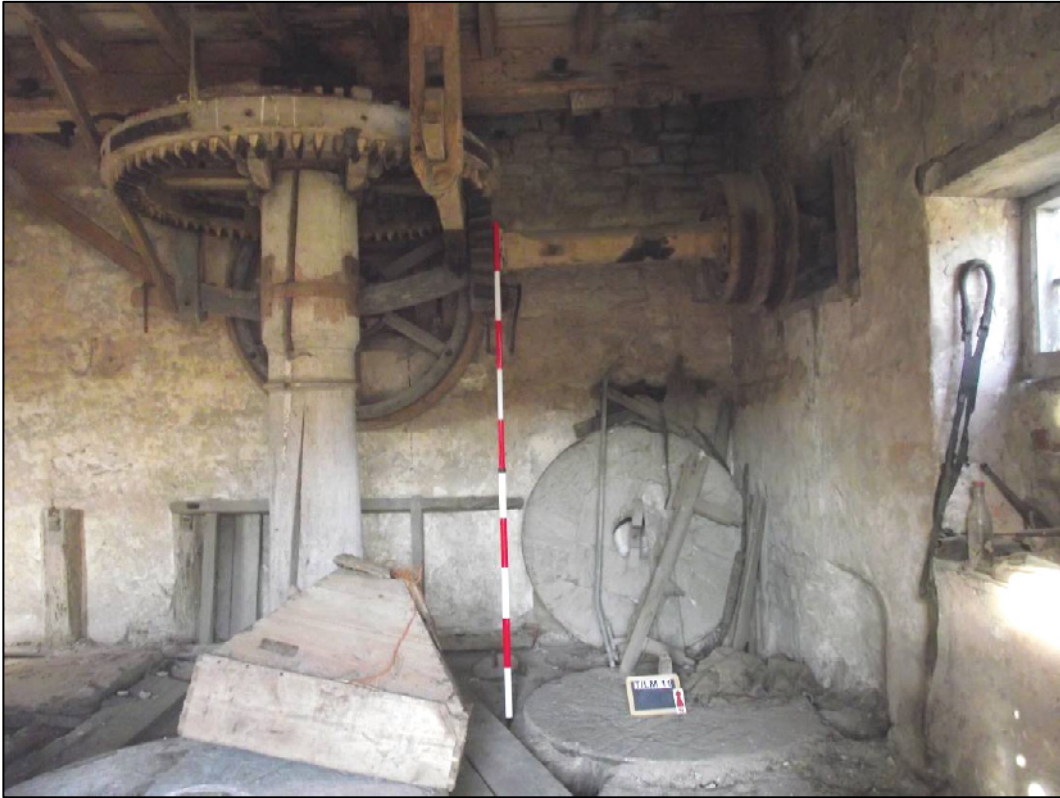
Plate 27 (Shot 55): General shot of machinery on first floor. The millstone runner in the corner would probably have been fitted on the bedstone in front of it. Looking north
