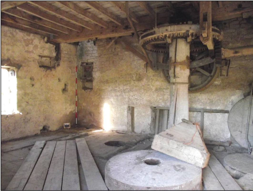
Plate 25 (Shot 52): General view of first floor, showing, main shaft, crown wheel and millstones turned by the spindles below. Note missing millstone to west of shaft. Looking north-west
