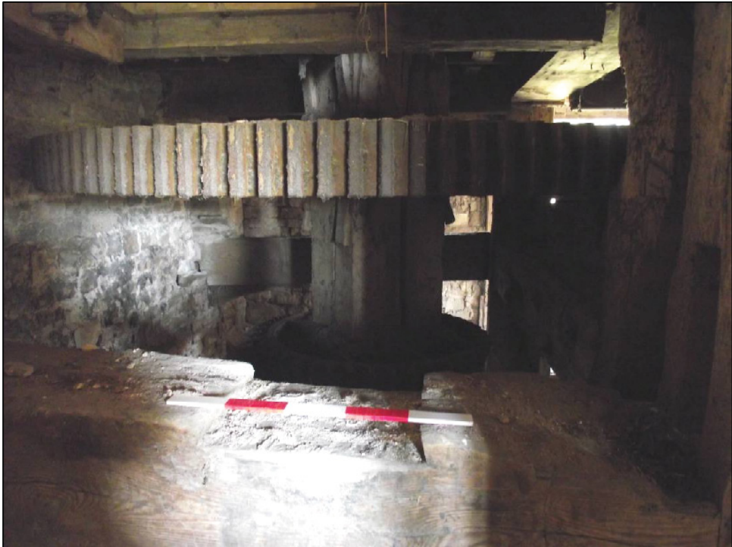
Plate 22 (Shot 46): The great spur wheel, which makes the stone nut turn above (see Plates 23 and 24). A former stone nut that fitted in to the slot in the wooden beam in the foreground is presently located on the floor west of the cog-house (see Plate 17). Looking east
