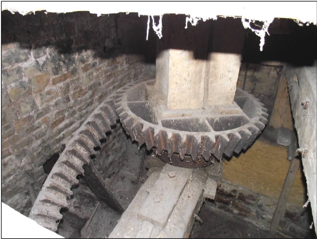
Plate 21 (Shot 37): General shot into the base of the cog-house showing the pit wheel connected to the waterwheel on the outside via the shaft, making the horizontal wallower/primary crown turn the main shaft, connected to the great spur wheel above shown on Plate 22. Looking north-north-east
