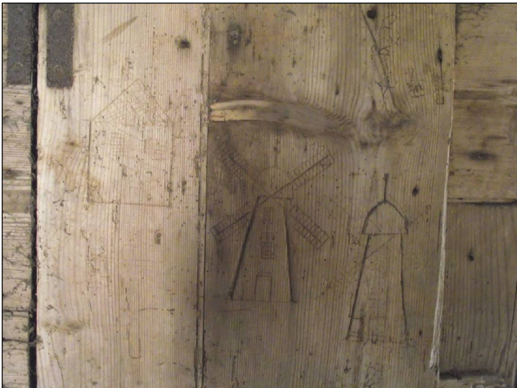
Plate 20 (Shot 39): Detail of group of graffiti on door of the cog-house. Looking east
