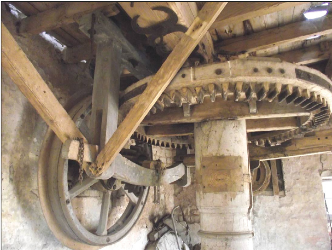
Plate 28 (Shot 54): Detail of machinery showing main shaft and crown wheel and belt driven secondary machinery to the left. Looking east-north-east
