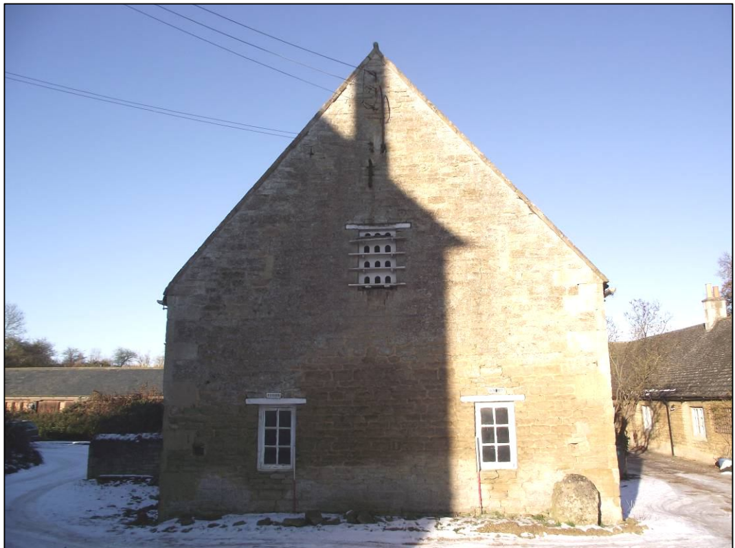
Plate 4 (Shot 5): South-east elevation showing nesting holes on the gable, looking north-west
