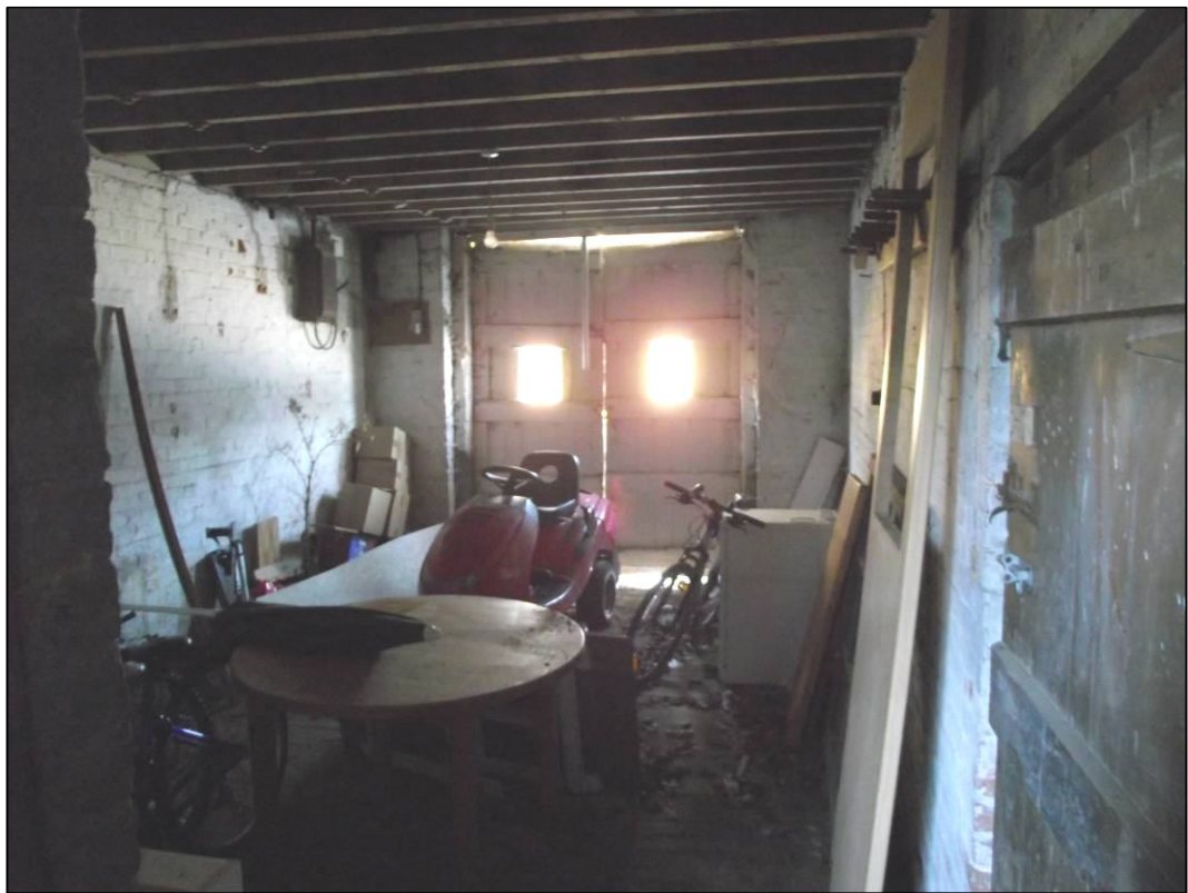
Plate 11 (Shot 14): General shot of garage/store interior, looking north-east
