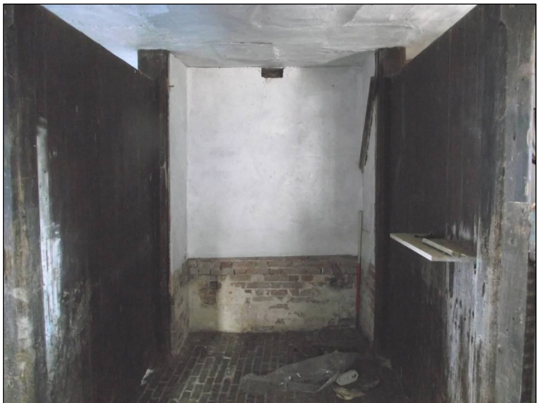
Plate 8 (Shot 11): Close-up of stable with hatch in the ceiling, looking south-west. The wooden partitions about the brick roof supports visible on the first floor (see Plate 16)
