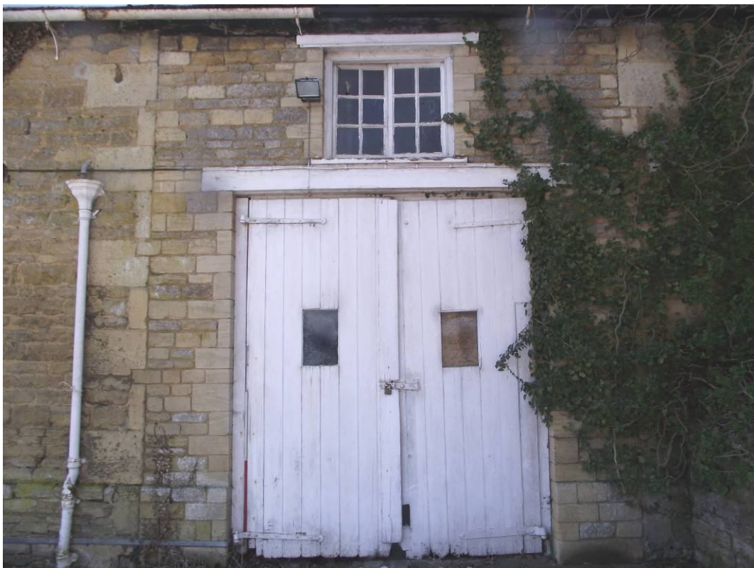
Plate 6 (Shot 9): Detail of quoins on the early stable block and wooden double doors and first floor window on the later extension. Also notice the quoins on the right hand side of the shot, suggesting a space may have only been blocked up rather than it being an added extension, looking south-west
