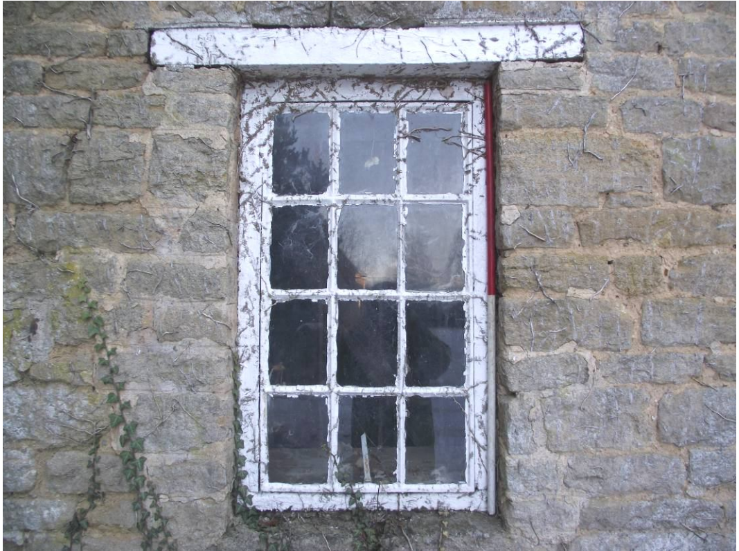
Plate 3 (Shot 4): Detail of window on south-west elevation, looking north-east
