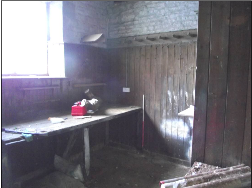
Plate 13 (Shot 16): General shot of tack room, looking north-west
