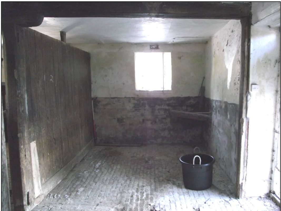
Plate 10 (Shot 13): Close-up of south stall in stable block, looking south-east
