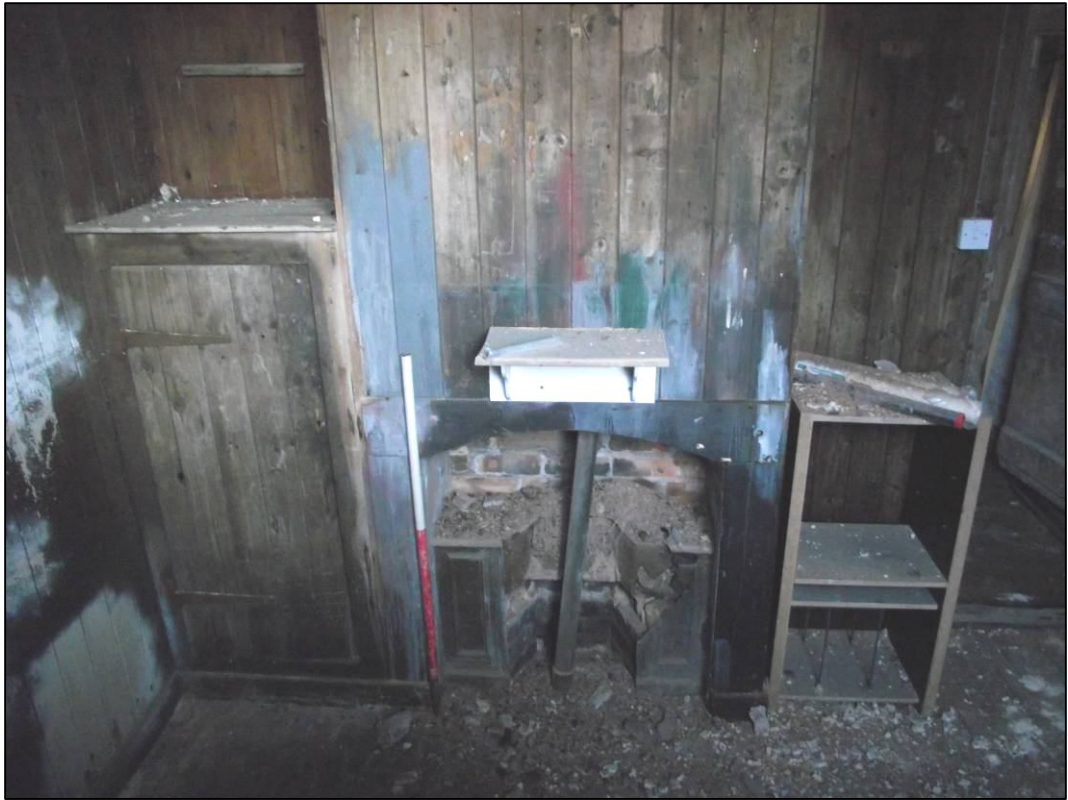
Plate 15 (Shot 17): Detail of fireplace in tack room, looking east-north-east
