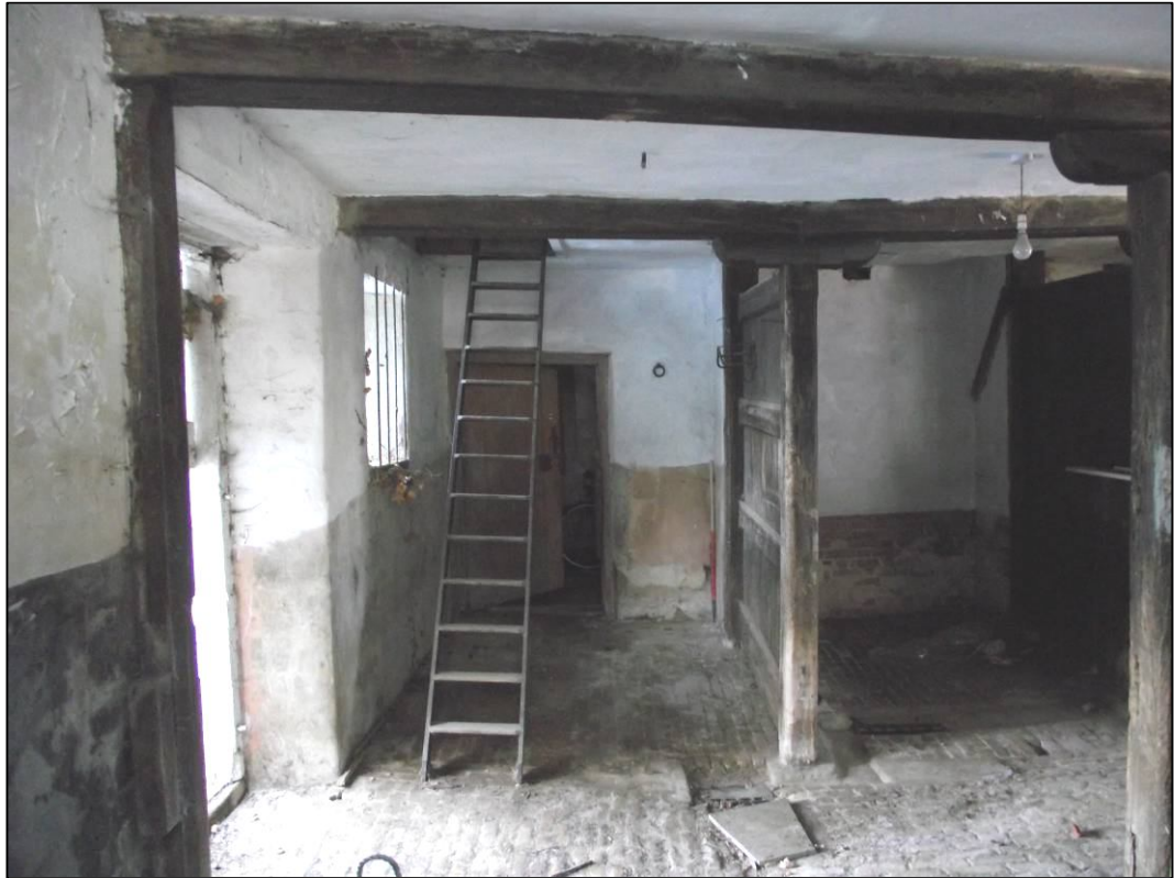
Plate 9 (Shot 12): General view of stable interior with hatch and ladder leading up to the hayloft. Notice the steel bars in front of the opening to the left of shot, there is also a metal fitting on the wooden partition wall for hanging a tack or harness, looking south-west
