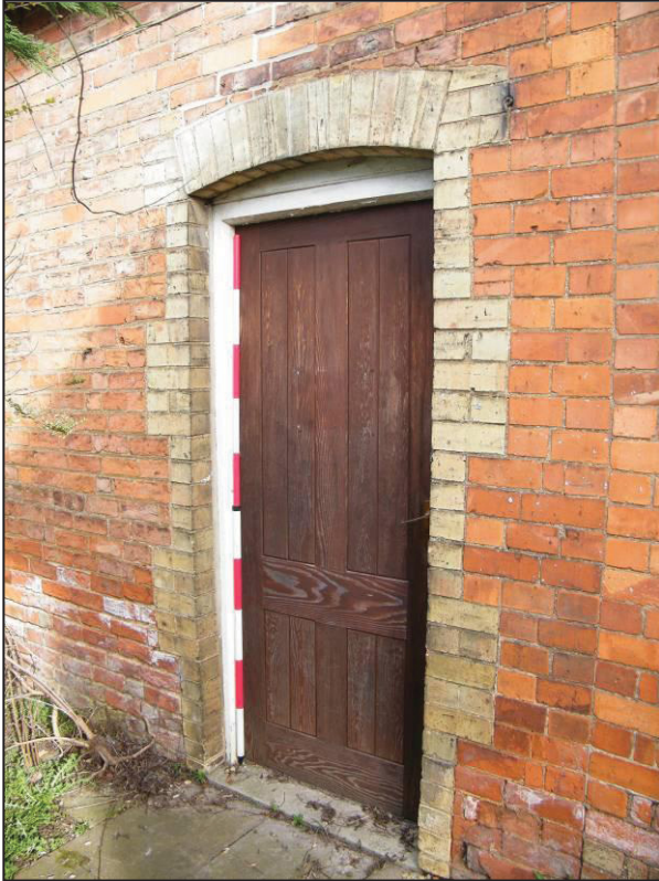
Plate 11 (Shot 21): Close-up of the door to the old schoolroom, showing yellow brick dressings. Note the join in the two phases of brickwork to the right of the door
