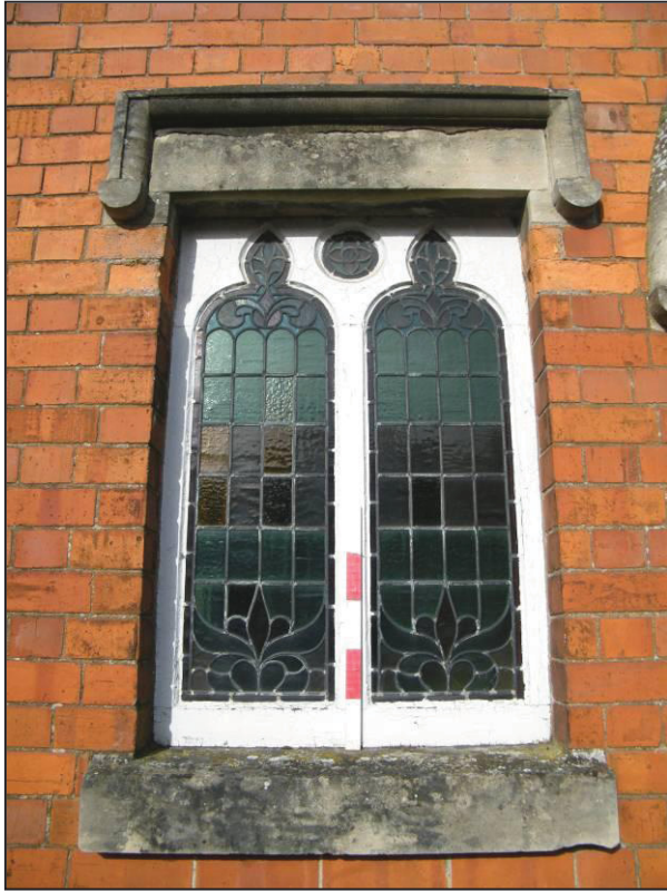
Plate 3 (Shot 2): Representative shot of one of two windows with a label mould, stone lintel and stone sill on the main entrance, looking west
