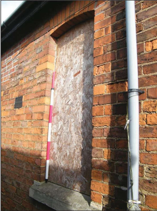
Plate 13 (Shot 23): Detail of window in old schoolroom, looking north-west
