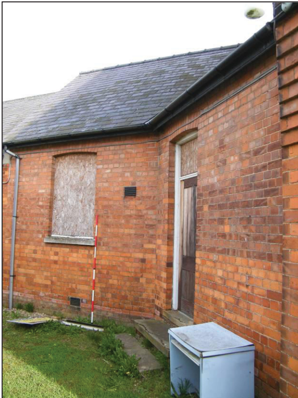
Plate 10 (Shot 18): South elevation of extension adjacent to the chapel, looking north-west
