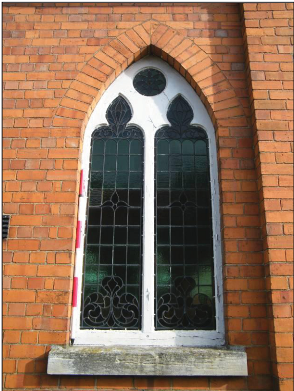
Plate 6 (Shot 16): Window in south elevation, looking north
