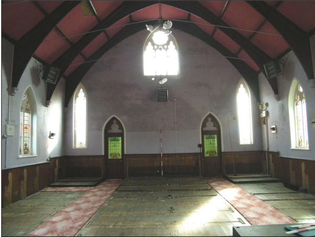
Plate 17 (Shot 28): View of chapel interior, looking east
