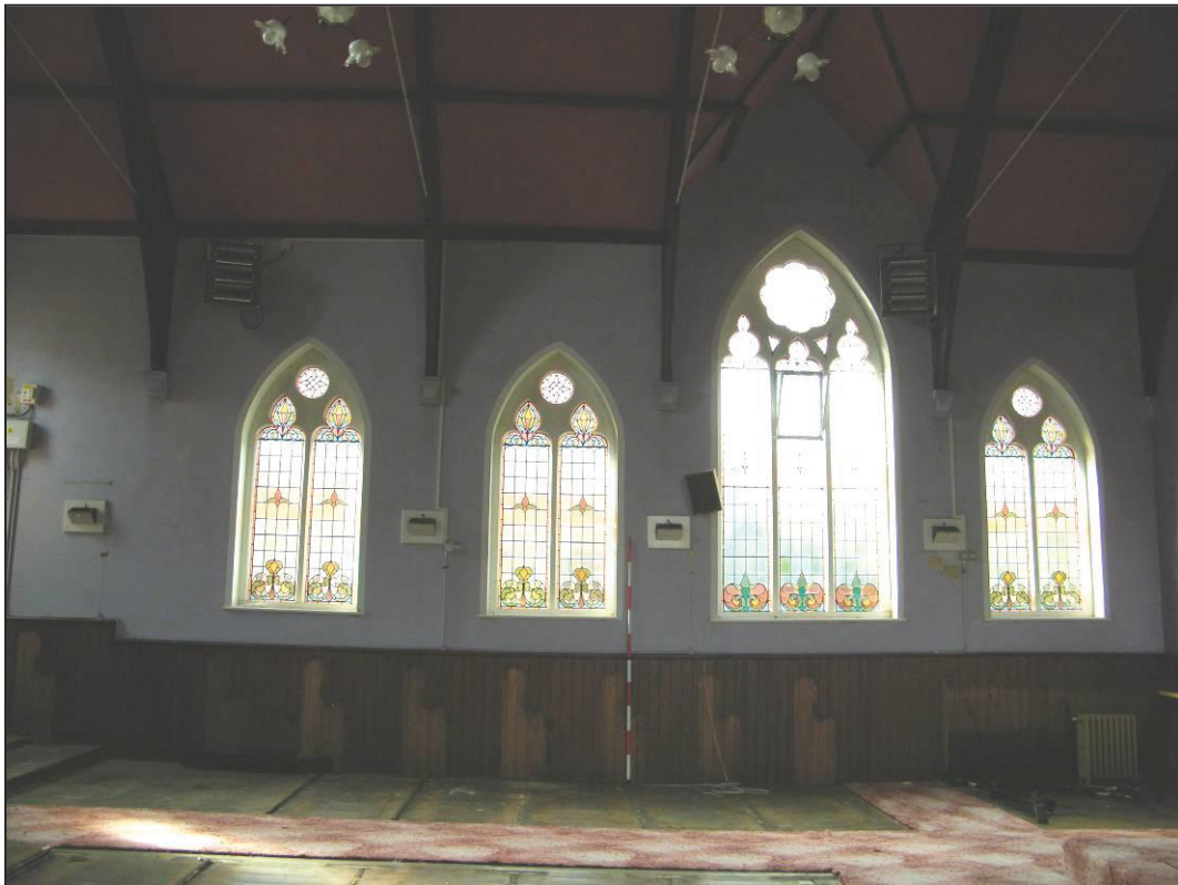
Plate 20 (Shot 31): South elevation of the chapel, looking south
