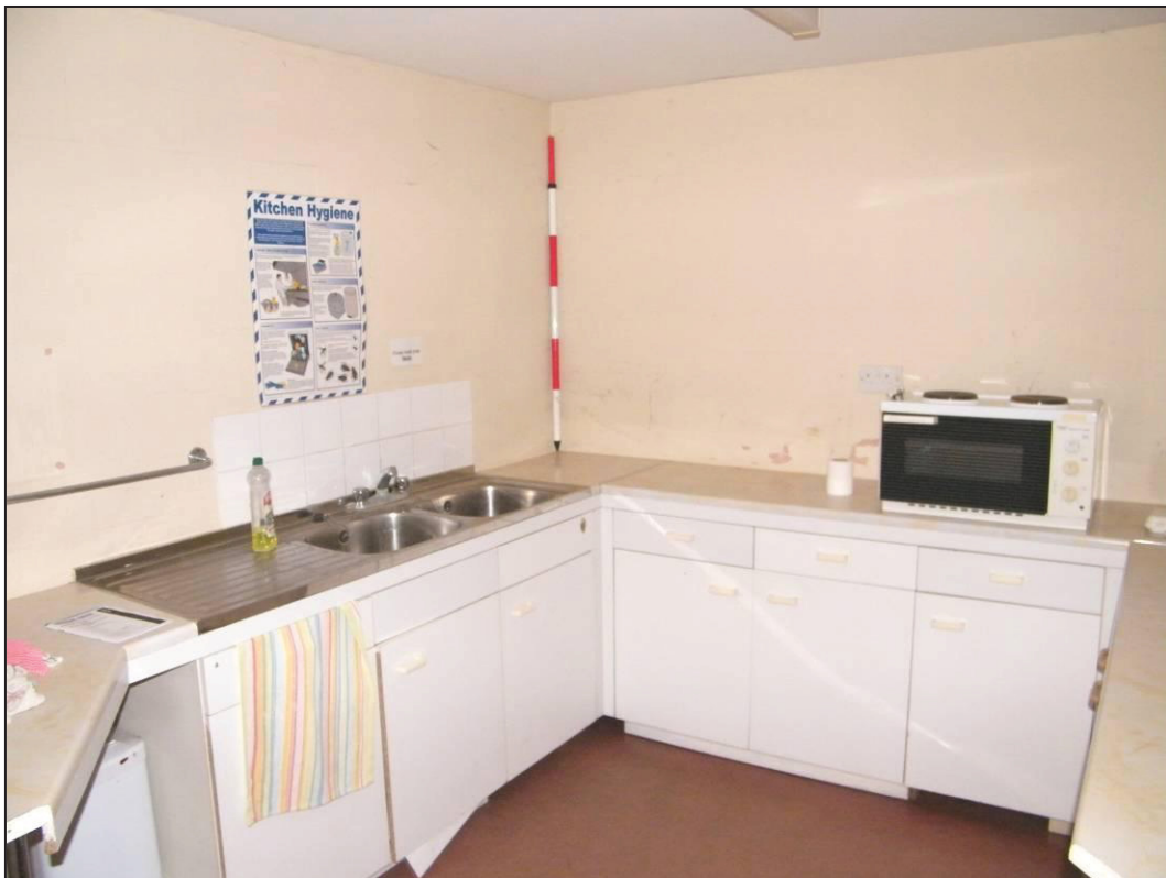
Plate 30 (Shot 42): Kitchen area in westernmost block, looking south-east
