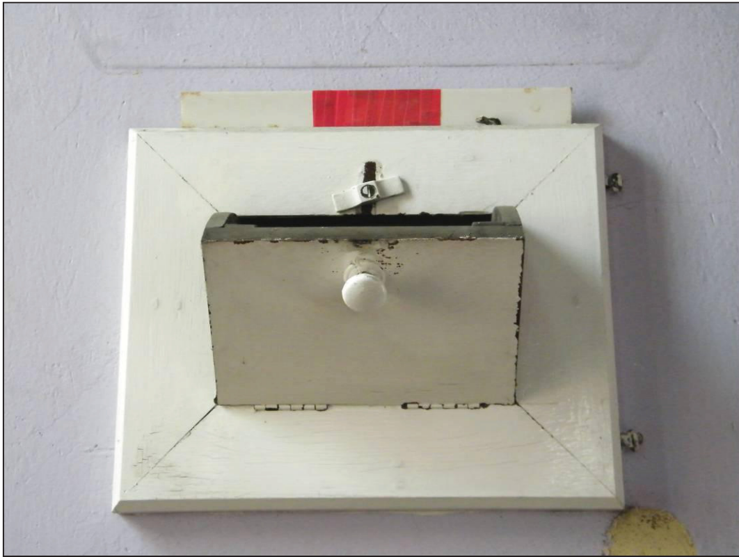
Plate 21 (Shot 45): Detail of one of eight ventilation holes in the chapel. Looking south
